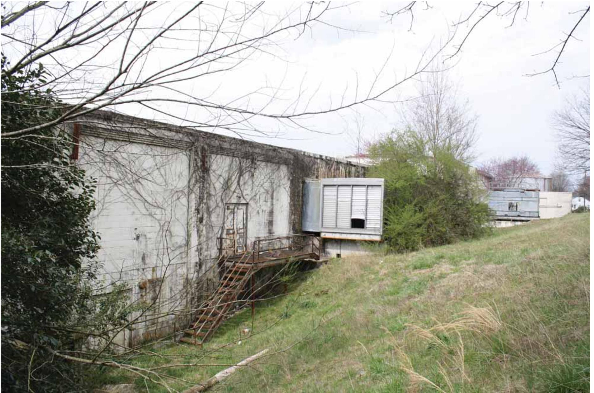
**Photo 5 of 20.** Black Ox – Duplan Corporation Mill, facing northwest from the southeast corner of the property. Showing the one-story 1947 addition (left) to the south end of the circa 1929 addition and the two circa 1980 air handling units.
