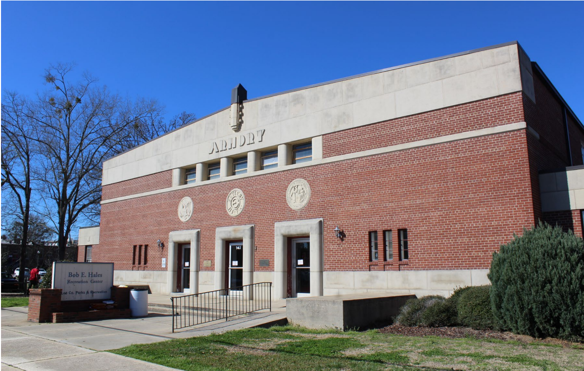
147 McIver Street, Downtown Sanford Historic District Boundary Increase, Facing West
