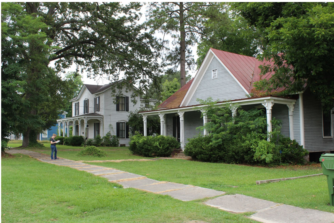
122-200 Southwest Railroad Street, Enfield Historic District, Facing Southwest
