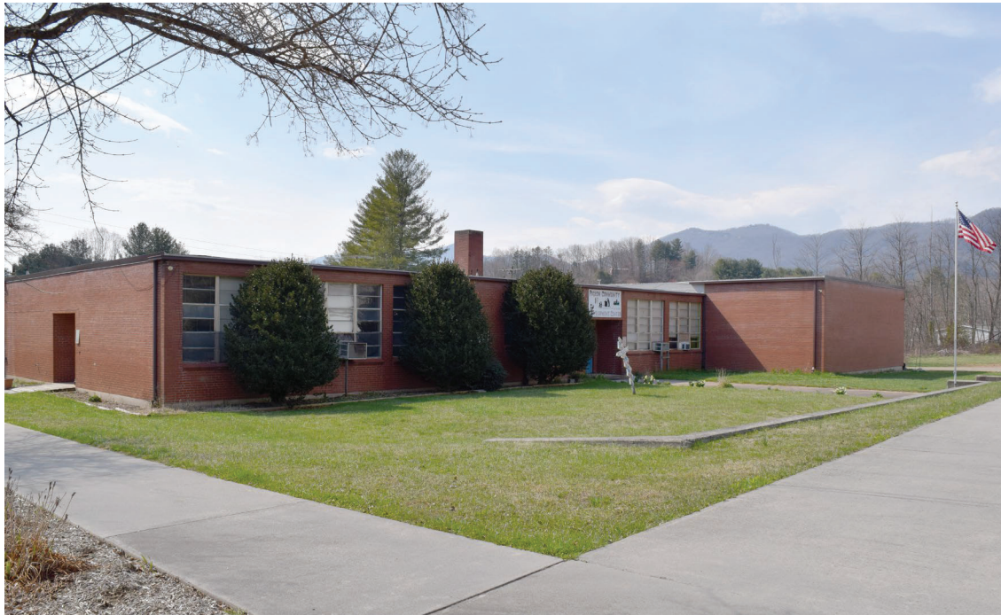
Site and building location, view southwest.
