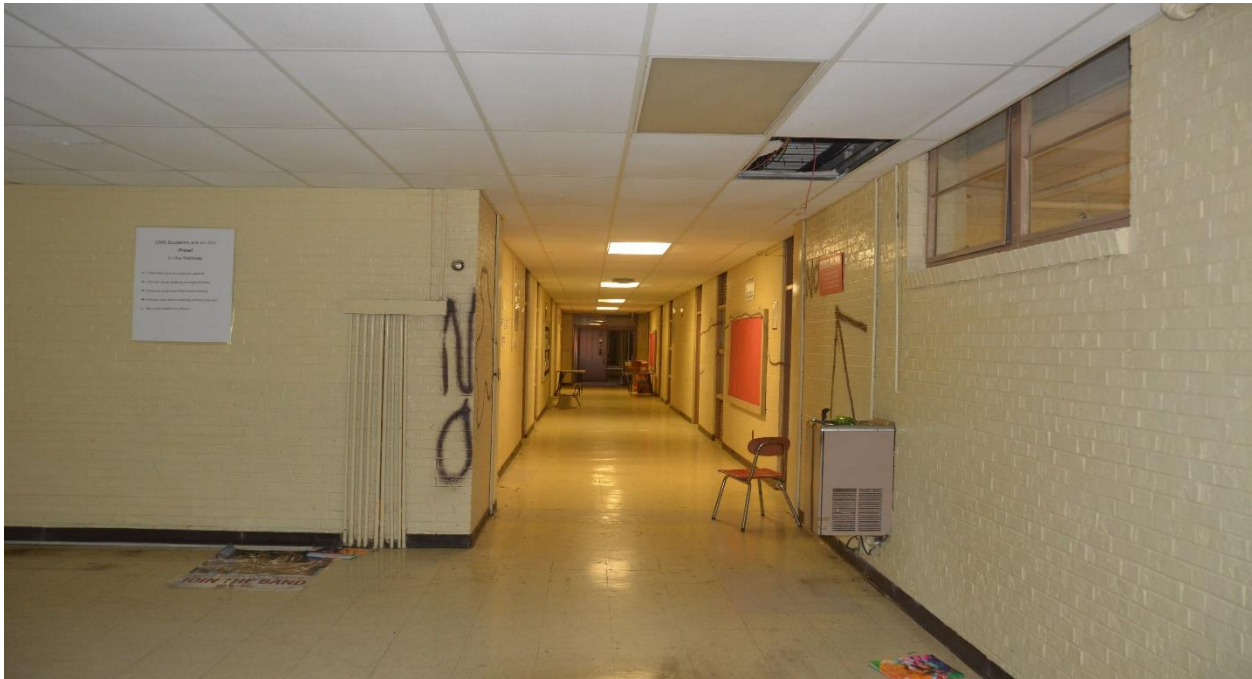
Westside corridor looking to doors to south
