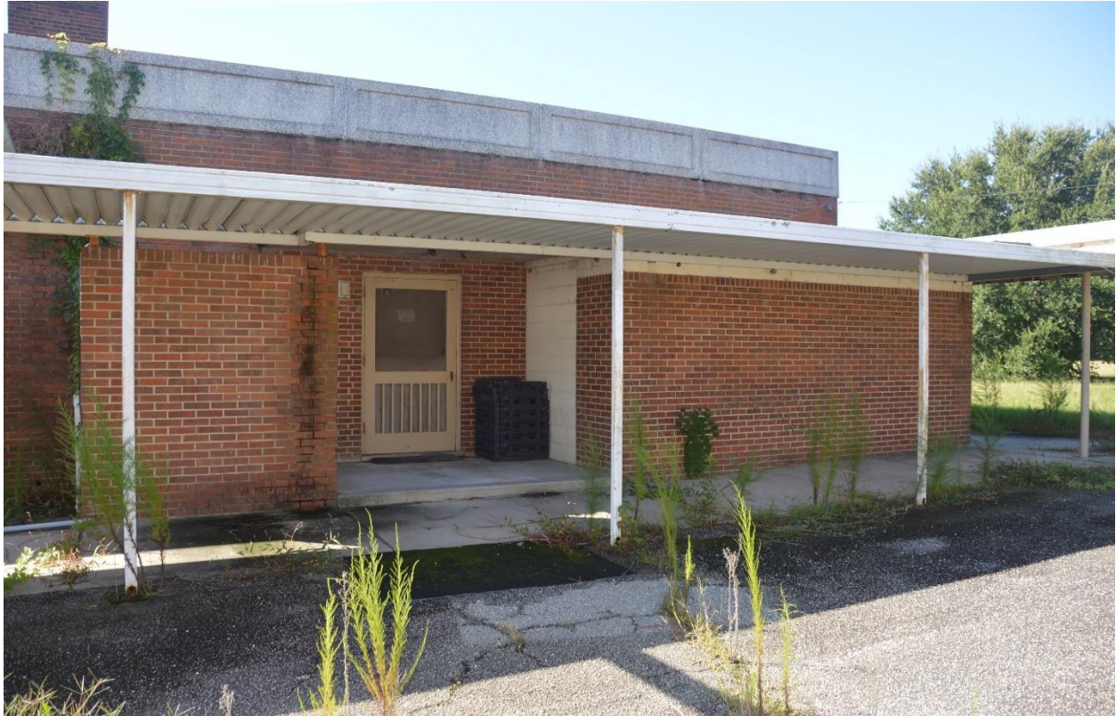
Westside Entrance Kitchen/Boiler Room Access
