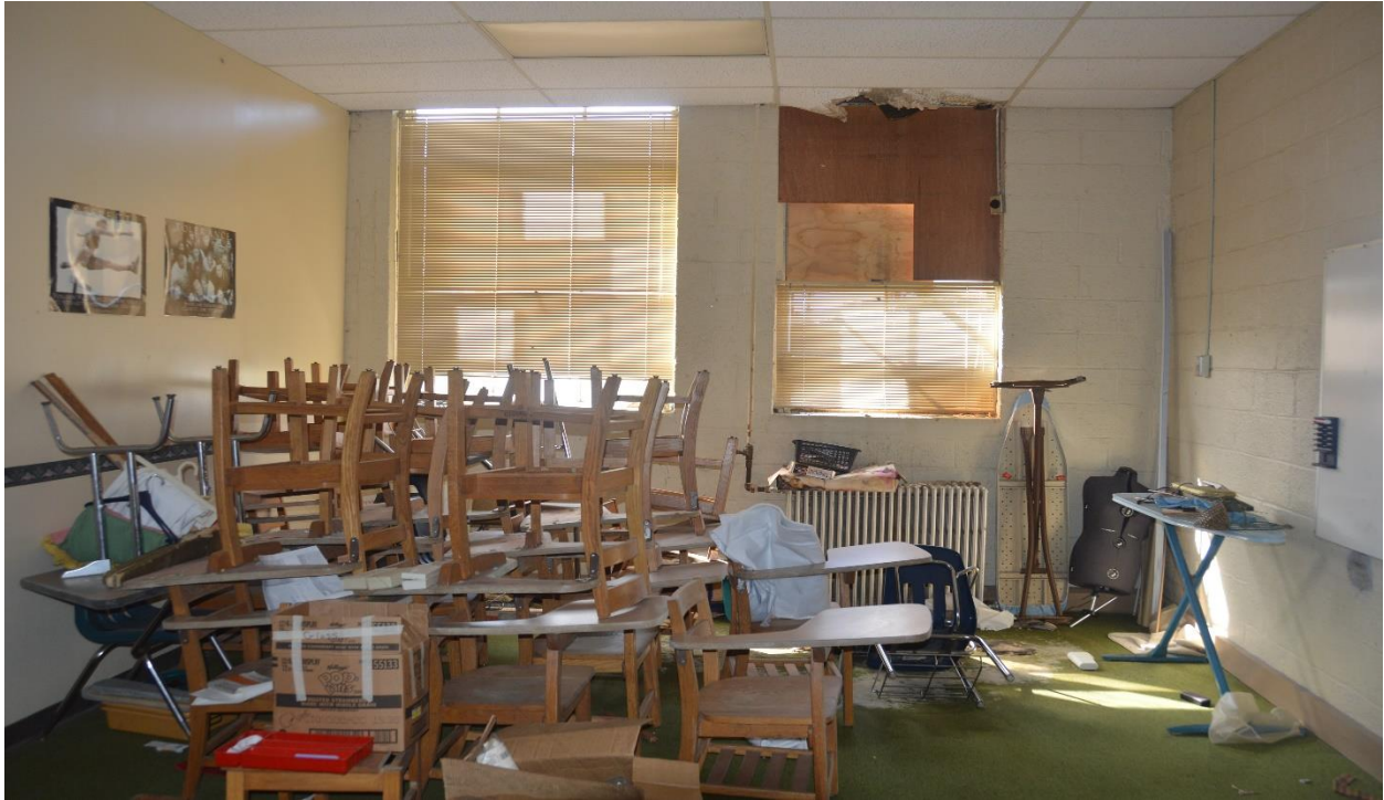
Westside Classroom on east of corridor
