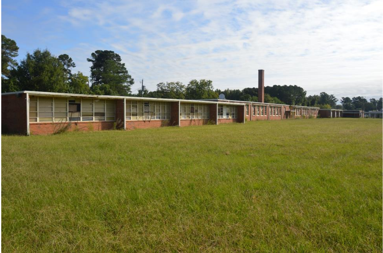
West View of Building Front
