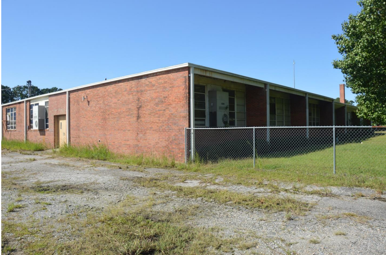
Westside School, façade, Rear elevation
