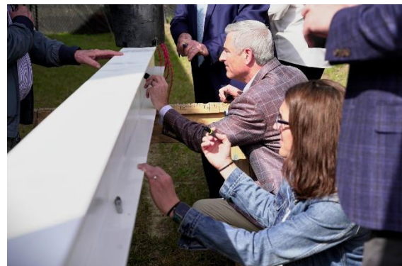
Figure 4: Kirk DeViere, chair of the Cumberland County Board of Commissioners, signs the final steel beam during the topping off ceremony for the North Carolina History Center on the Civil War, Emancipation & Reconstruction
