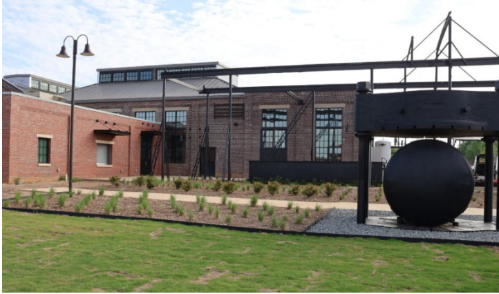
Figure 8: A current project that's underway and scheduled for completion in early 2027. The former Spencer Shops' Powerhouse is being completely renovated and will serve as a venue for rotating exhibits and event space for gatherings.
