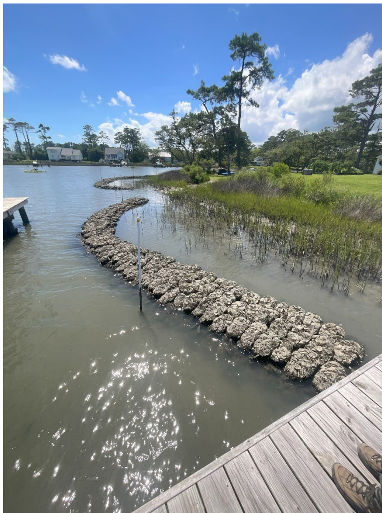
Figure 17: Living shoreline with oyster sill, credit NCCF
