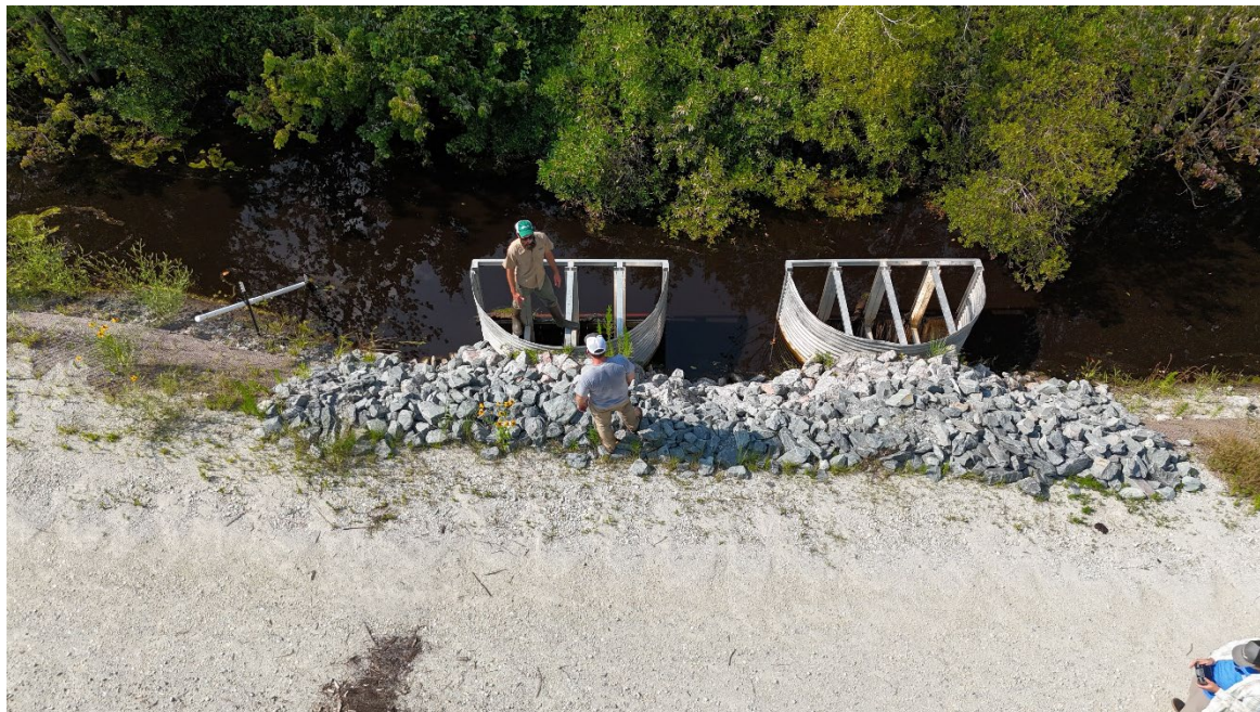
Figure 7: TNC & WRC staff monitor water levels at new water control structures in restored peatlands at Angola Bay Game Land, credit Margaret Fields
