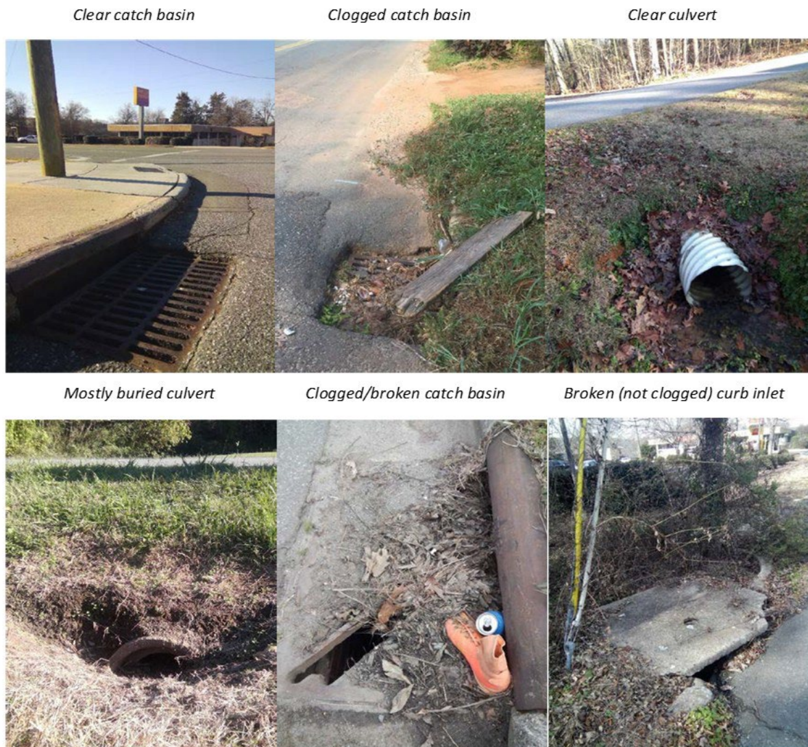
Figure 12: Regular maintenance can prevent water pollution and ponding around clogged stormwater infrastructure, credit Maya Cough-Schulze
