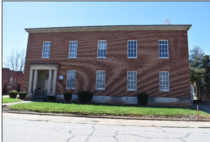
Photograph 44. Bellsouth Telecommunications Building, 35 Academy Street (HW0922)
