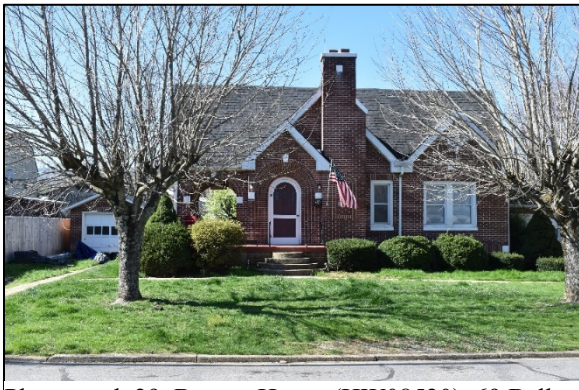
Photograph 29. Bryson House (HW08520), 69 Belle Meade Drive
