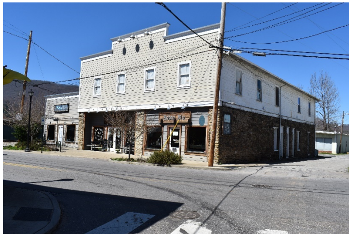
Photograph 43. 486 Hazelwood Avenue (HW0915)
