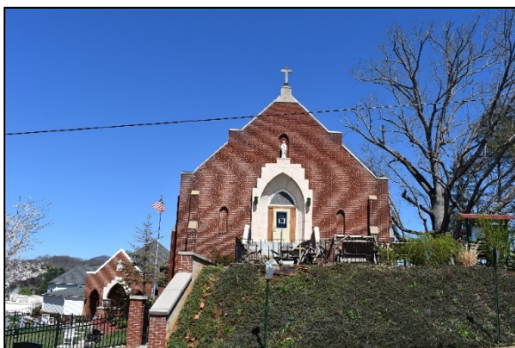
Photograph 47. St. John’s Catholic Church (HW0783), 214 Church Street
