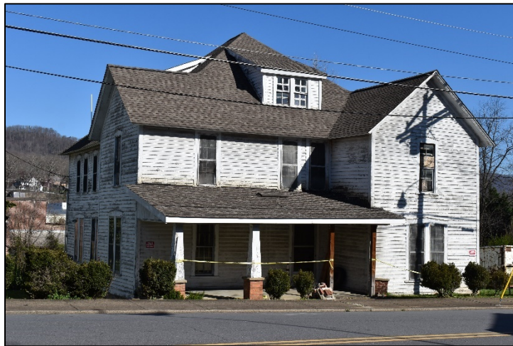
Photograph 54. Miller House (HW0947), 200 Branner Avenue
