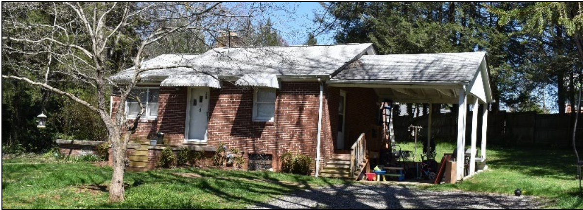
Photograph 38. 306 Balsam Drive (HW0814)
