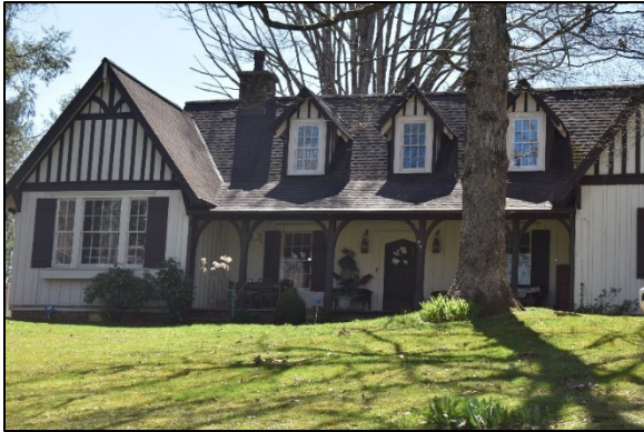
Photograph 27. 95 Balsam Drive (HW0822)
