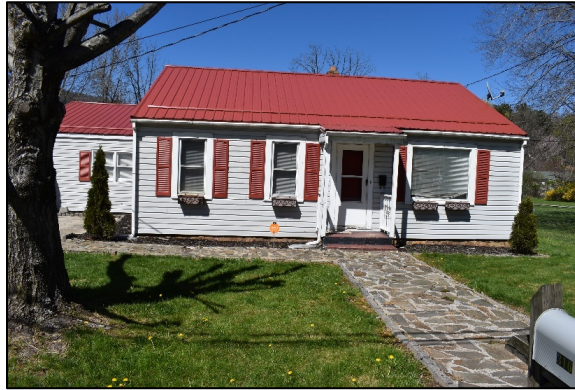
Photograph 32. 316 Hazelwood Avenue (HW00829)
