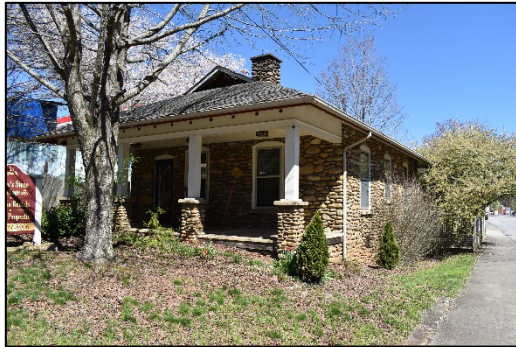
Photograph 4. 33 Pigeon Street (HW0981)
