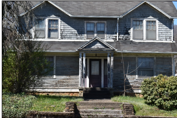
Photograph 16. 506 S. Haywood Street (HW0767)
