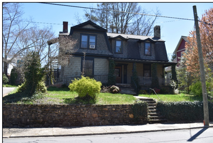
Photograph 18. 635 S. Haywood Street (HW0924)
