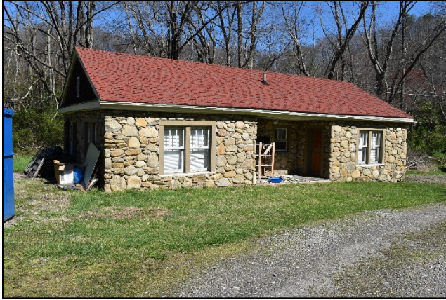
Photograph 55. Skyland Cottages (HW0955)
