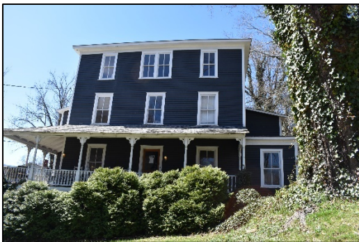
Photograph 2. Palmer House (HW0115)
