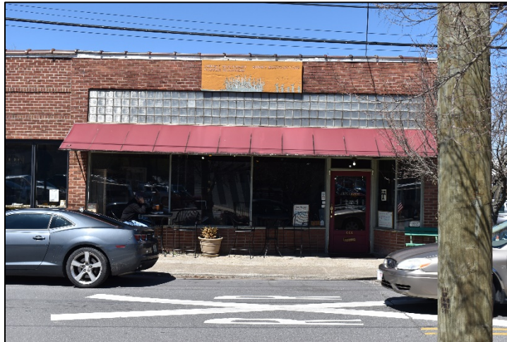
Photograph 42. 444 Hazelwood Avenue (HW0911)
