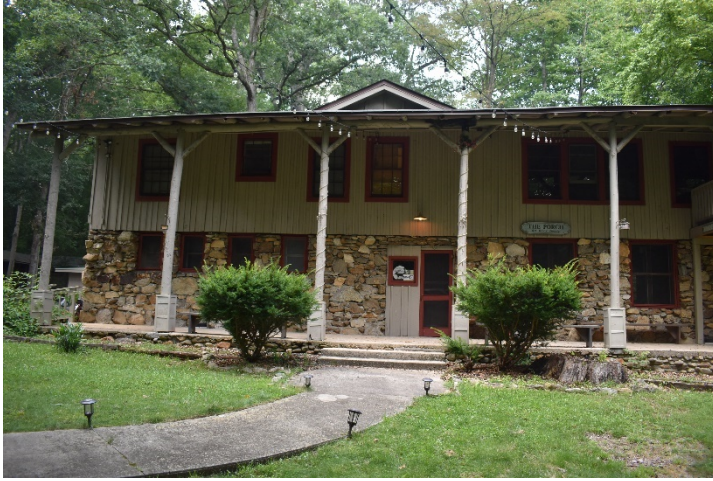
Photograph 59. Furry's Lodge, Main Lodge (Building A)
