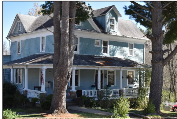
Photograph 12. 101 East Street (HW0867)
