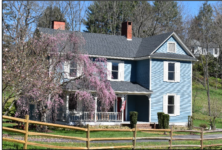
Photograph 7. Howell House (HW0807)
