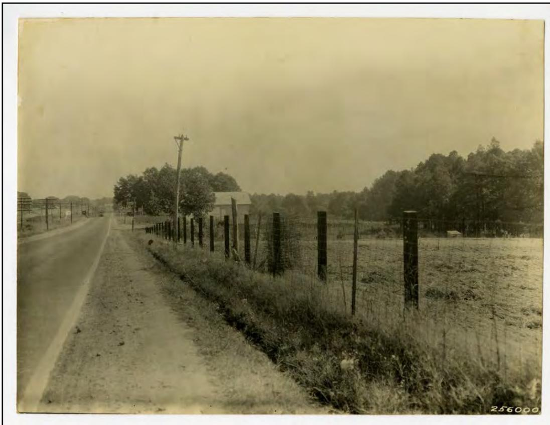
Figure 2.8: Photograph of red oak telephone poles and wire fence in Cary (Graeber 1930).
