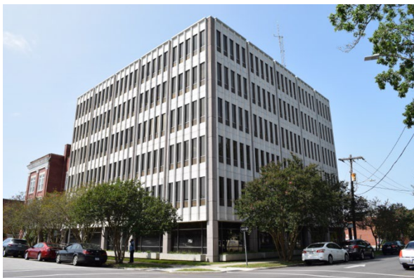
The second Carolina Telephone and Telegraph Building (ED1516) on E. James Street.
