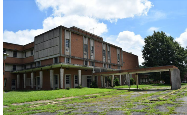
Edgecombe Memorial Hospital (ED2016) on North Main Street dates to 1959
