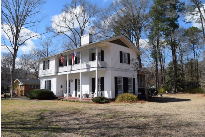
Bridgers House (ED2001) at 1400 W. Canal Street, Tarboro
