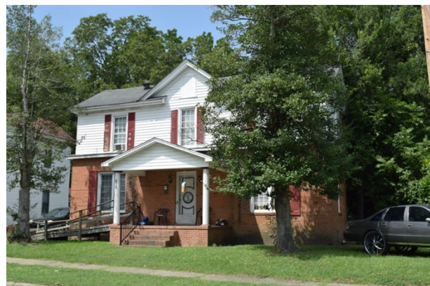
Pattillo House (ED1519) on East St. James Street
