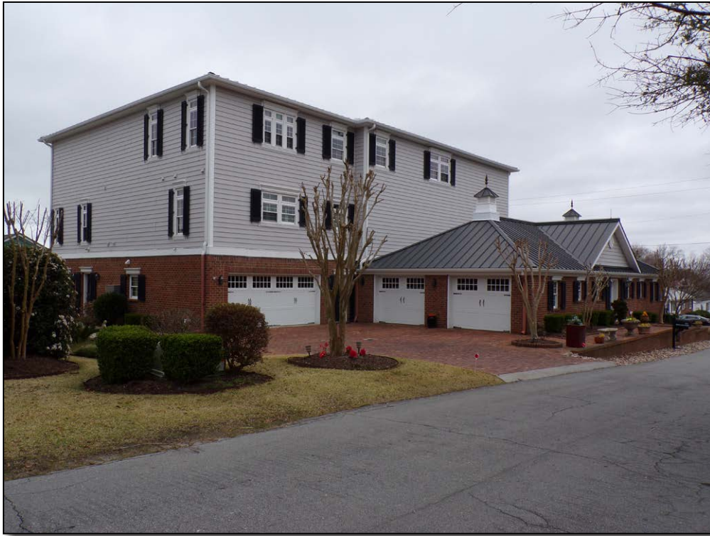
Figure 5a: View south of the house at 223 Walnut Street (ON0879).
