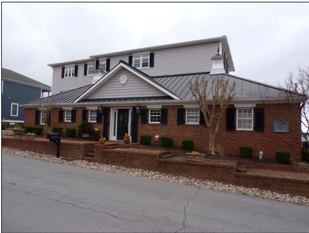
Figure 5b: View southeast of the house at 223 Walnut Street (ON0879).
