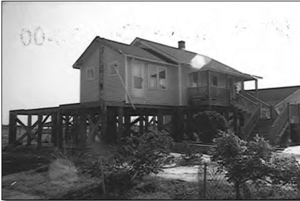
Figure 7a: View south of the Bessie Darmo House at 215 Water Street (ON1007) in 2000, after elevation but prior to enlargement of the wing (NC HPO).
