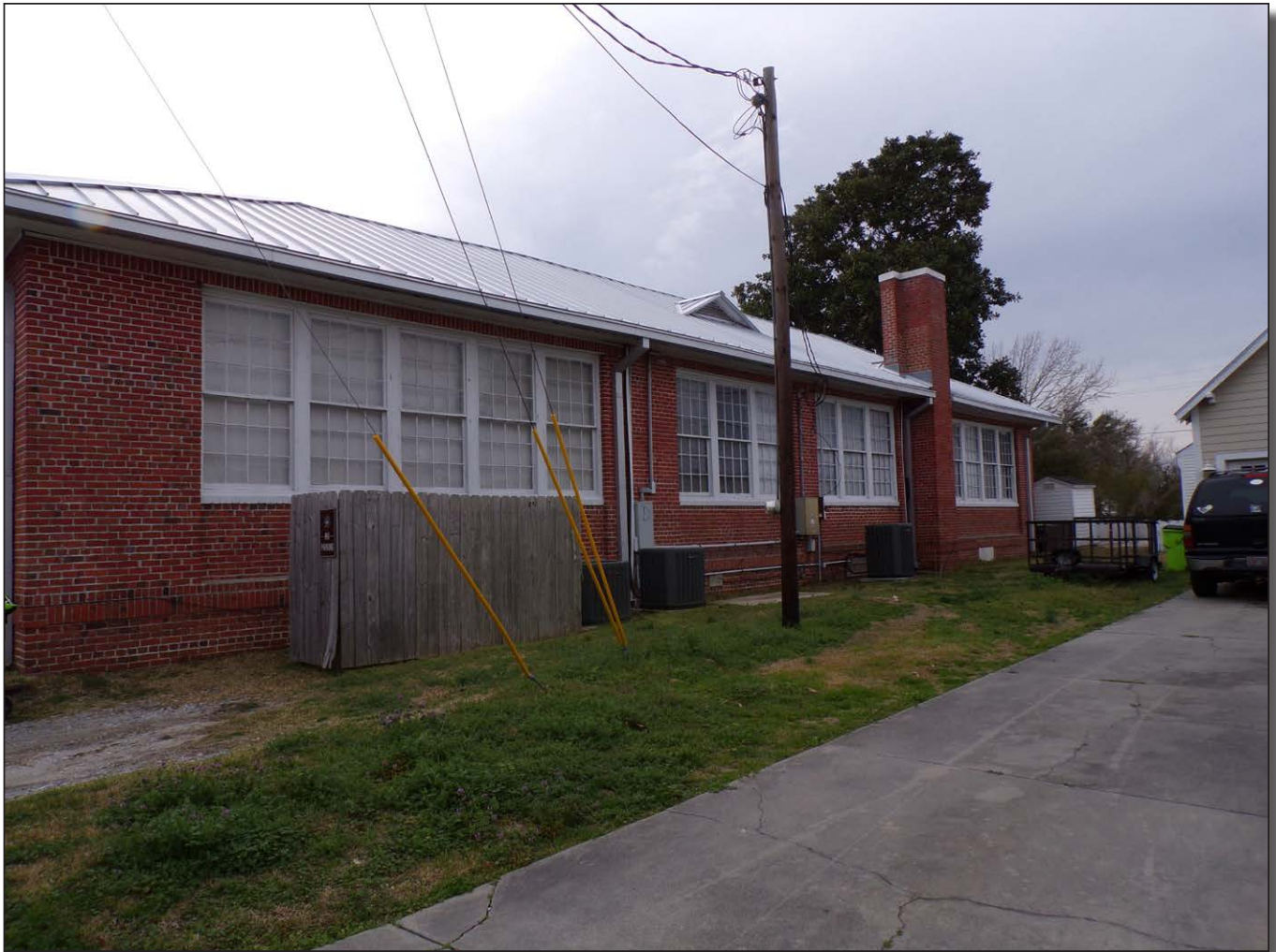
Figure 12: View north of the Emmerton School at 502 Church Street (ON0833).
