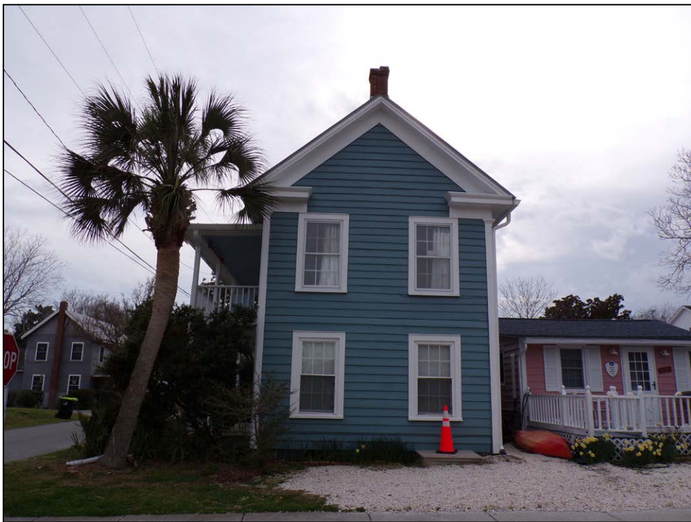
Figure 9b: View southwest of the Robert Lee Smith House at 202 Walnut Street (ON0914).
