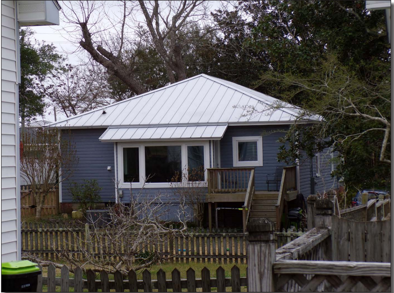
Figure 11: View southeast of the Mart Bloodgood House at 116 Water Street (ON0823).
