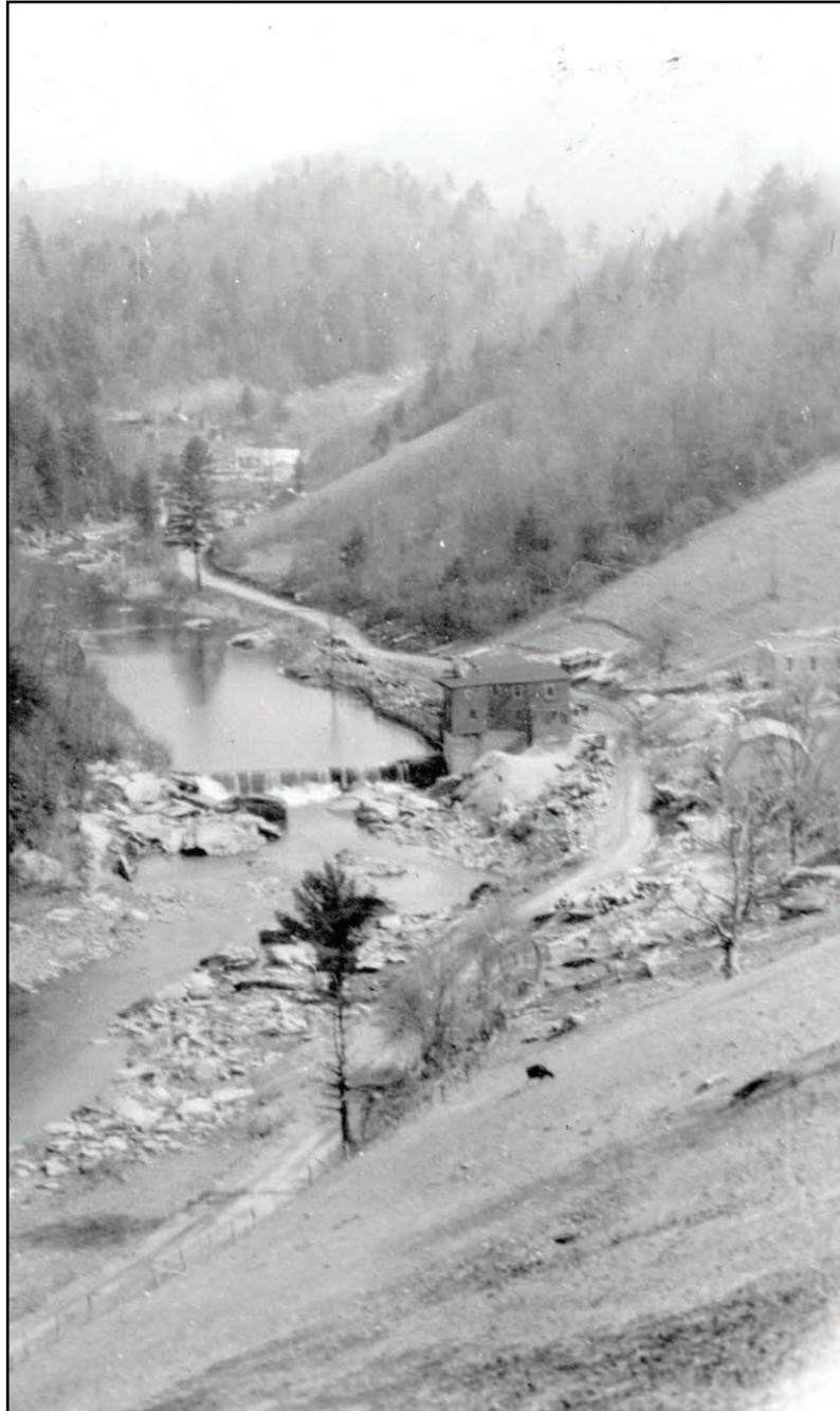
Figure 2.7: Lorenzo Ward's circa 1905 hemlock dam across Watauga River. This dam was dismantled in 1963 and replaced with a concrete dam (Courtesy of The Foxfire Museum).
