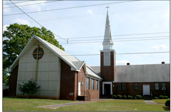
Figure 37: Westminster Presbyterian Church, 1126 West Webb Avenue (AM2708)
