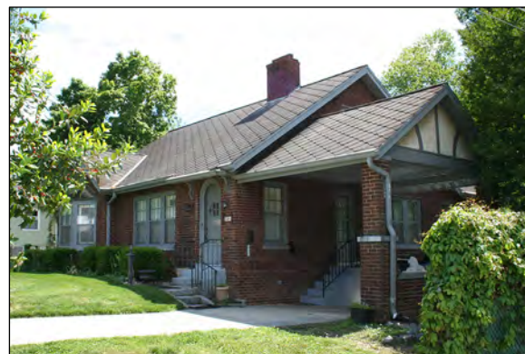
Figure 27: Louis Allen Sr. House, 336 Hillcrest Avenue (AM0664)
