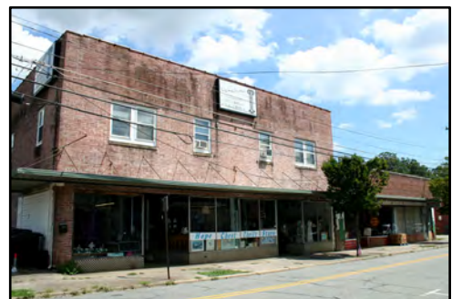
Figure 79: Commercial Buildings (AM1099), 300-block Trollinger Street.
