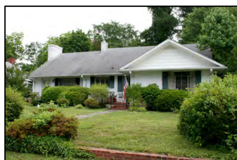
Figures 57-58: West Davis Street-Fountain Place NRHD Boundary Increase Area A. Top to bottom: 819 Central Avenue; 815 Central Avenue.
