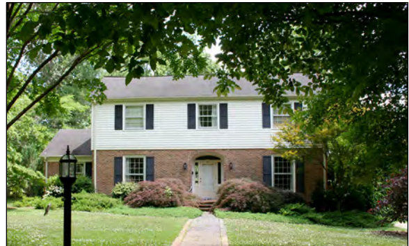
Figure 32: House, 1218 Edgewood Avenue (AM2741)
