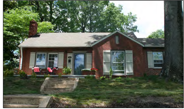
Figure 28: E. Graham Cheek House, 416 Fountain Place (AM0726)
