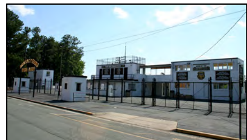
Figures 49-52: Walter M. Williams High School (AM2714). Top to bottom: Exterior facing east, gymnasium, lobby, Burlington City Schools Memorial Stadium
