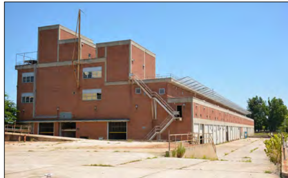
Figure 7: Western Electric Company-Tarheel Army Missile Plant (AM2021) Image courtesy of Heather Fearnbach, July 2015
