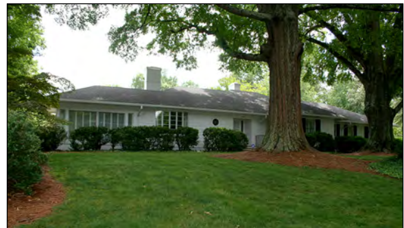
Figure 30: House, 1204 Edgewood Avenue (AM2739)
