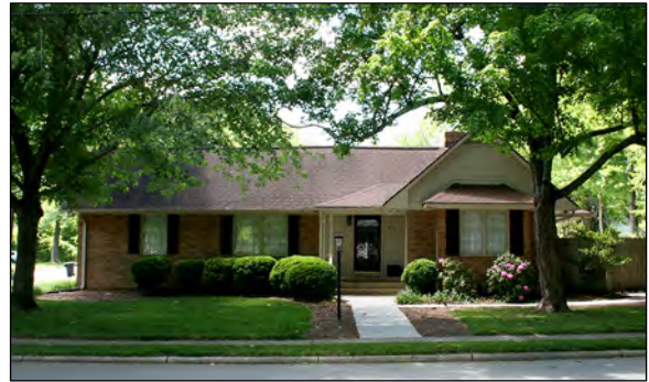
Figure 31: House, 704 West Front Street (AM2691)
