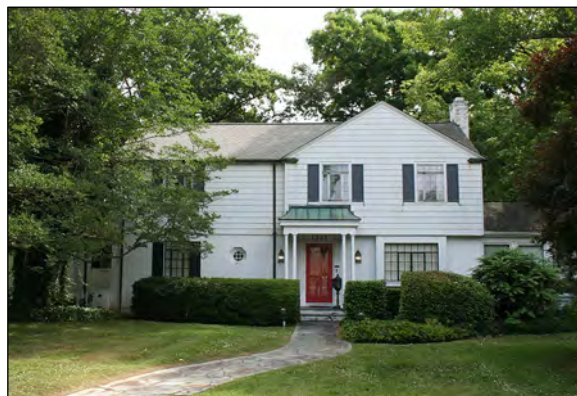
Figure 26: Walter M. Williams House, 1303 West Davis Street (AM1293)
