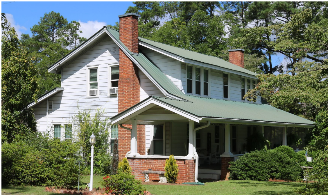
Figure 20. 250 Ashemont Road, Façade and South Elevation
