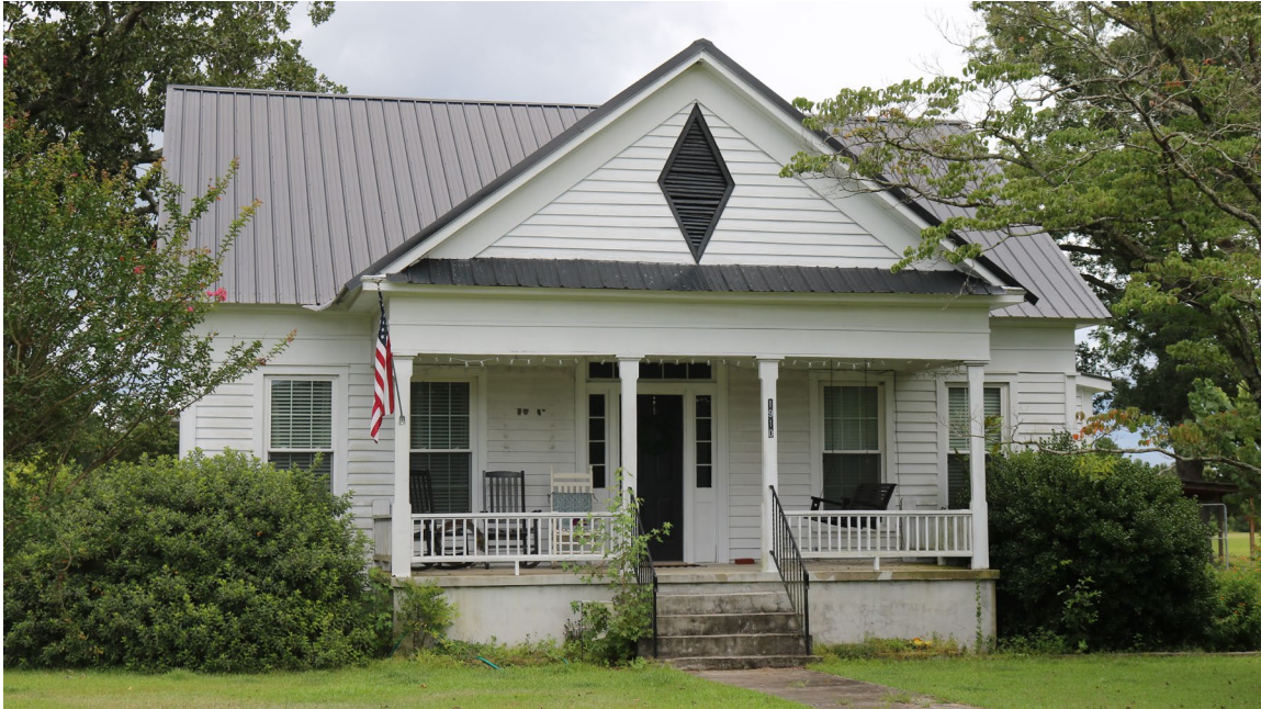
Figure 8. 1910 North Old Wire Road, Façade
