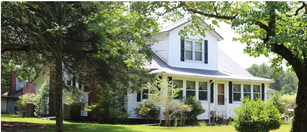
Figure 18. 1047 Quewhiffle Road, Façade and North Elevation
