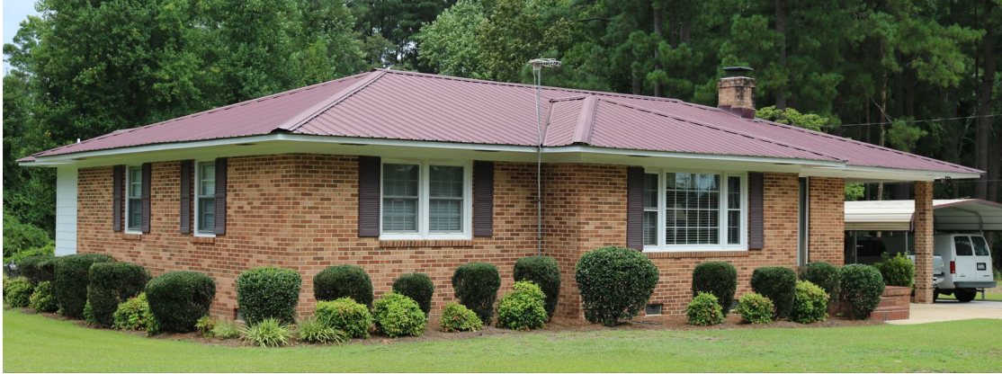
Figure 25. 325 Mockingbird Hill Road, Façade and South Elevation
