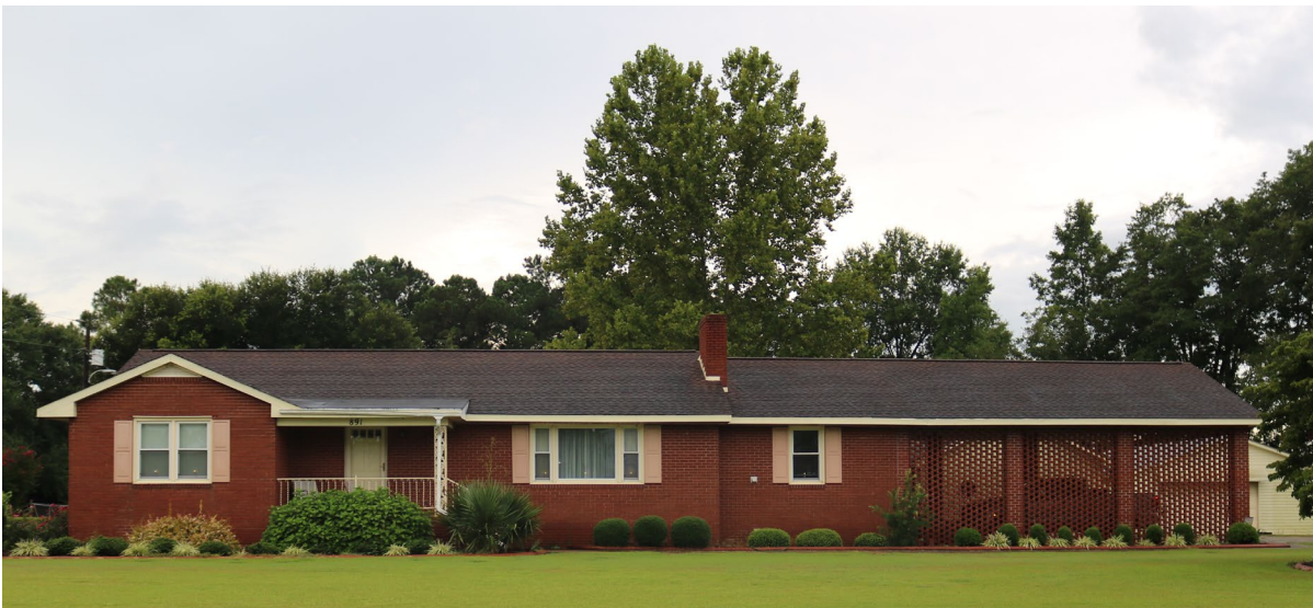
Figure 26. 891 Neill Maxwell Road, Façade
