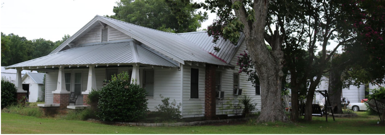
Figure 22. 1176 Will Monroe Road, Façade and East Elevation
