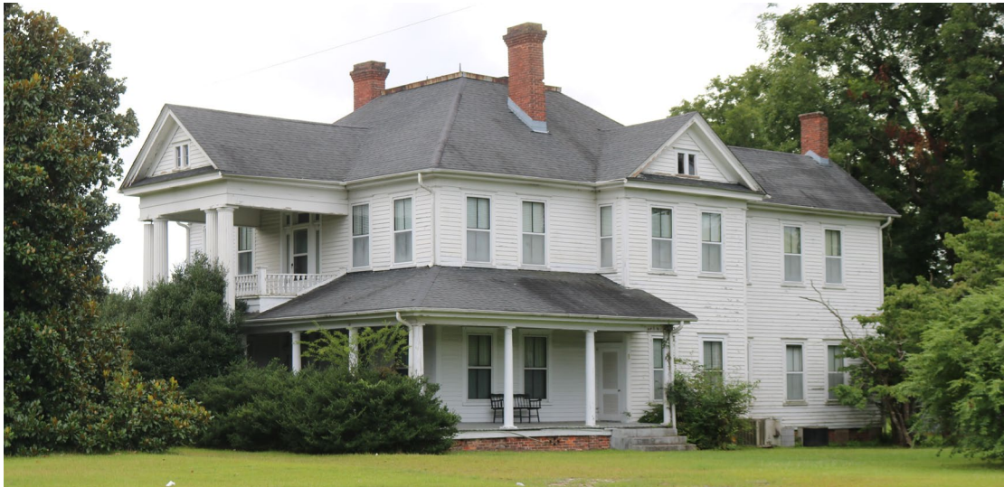
Figure 17. McDonald House, 6588 Red Springs Road, Façade and North Elevation
