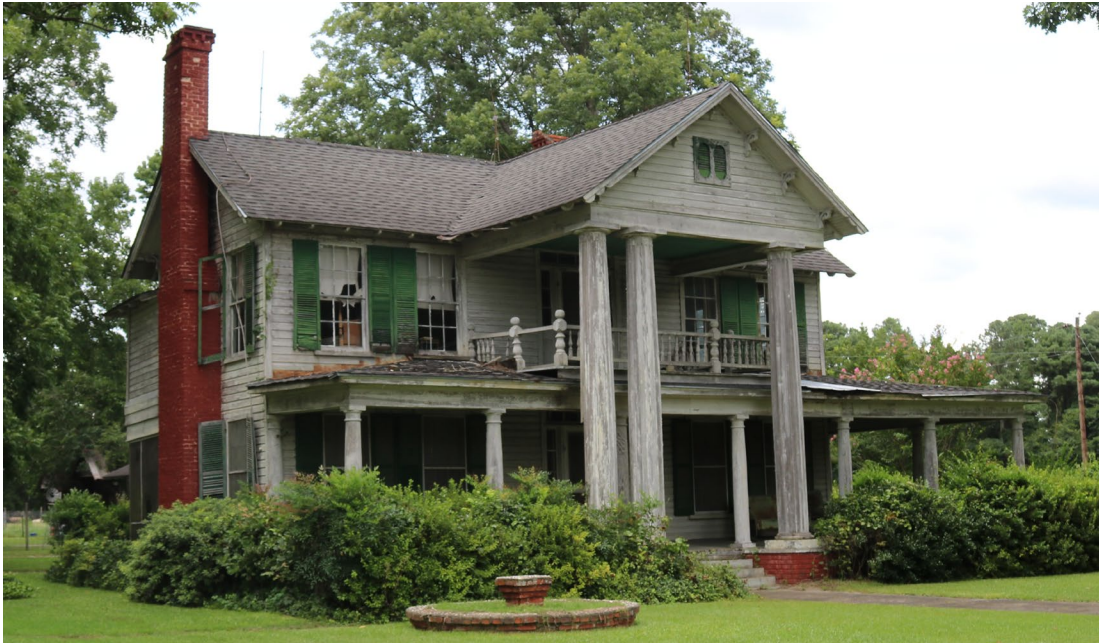
Figure 16. McPhaul House, 2405 North Old Wire Road, Façade and South Elevation
