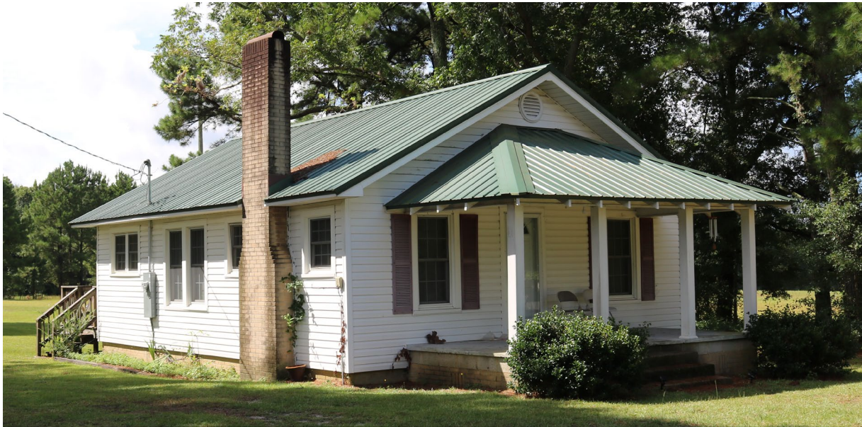
Figure 21. 125 Reservation Road, Façade and East Elevation
