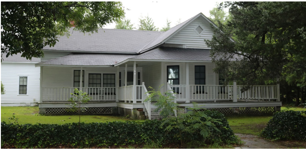
Figure 14. 404 Neill Maxwell Road, Façade
