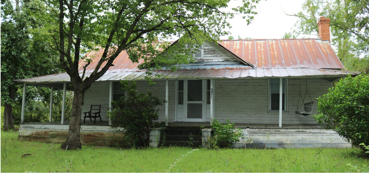
Figure 15. 3211 North Shannon Road, Façade
