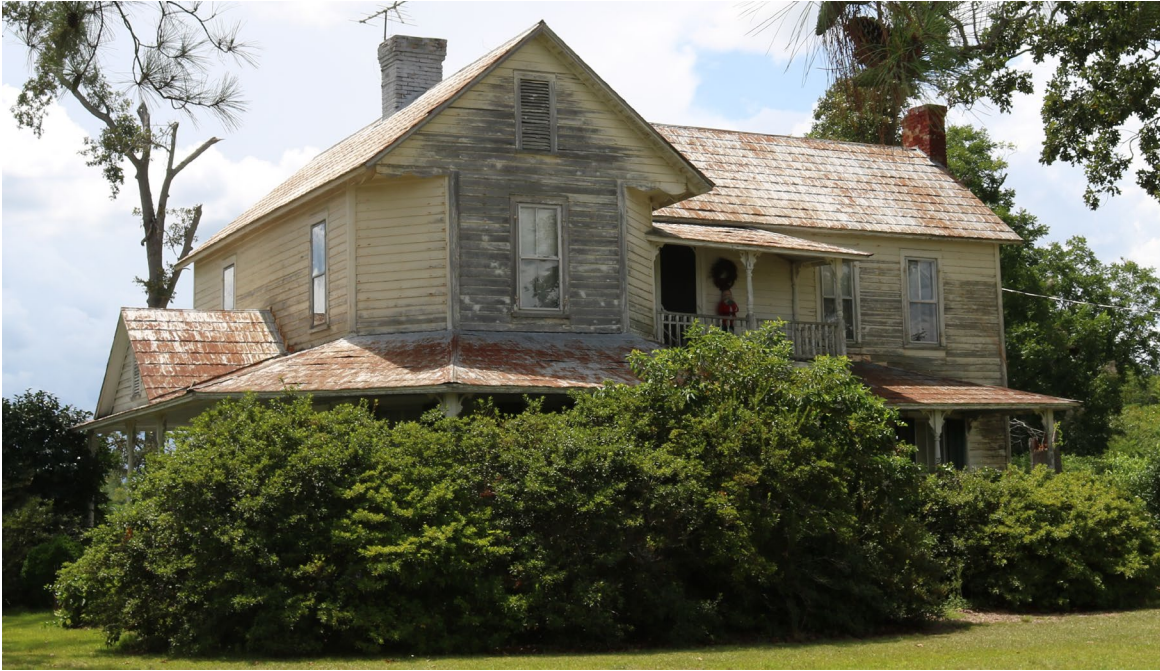
Figure 10. 1574 Saint Pauls Drive, Façade
