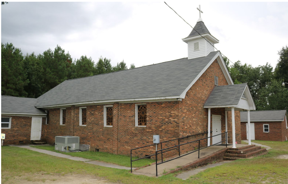
Figure 38. McCormick Chapel, Shannon Vicinity
