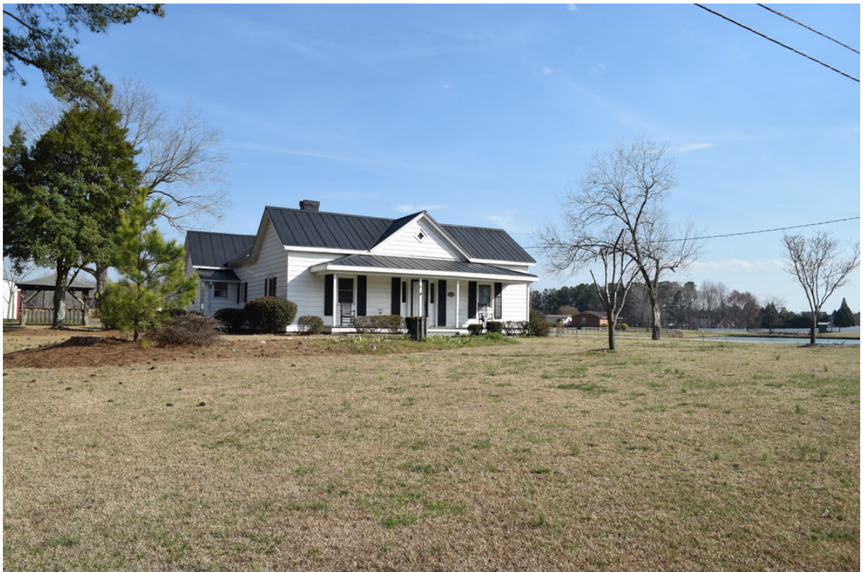
Stephenson-Sauls House, view from Old Stage Road to the east-southeast
