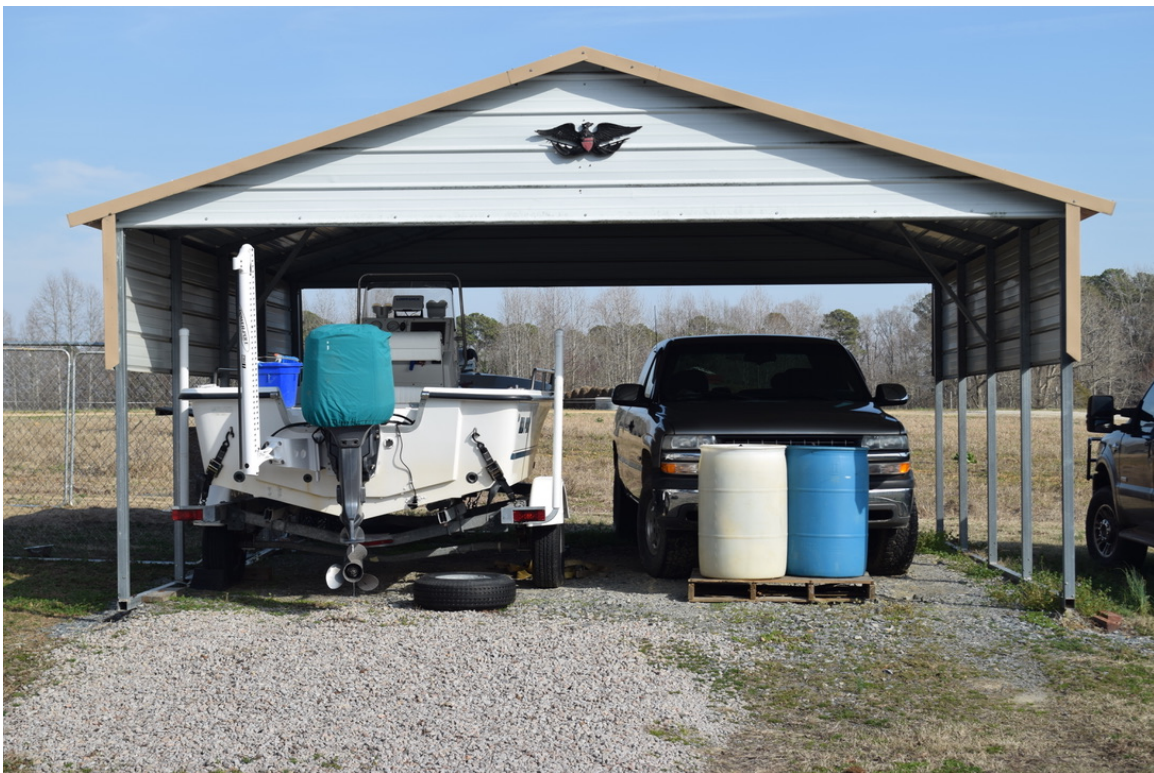
Carport, view to the east
