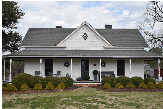
John H. and Nevada Seagroves house facade, view to the north
