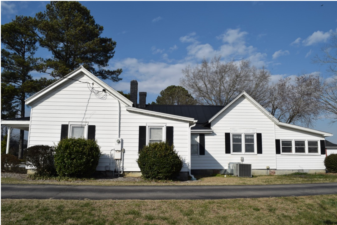
South elevation, view to the north
