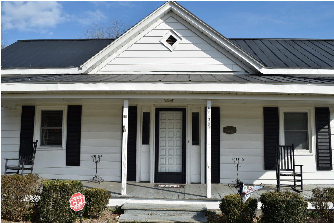
Front of the house, view to the east
