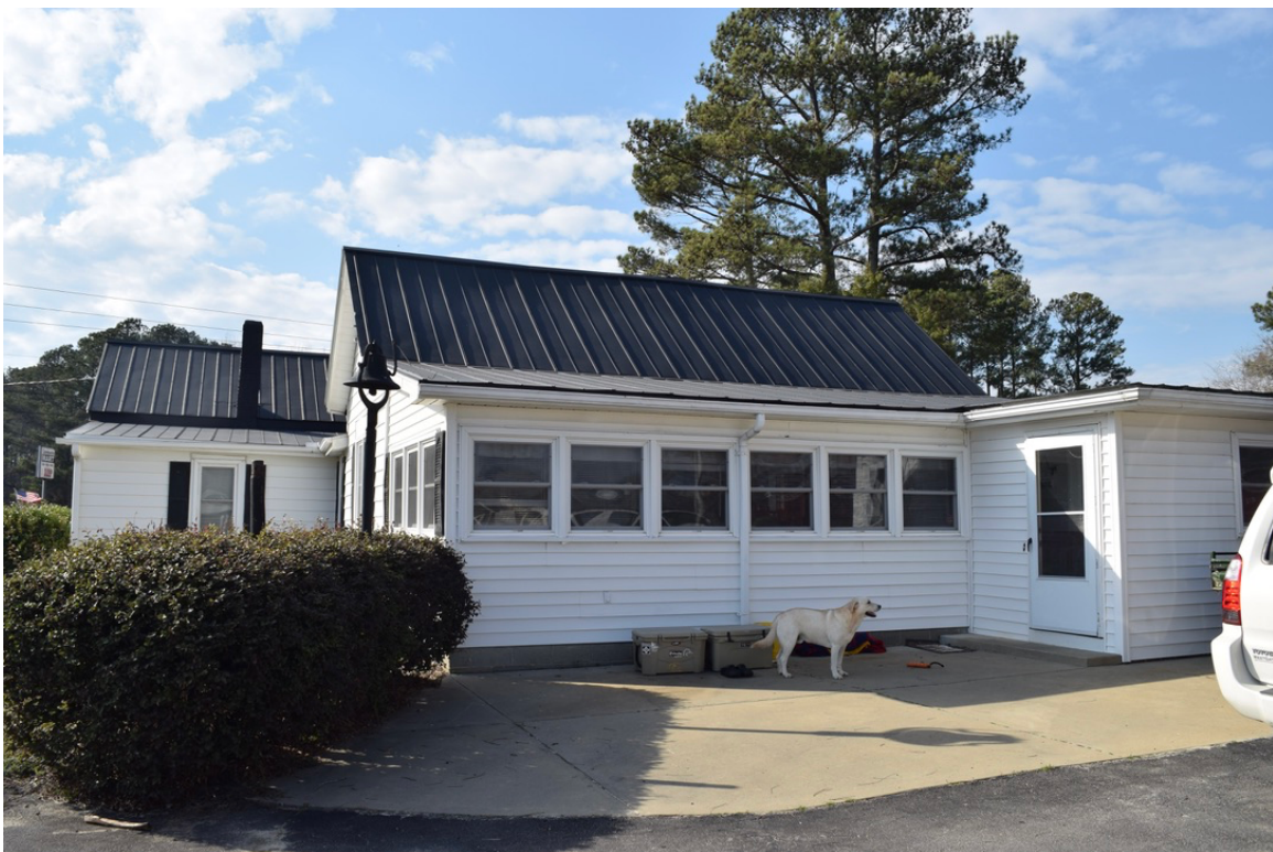
Rear elevation, view to the west
