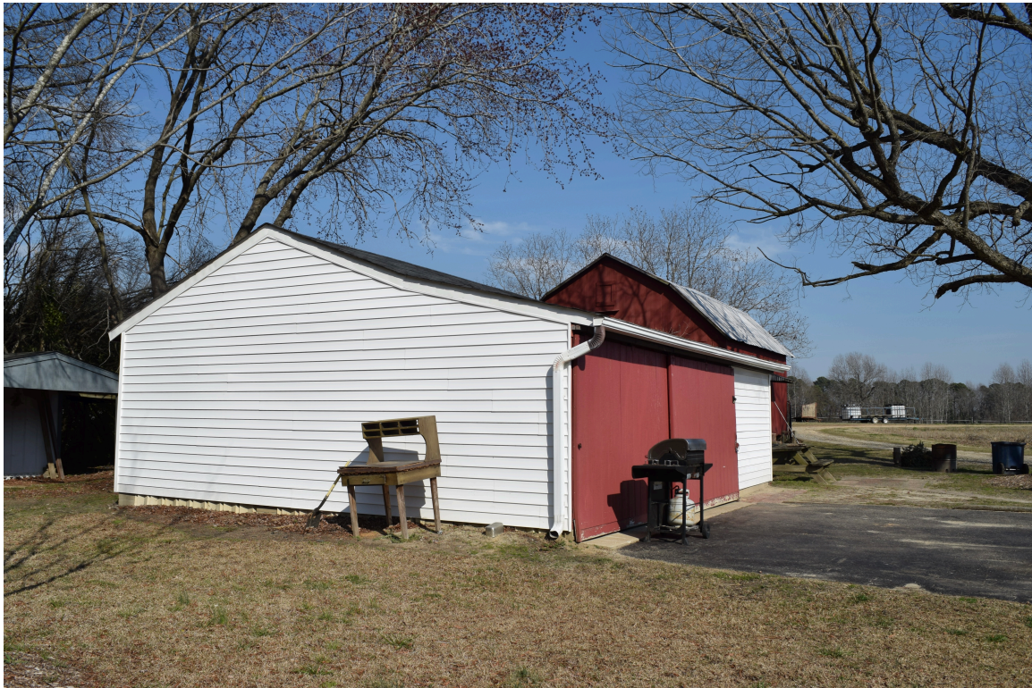
Garage, view to the east-northeast
