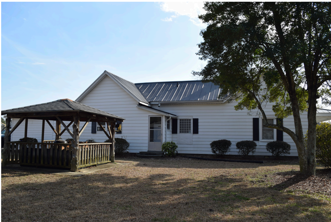
North (side) elevation, view to the south
