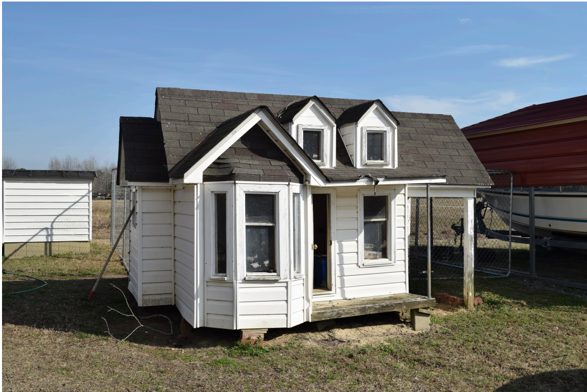
Playhouse view to the east-southeast
