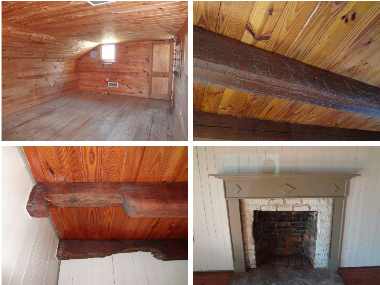
Figure 22. Representative photographs of interior alterations to the original log structure. Top left: loft space with replacement tongue and groove finishes; top right: hand hewn adze marks on ceiling joists; bottom right: replacement mantel; and bottom left: exposed notching on ceiling joists.
