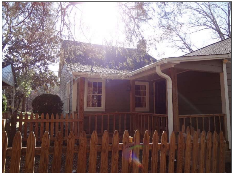
Figure 20. View of the northeast corner of the structure showing the original single-pen, the shed roof addition and the addition attached to the north façade.
