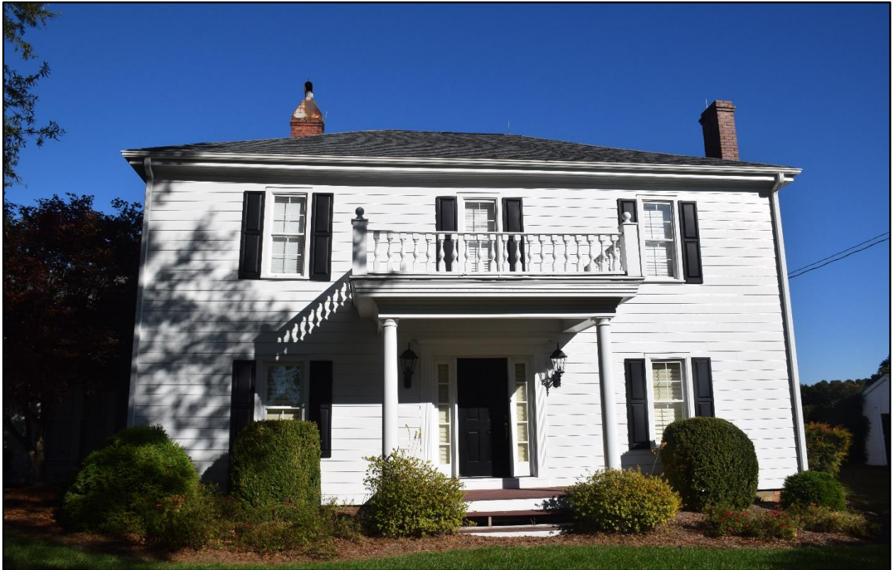
Figure 5- Main House- Facing north toward façade.
