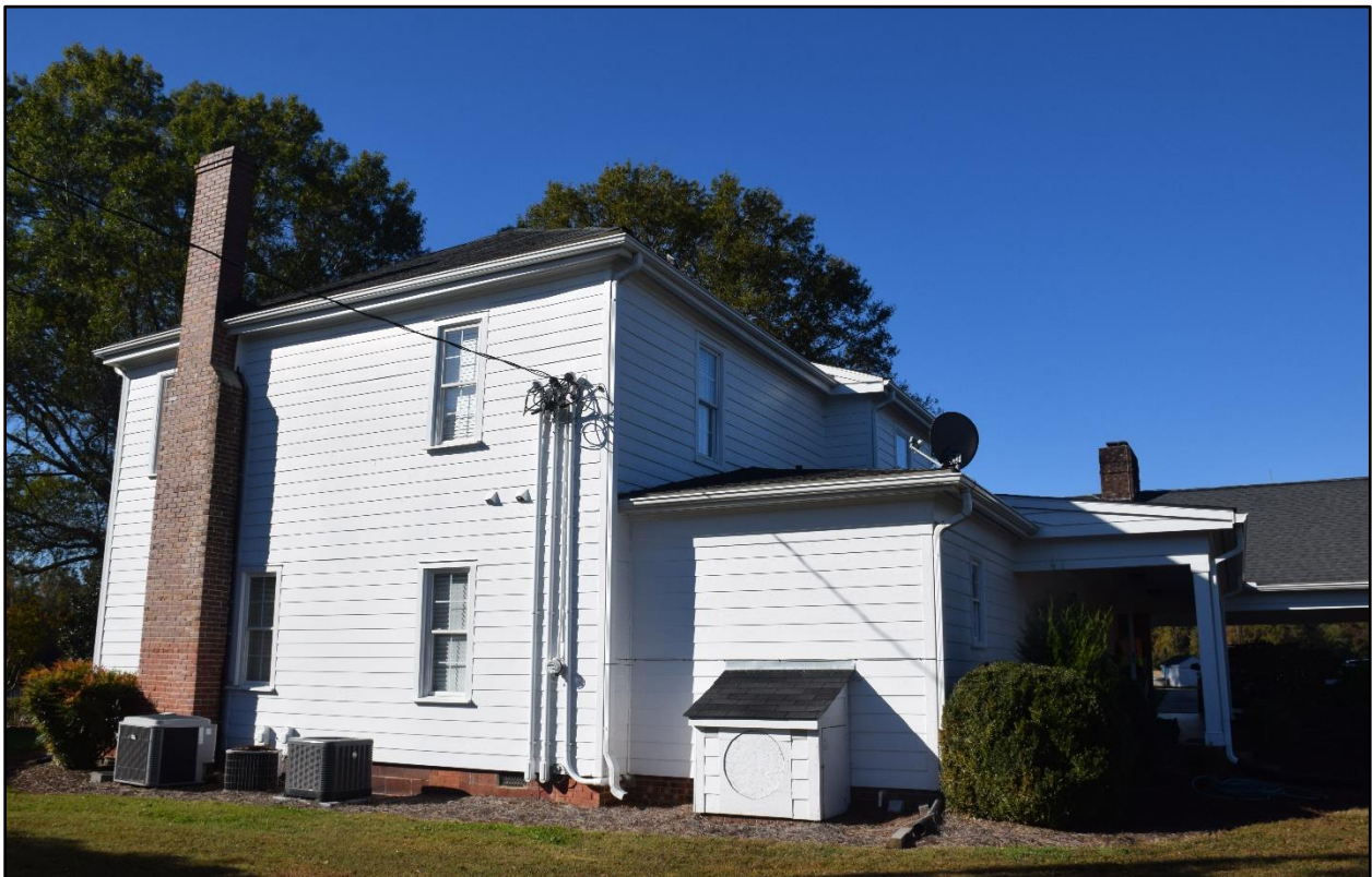
Figure 13- Main House- Facing west toward east elevation.
