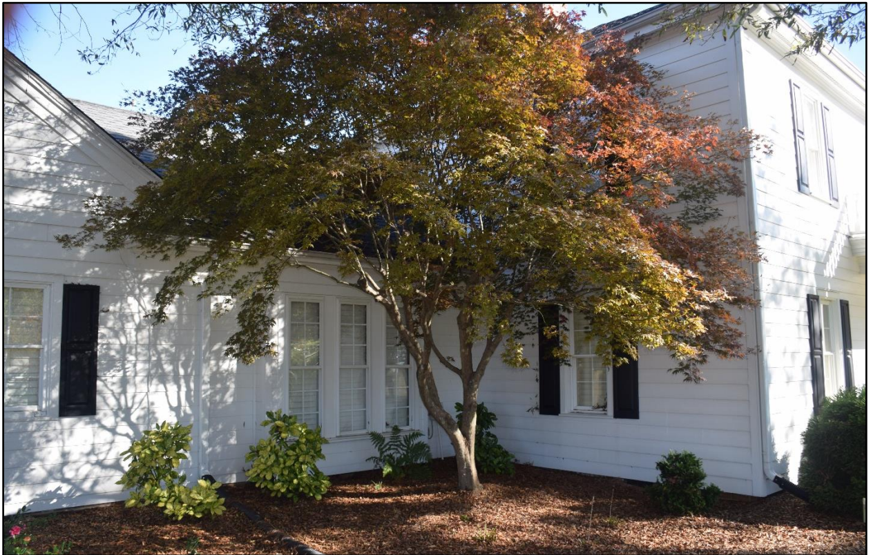
Figure 7- Main House- Facing northeast toward façade and west elevation.
