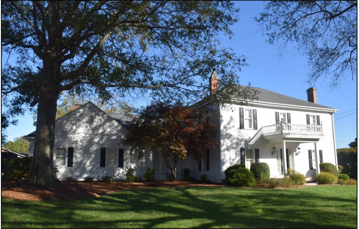
Figure 4- Main House- Facing north toward façade.
