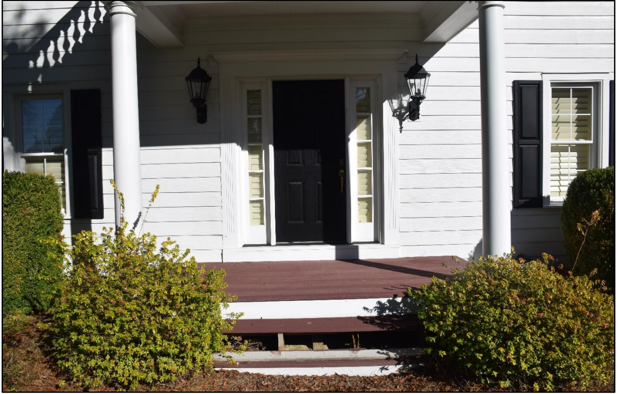
Figure 6- Main House- Front entrance door detail.
