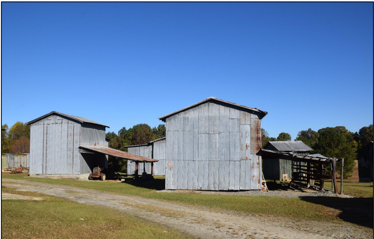
Figure 21- Facing north toward former ca. 1930 tobacco barns.
