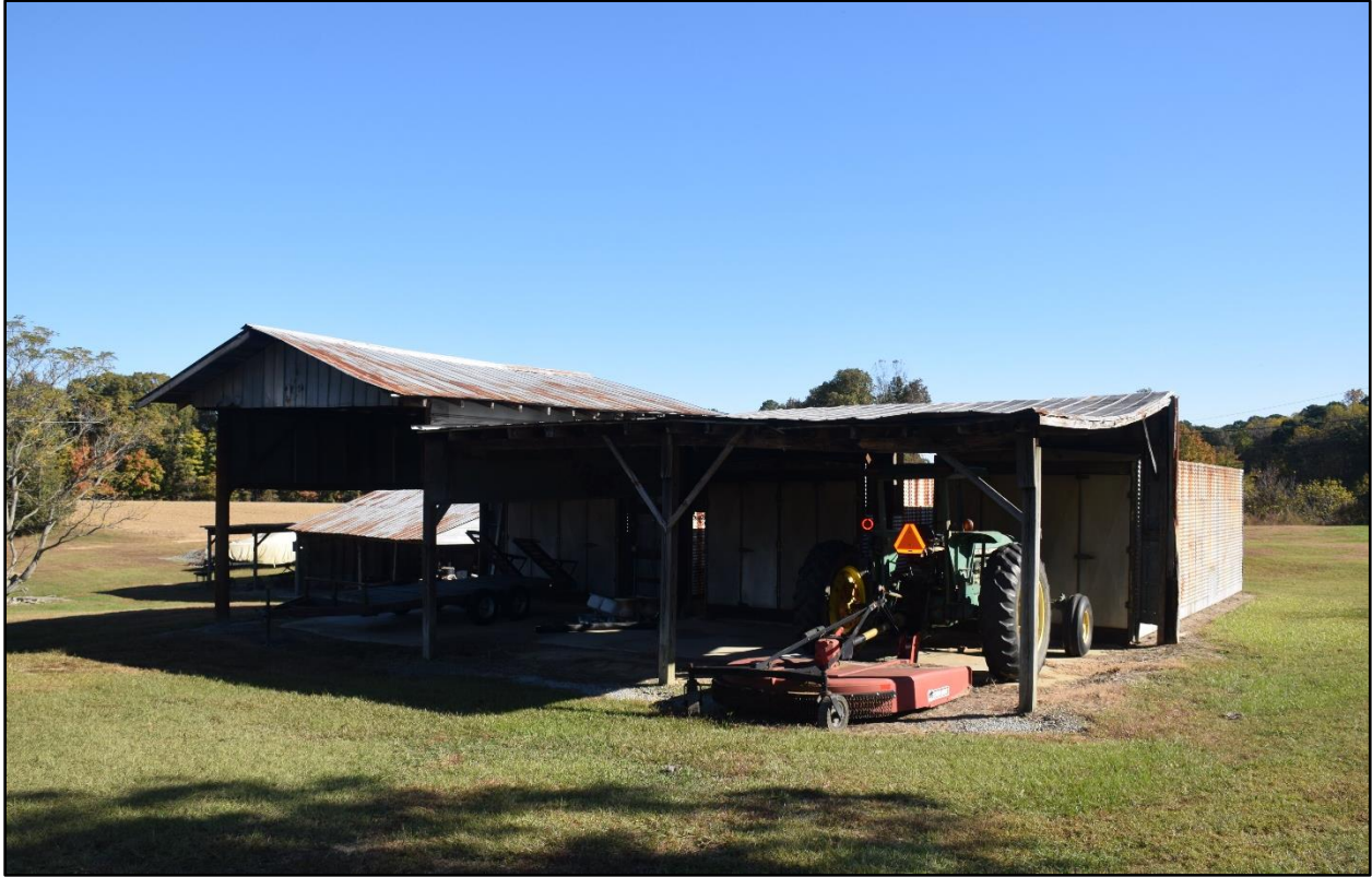
Figure 24- Facing east toward ca. 1980 storage shed.
