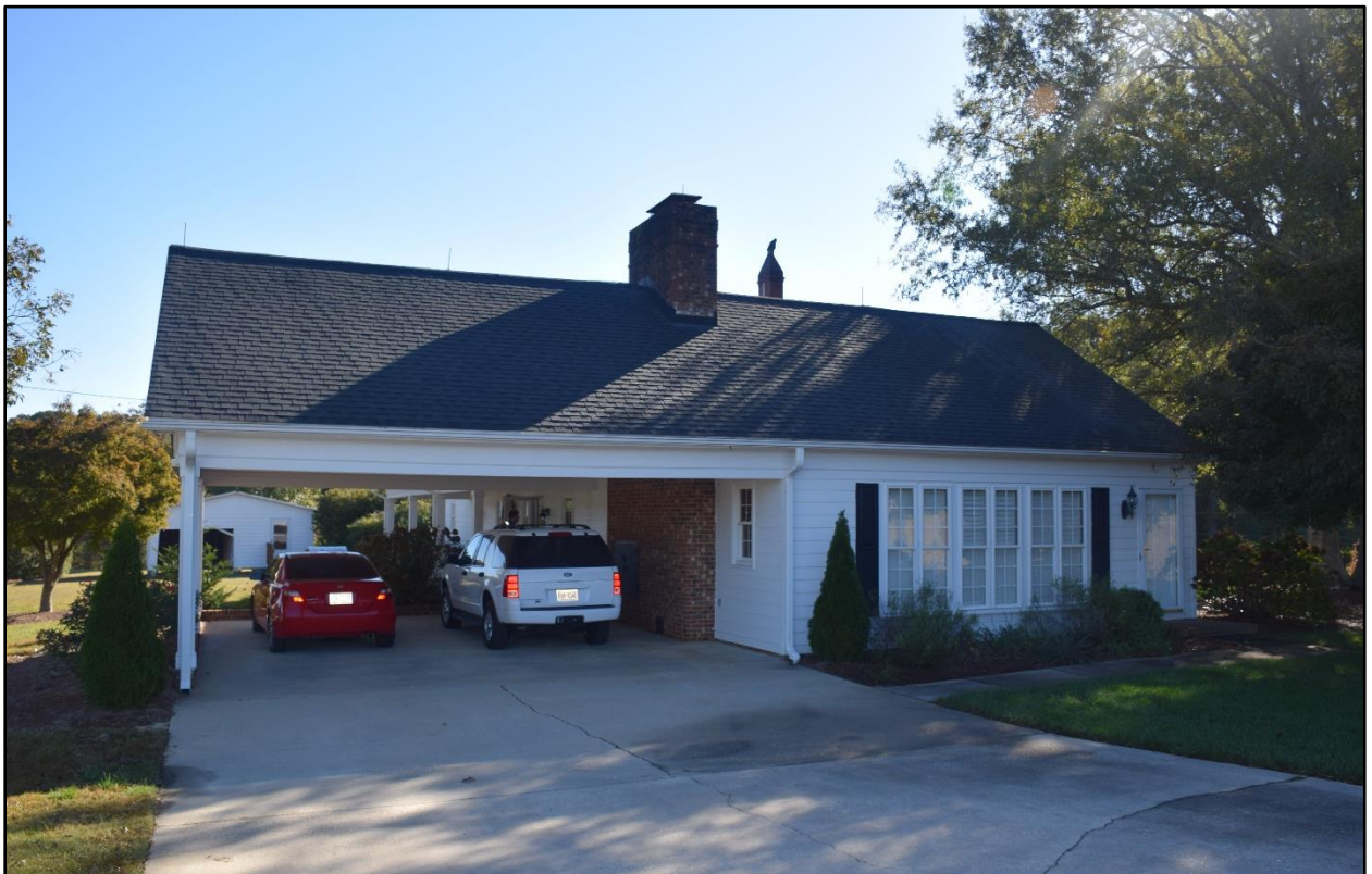
Figure 9- Main House- Facing east toward west elevation and carport addition.
