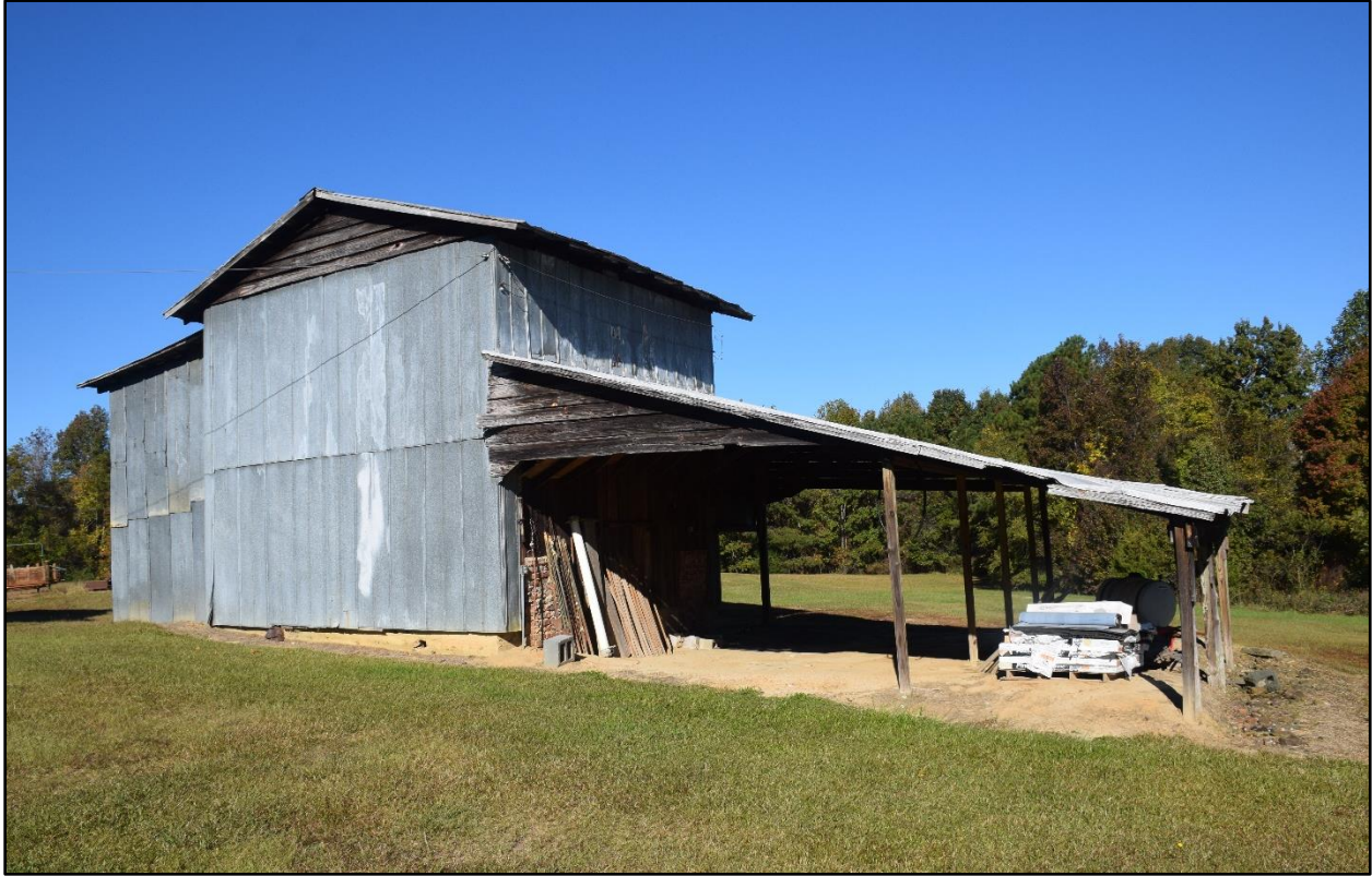
Figure 20- Facing north toward former ca. 1930 tobacco barn.
