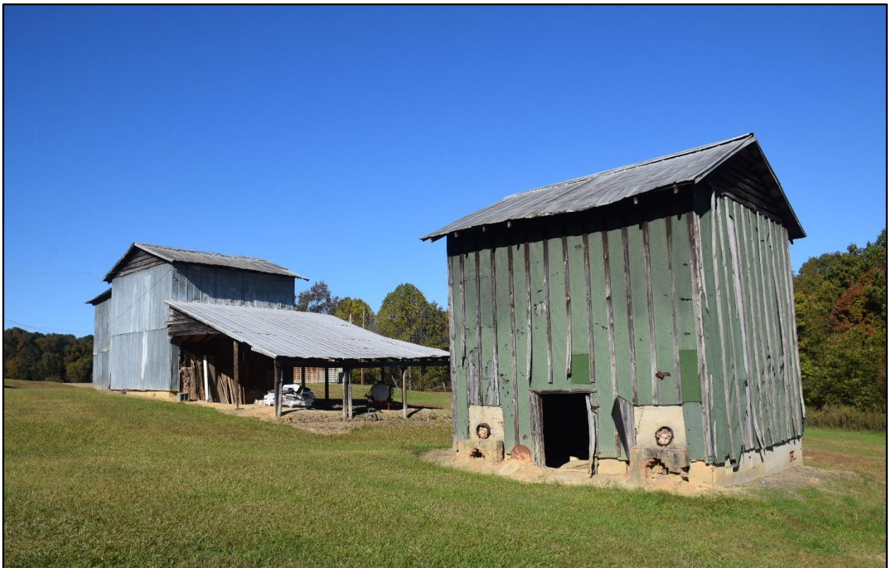
Figure 19- Facing northwest toward former ca. 1930 tobacco barns.
