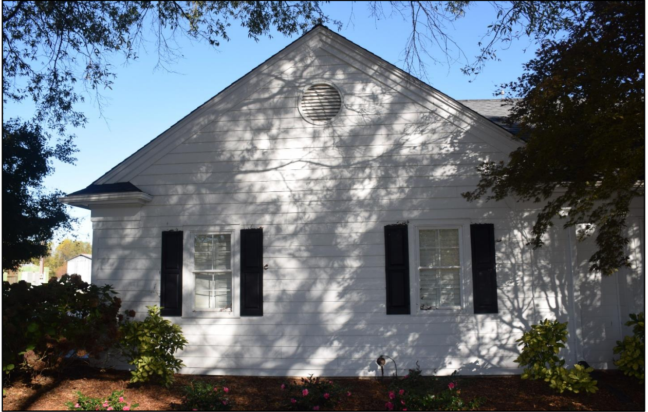
Figure 8- Main House- Facing north toward façade.
