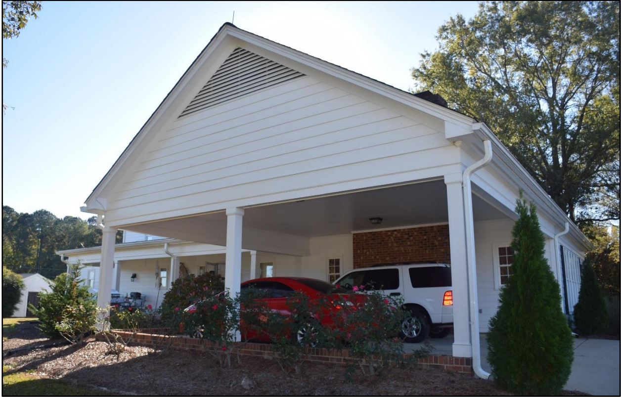
Figure 10- Main House- Facing southwest toward rear elevation and carport addition.
