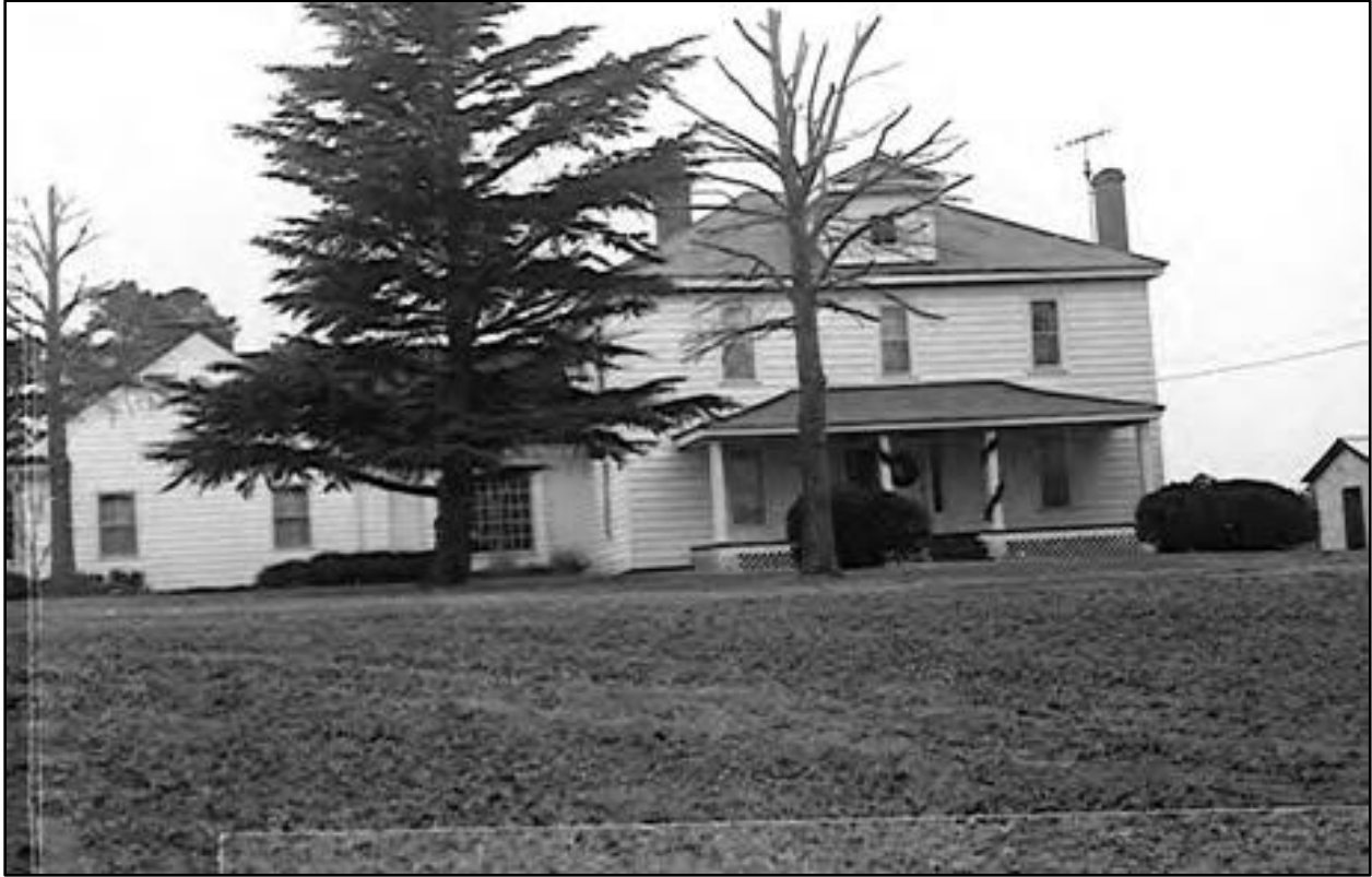
Figure 40- Photograph of Main House ca. 1990. (Source: 1988-1991 Wake County Survey).
