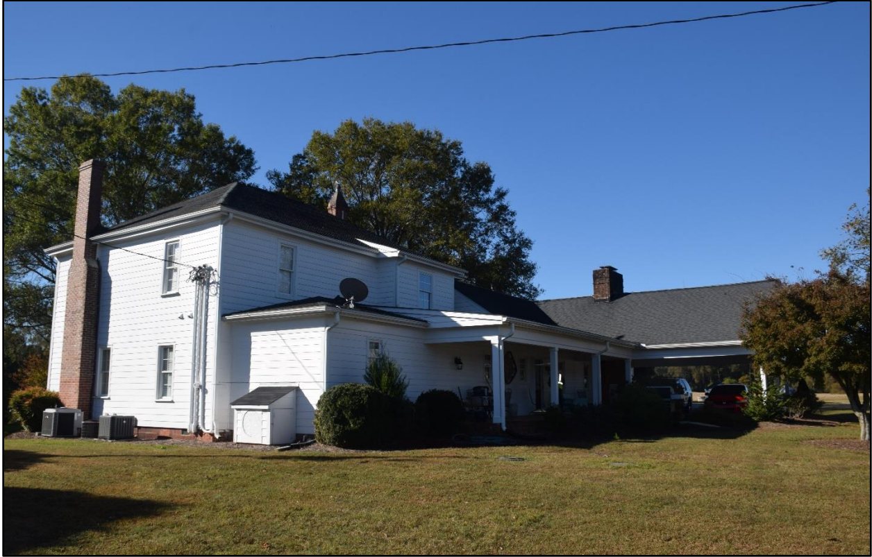
Figure 12- Main House- Facing southeast toward rear elevation and east elevation.
