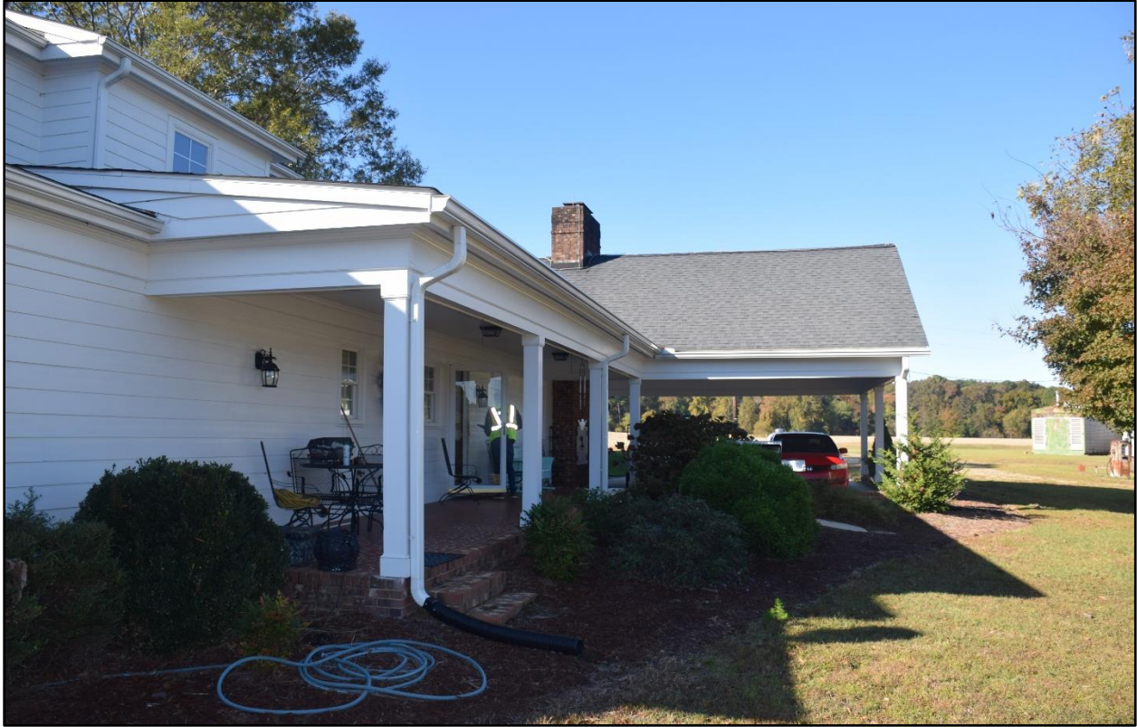
Figure 14- Main House- Facing west along rear elevation.
