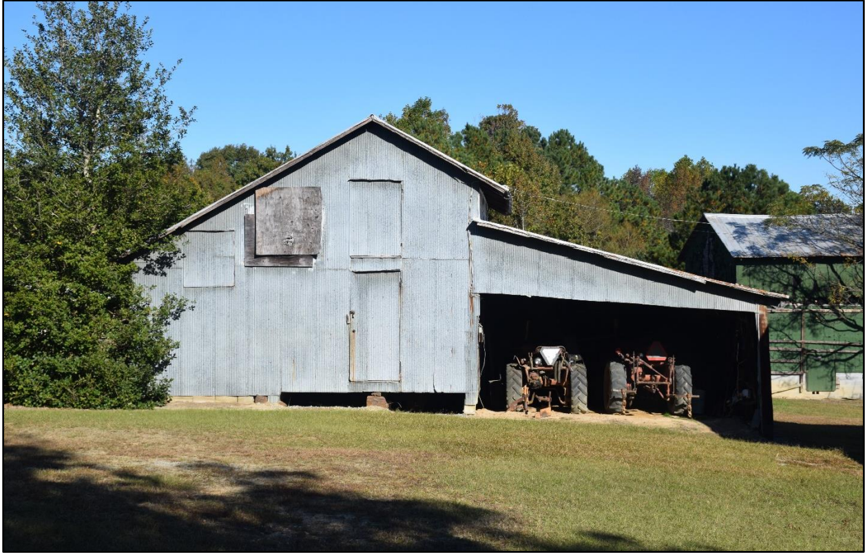
Figure 22- Facing north toward 1959-1964 equipment barn.
