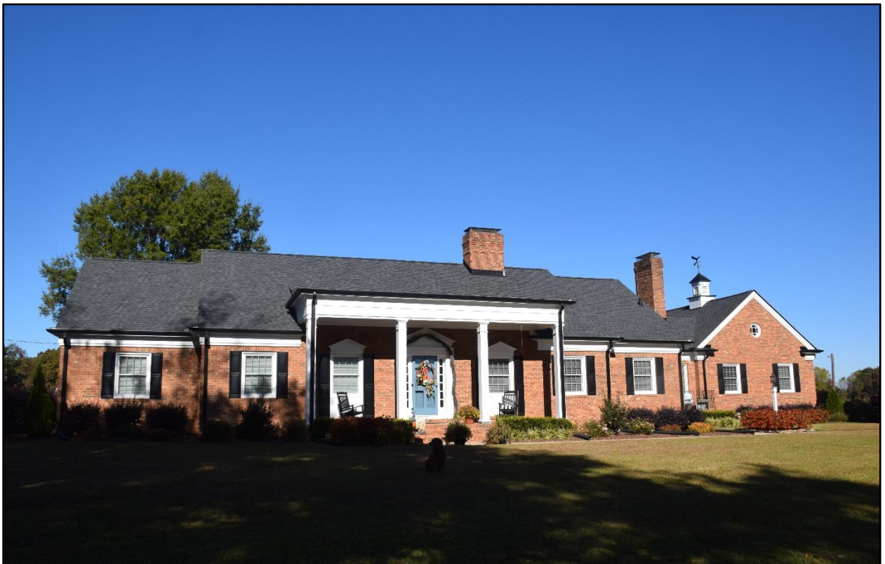
Figure 31- 1963 House (WA7502)- Facing north toward façade.
