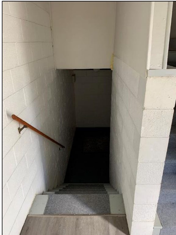
Photo 18: Side entrance leading to basement level.
