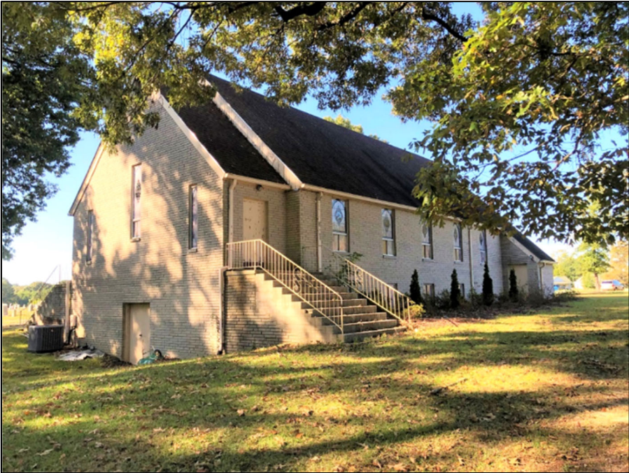
Photograph 9: East (rear) and north elevations, oblique view, view southwest.
