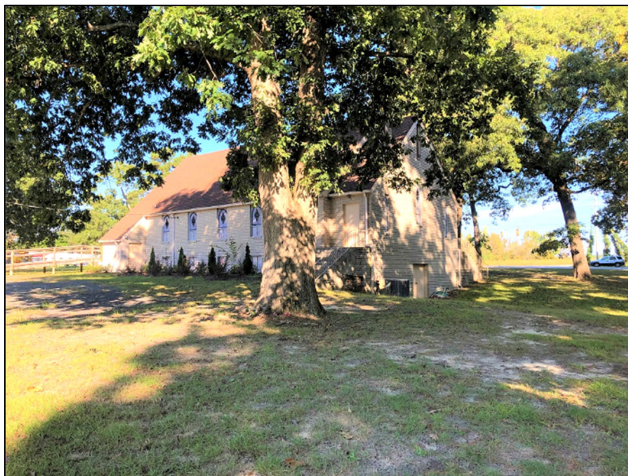
Photograph 7: South and east (rear) elevations, oblique, view northwest.
