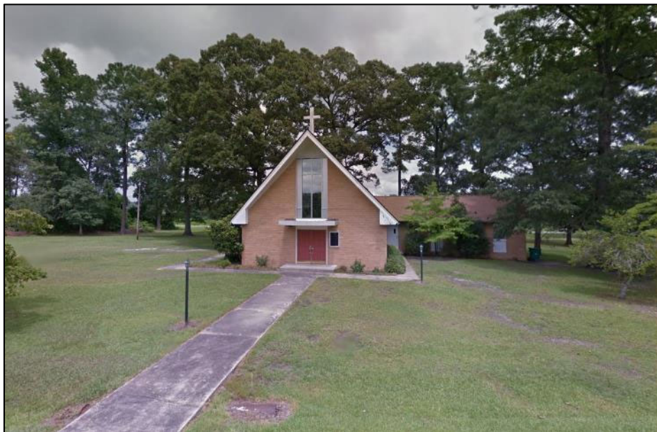
Figure 6: Christ the King Catholic Church (CB0182), 100 Burns Road, Riegelwood, NC. Front-gabled brick building constructed in 1950 with a one-story rear wing. 32 (Google Street View August 2012)
