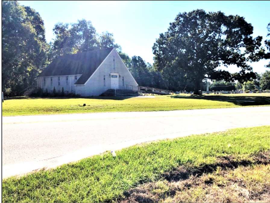
Photograph 2: View southeast of church and cemetery.
