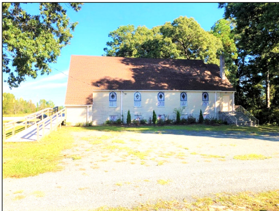
Photograph 6: View north of south elevation.
