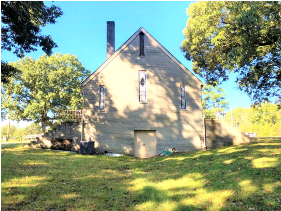
Photograph 8: East (rear) elevation, view west.
