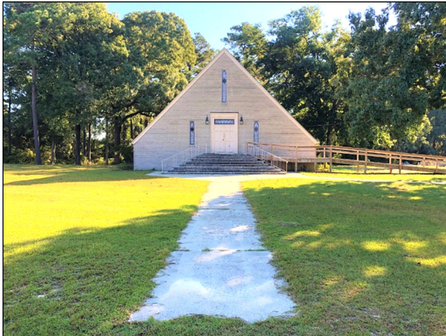
Photograph 4: View east of front entrance and sidewalk. The handicap ramp was added post-2016.
