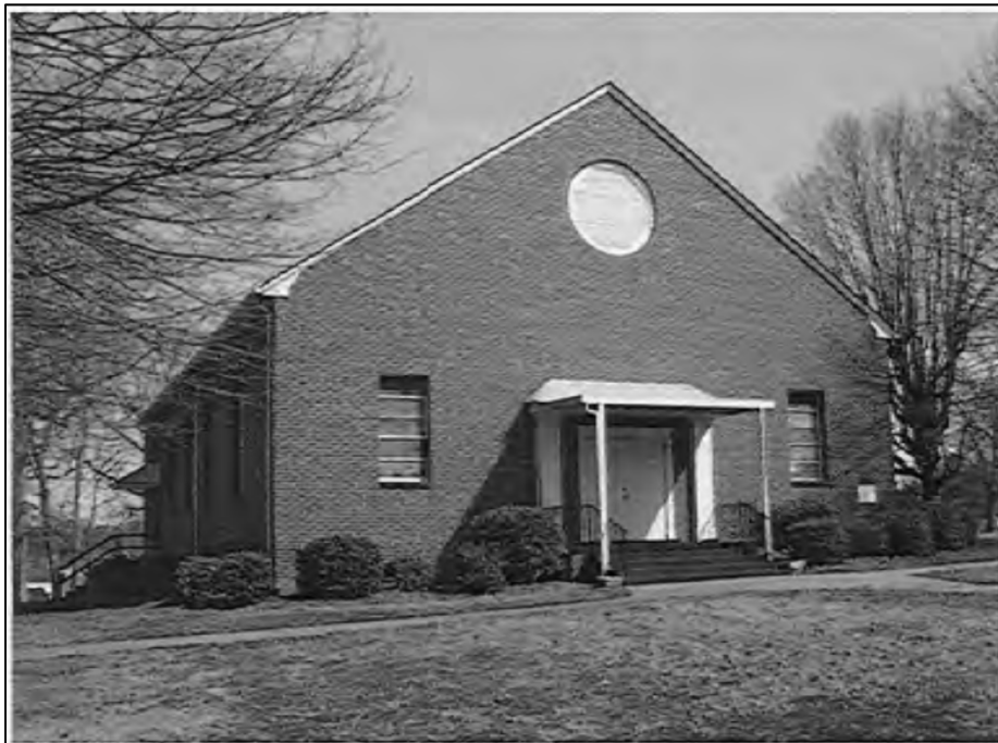
Figure 8: Saint's Delight Primitive Baptist Church (built ca. 1952), Winston-Salem, Forsyth County (FY0314). Built around the same time as Willow Springs Primitive Baptist Church (NC SHPO 2007)
