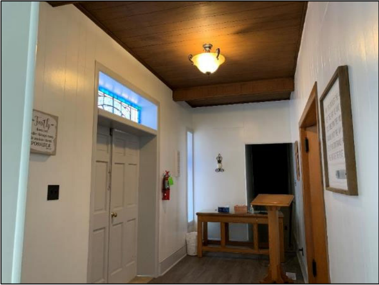
Photo 15: Narthex looking north.
