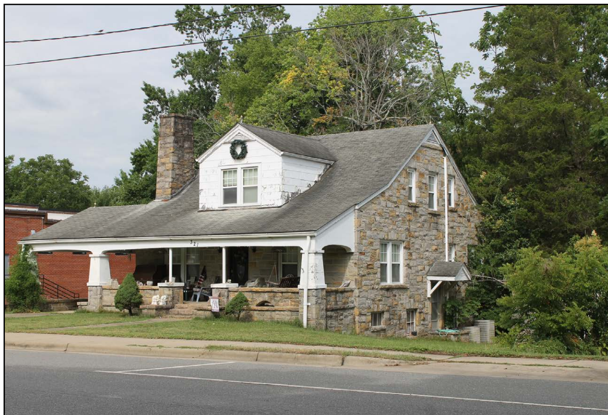
Figure 4.42: House at 321 North First Avenue, Knightdale (WA7678).
