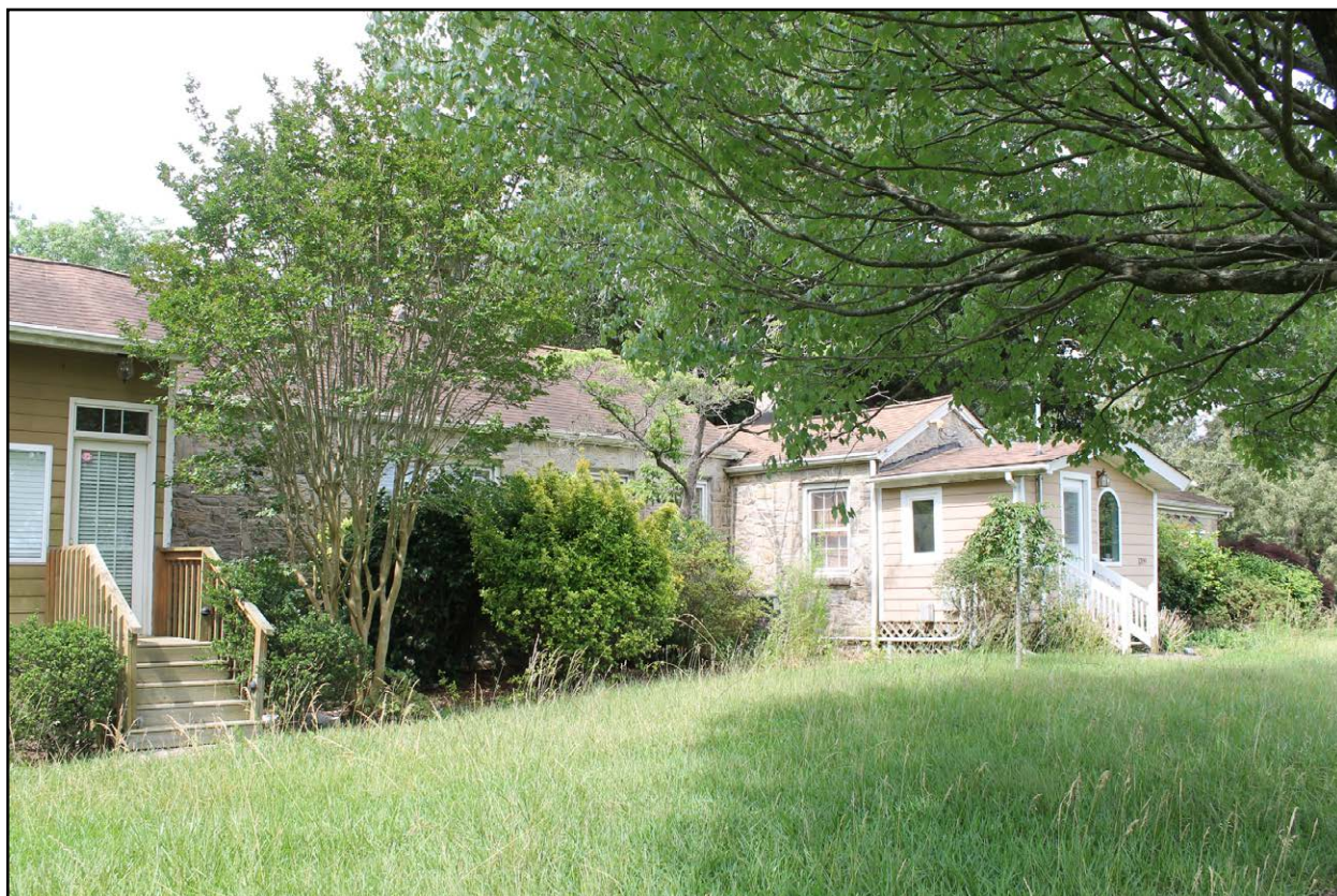
Figure 4.5: Joseph Collier house, view of north side elevation, facing southwest.
