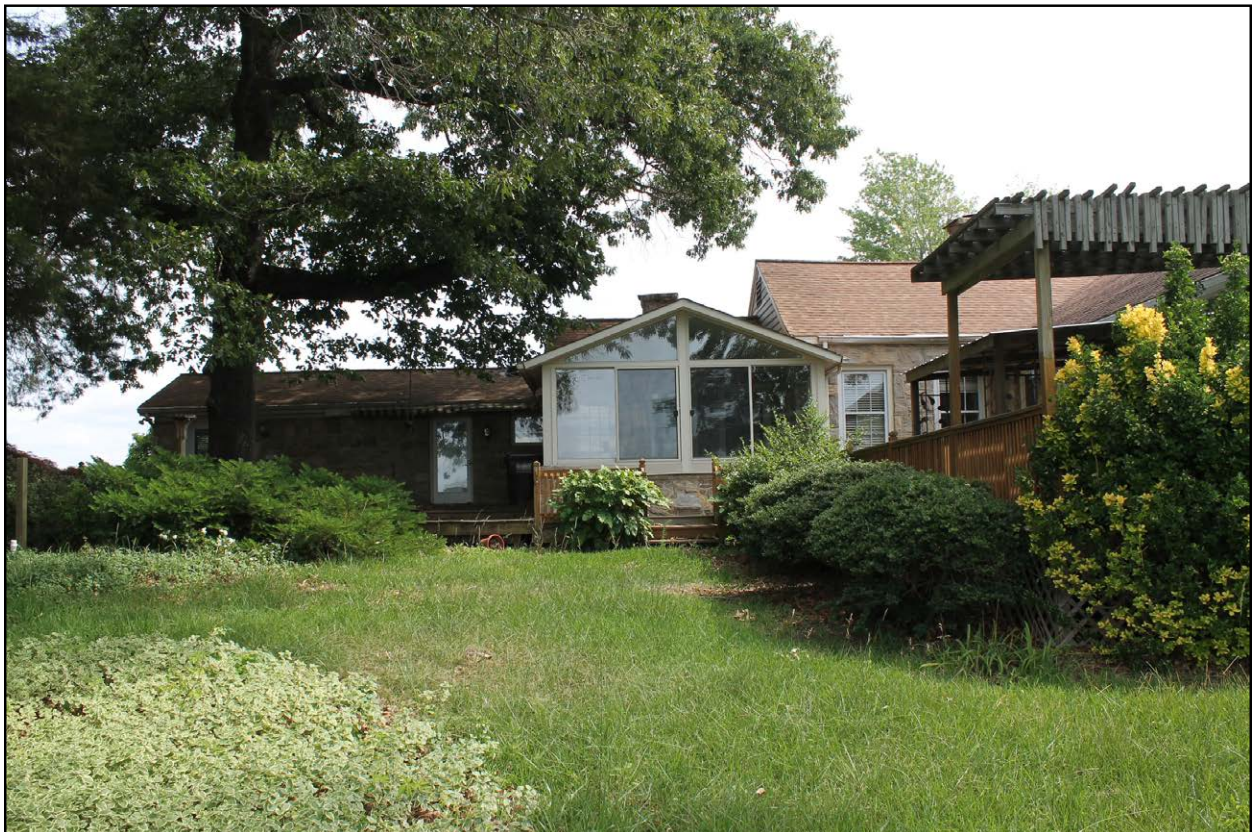
Figure 4.13: Joseph Collier house, view of south elevations of original house and rear wing, facing north.
