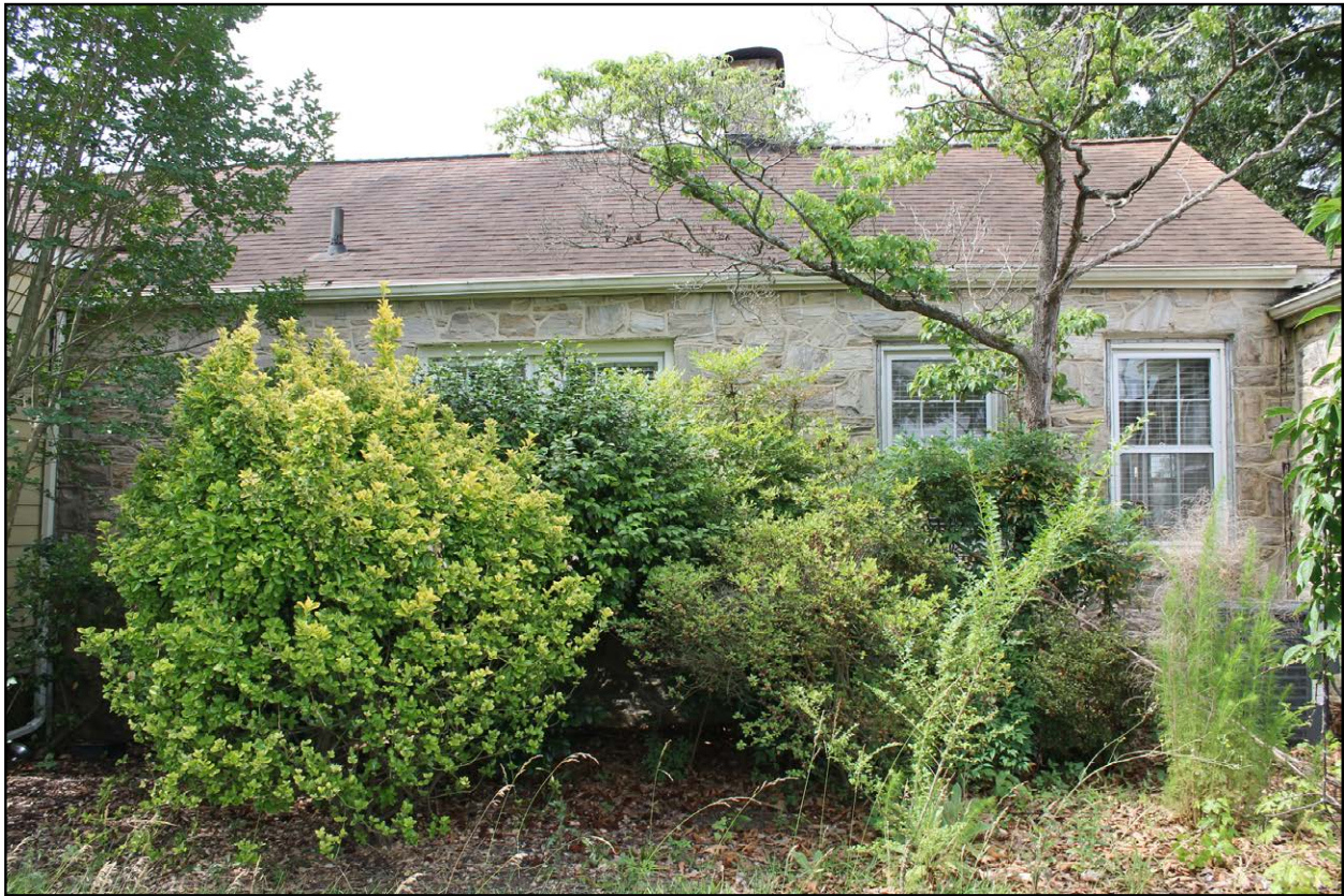
Figure 4.6: Joseph Collier house, view of portion of original north side elevation, facing south.
