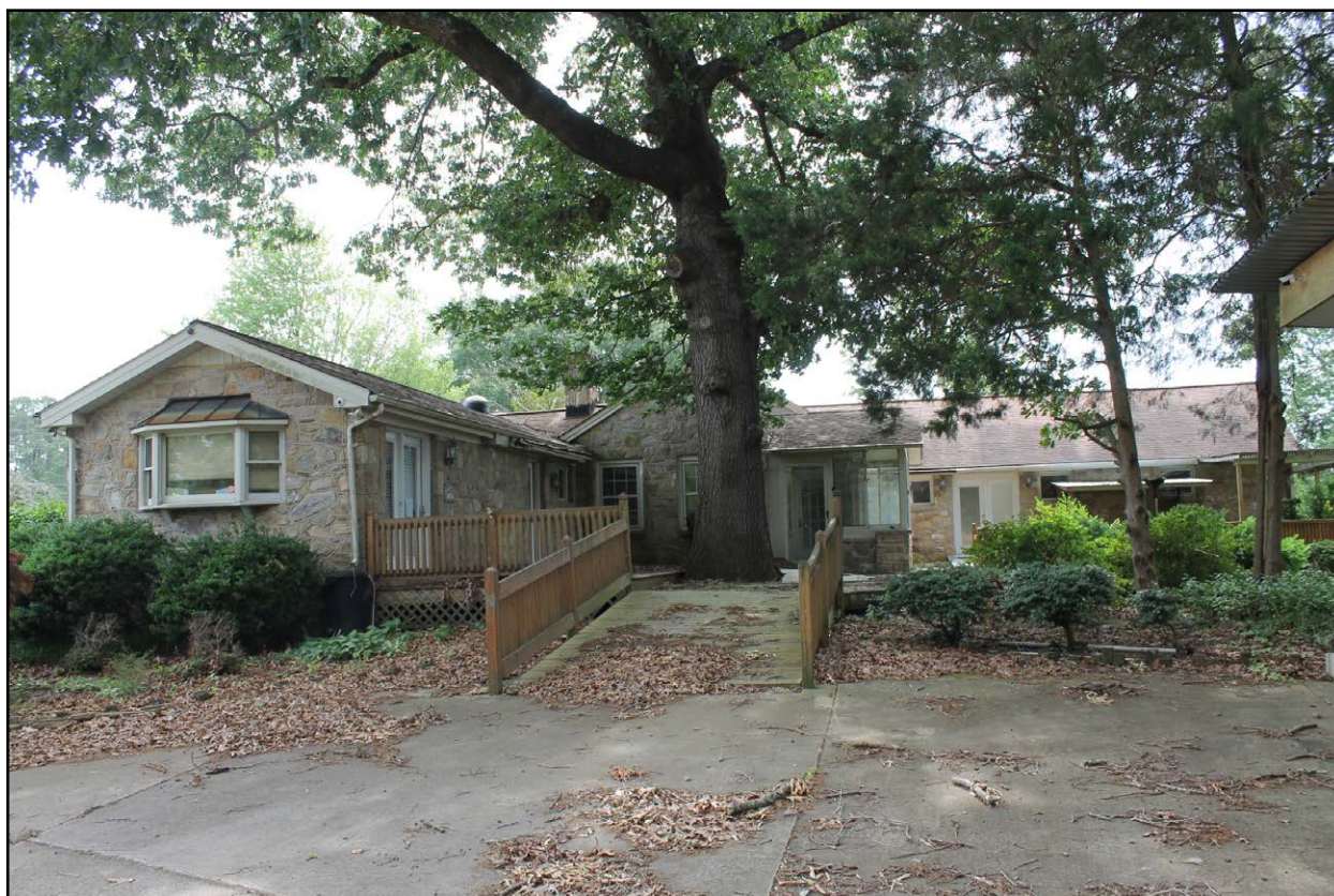
Figure 4.18: Joseph Collier house, view of rear elevation, facing east.
