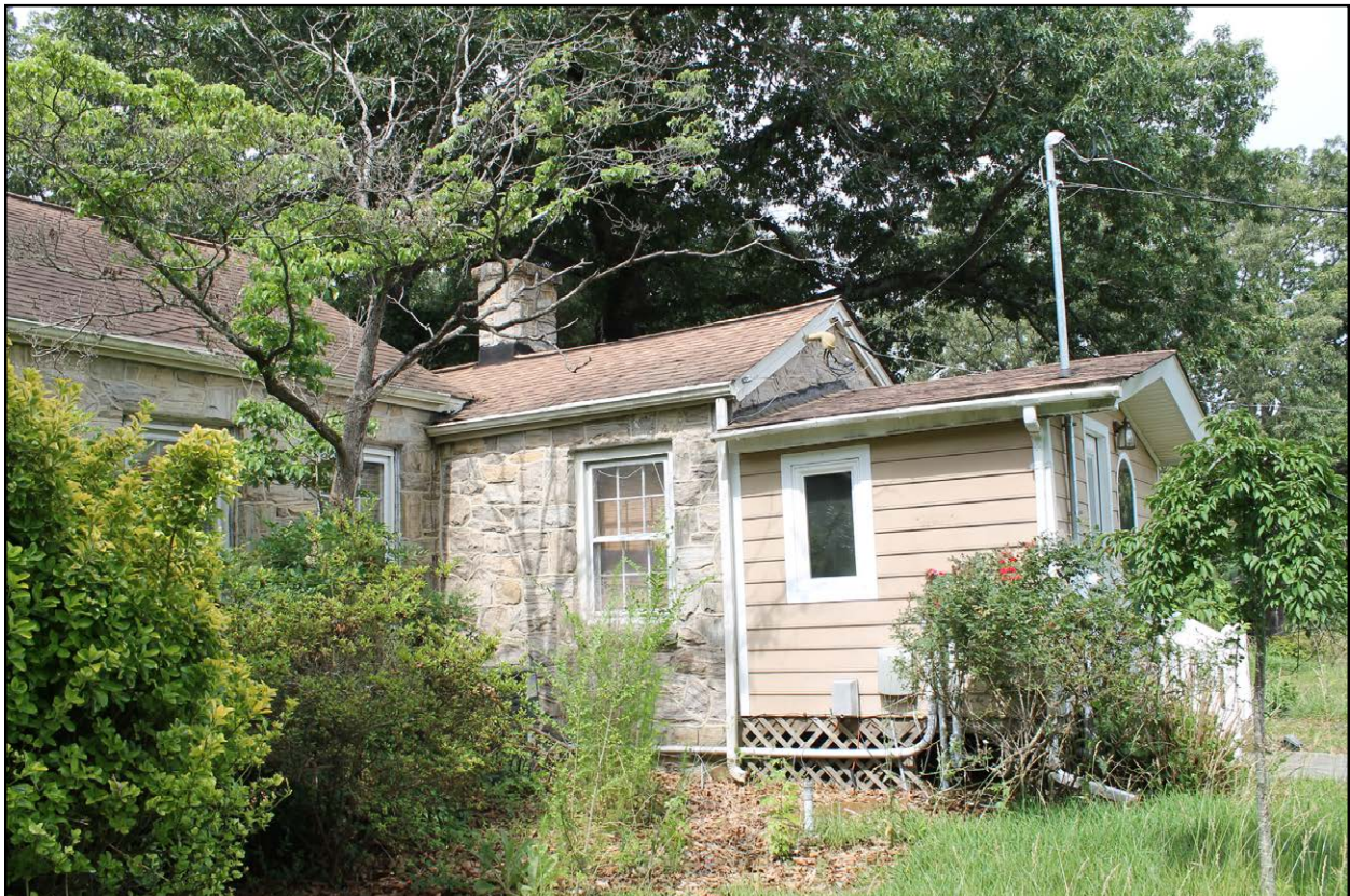
Figure 4.7: Joseph Collier house, view of original entry vestibule on north side elevation, facing southwest.
