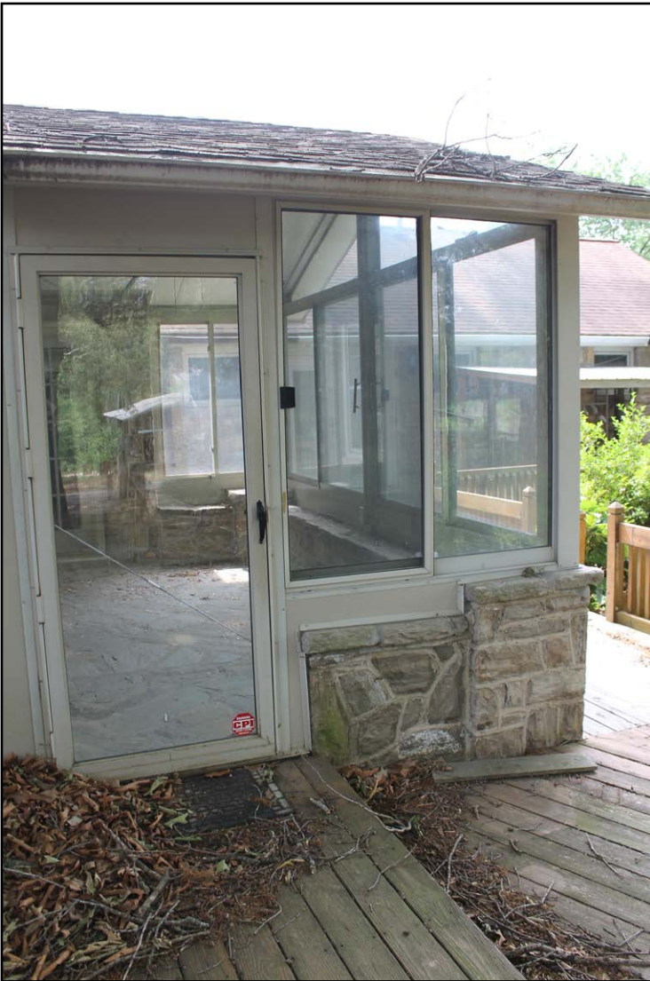
Figure 4.15: Joseph Collier house, view of original side porch piers, facing east.
