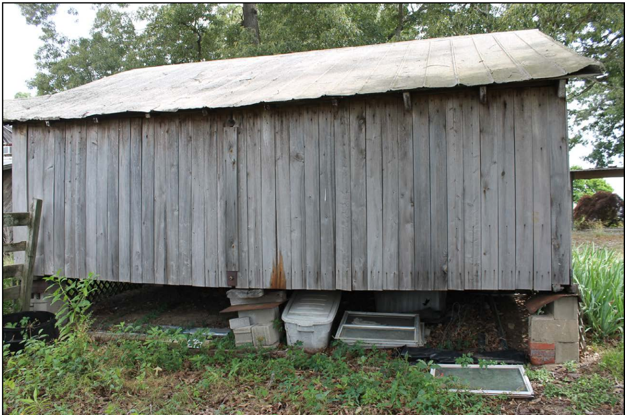
Figure 4.22: Storage building, view of south side elevation, facing north.
