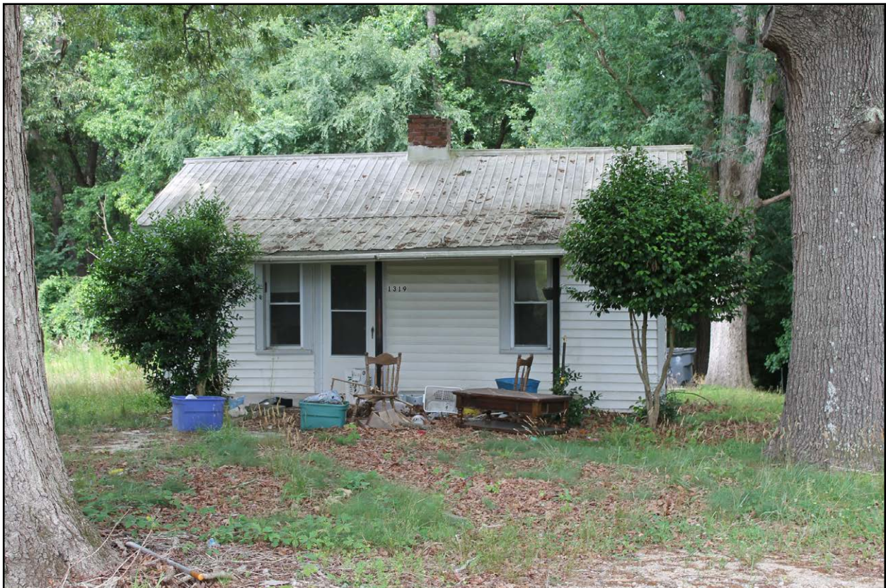
Figure 4.26: Tenant House #1, view of façade (east elevation), facing west.
