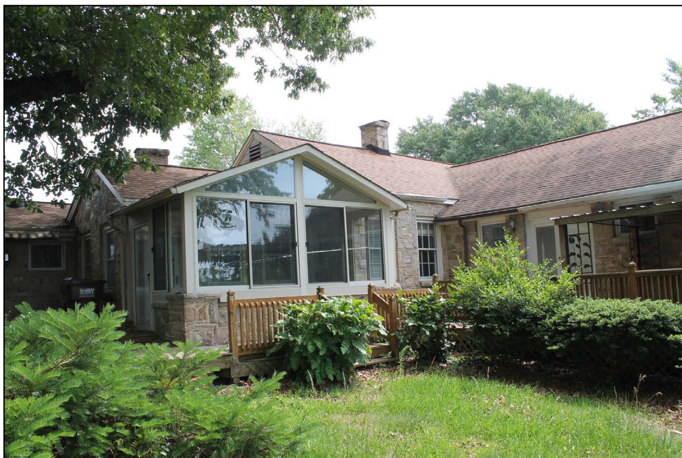
Figure 4.14: Joseph Collier house, view of original side porch with later glass enclosure, facing northeast.
