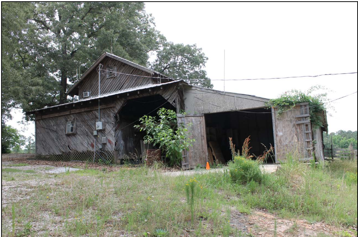
Figure 4.24: Barn converted to dwelling, view of north side elevation, facing southeast.
