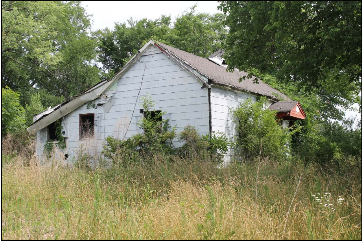
Figure 4.30: Tenant House #2, view facing northwest.
