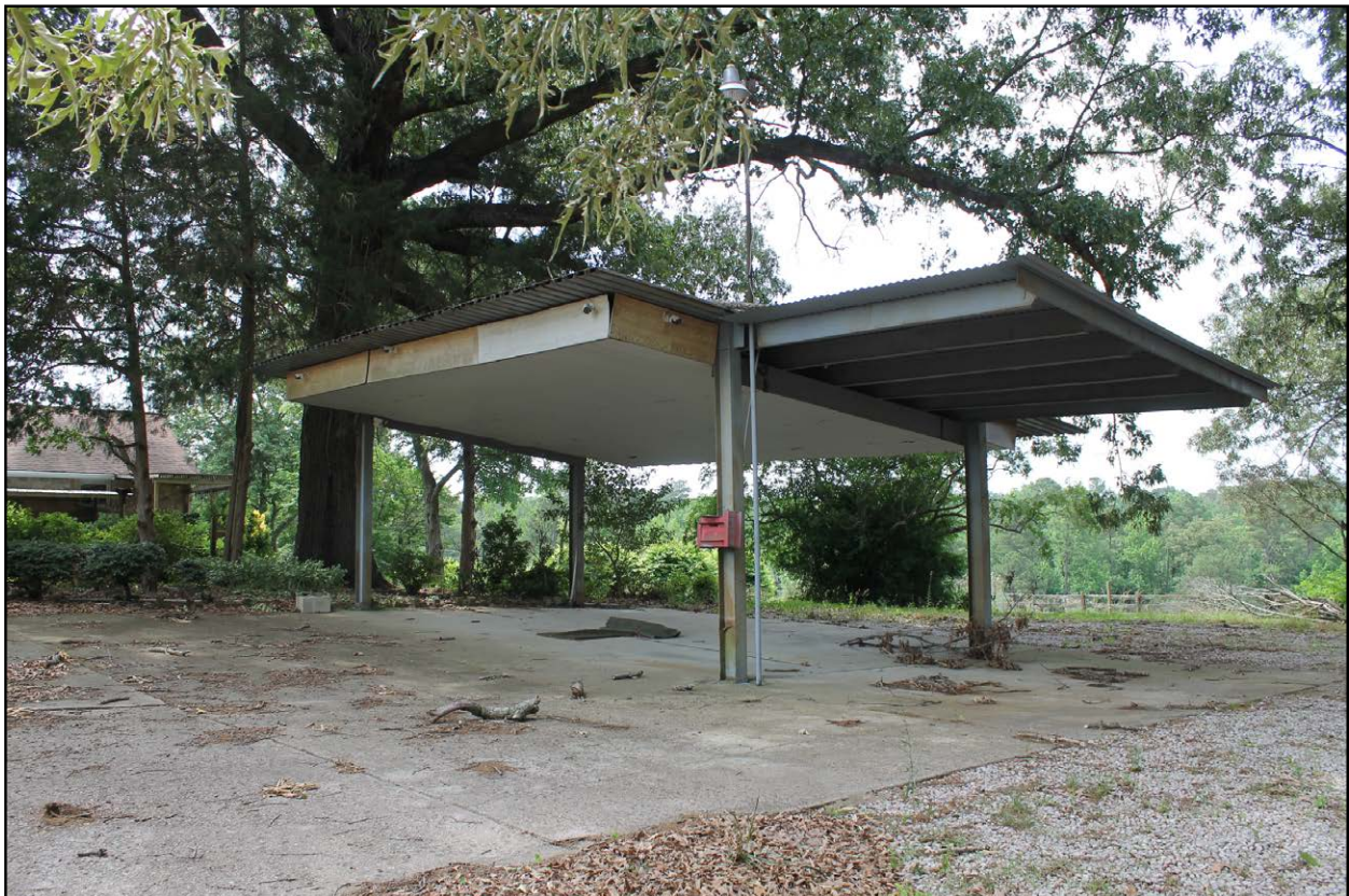
Figure 4.20: Carport, view facing southeast.
