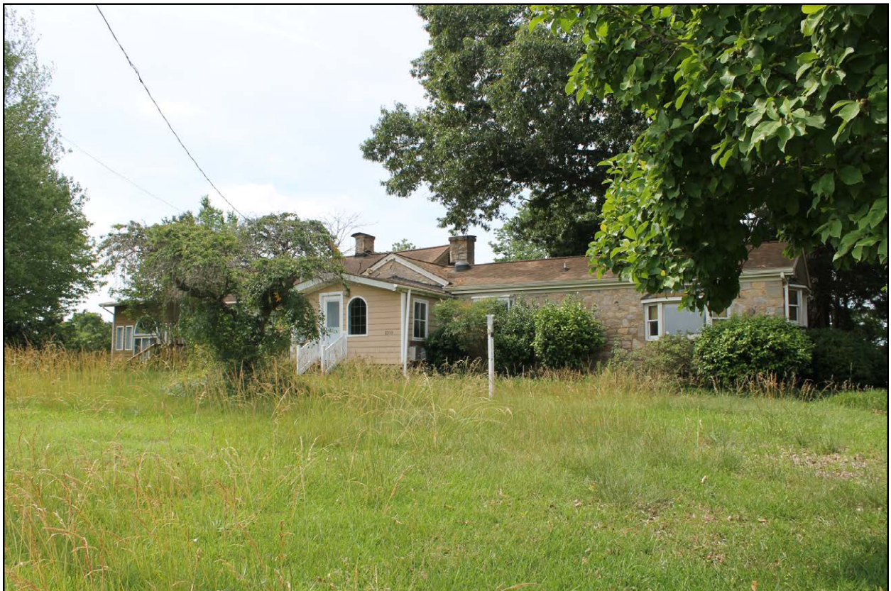
Figure 4.9: Joseph Collier house, view of north side elevation showing rear wing addition, facing south.
