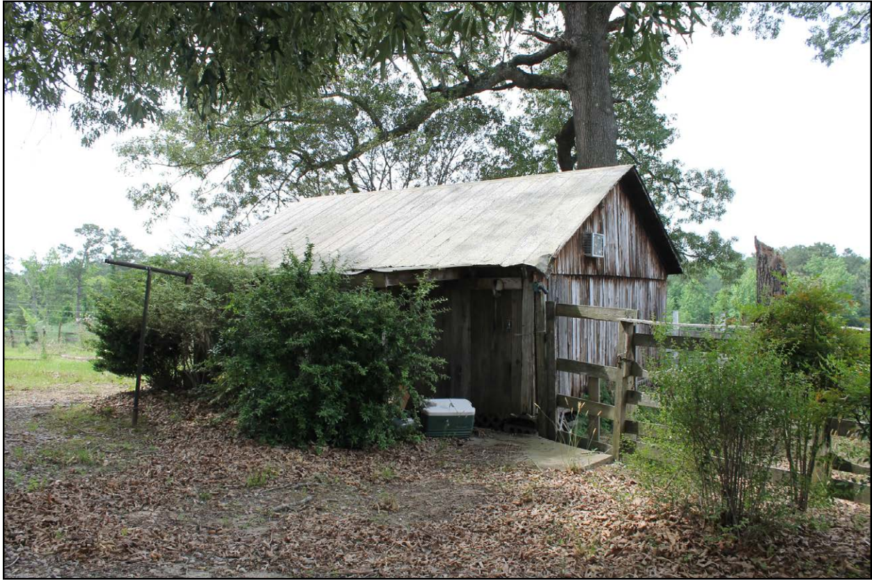
Figure 4.21: Storage building, view of north side elevation, facing southeast.
