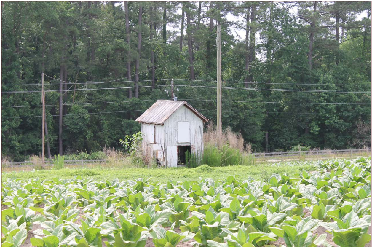
Figure 4.31: Outbuilding, view facing east.
