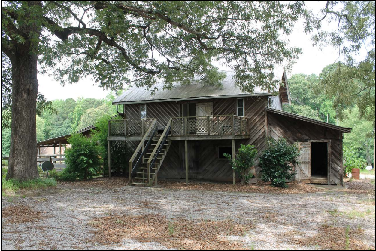
Figure 4.23: Barn converted to dwelling, view of east elevation, facing west.
