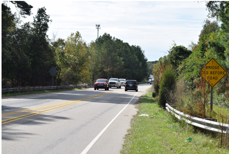
NC 50 (Benson Road) from Bridge No. 25 over Swift Creek, view to the south
