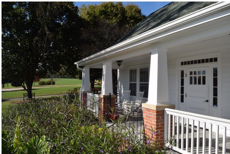
Rebuilt porch with replacement posts and altered plinths, view to the south
