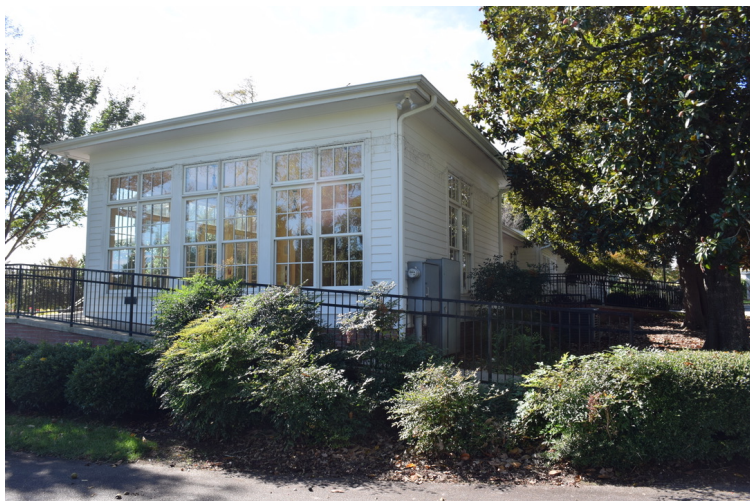
North end of ballroom, view to the south-southeast
