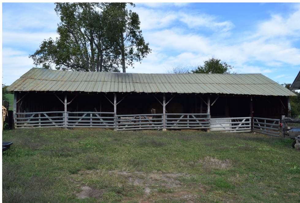
Equipment shed or lounging barn, view to the north
