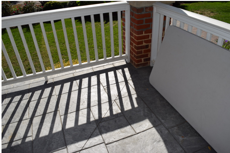
Modern porch floor and alerted brick plinths, view to the east
