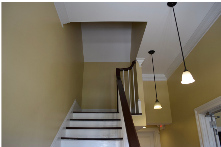
Center hall stair has been blocked with drywall to prevent public access to upper level, view to the west
