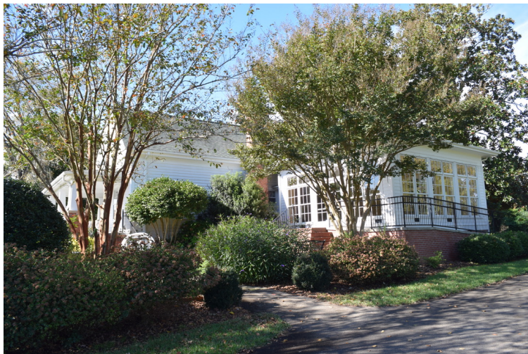
Northeast (front) corner, view to the southwest
