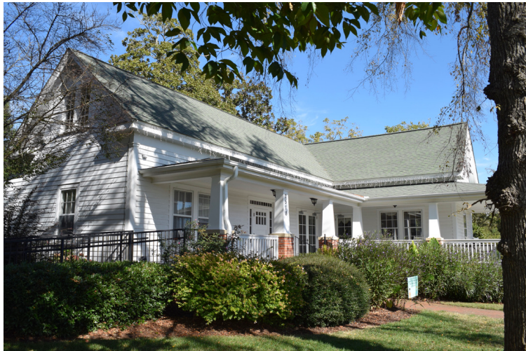
Southeast (front) corner, view to the northwest
