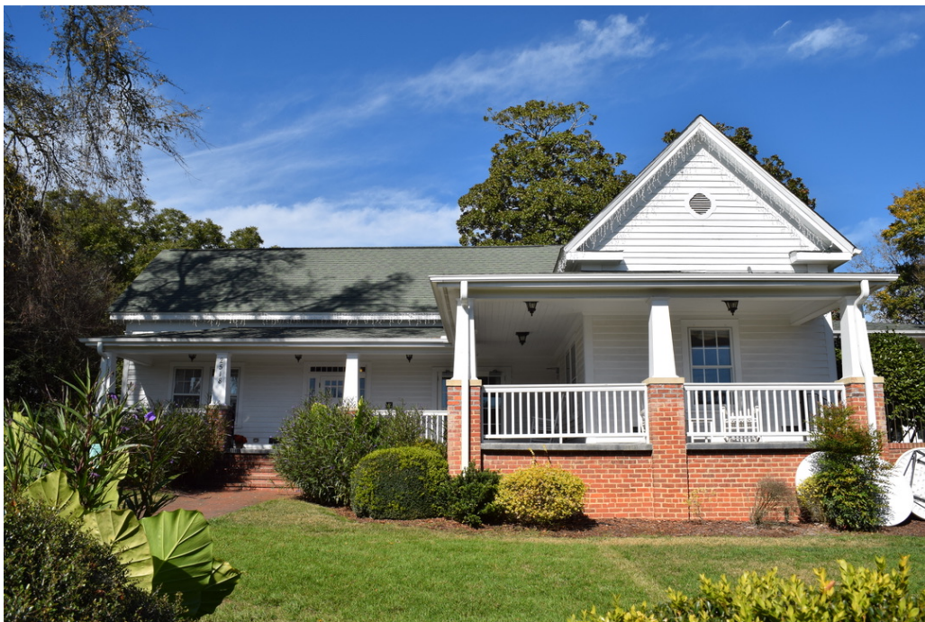
Rand-Bryan House facade, view to the west
