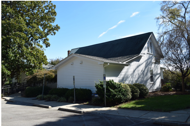
Southwest (rear) corner, view to the east-northeast
