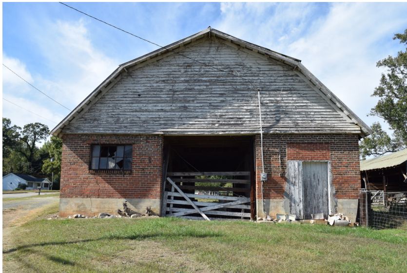
East end, view to the west
