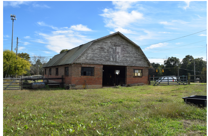
Brick dairy barn, view to the southeast
