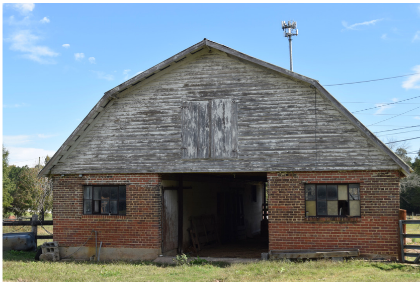
West end, view to the east
