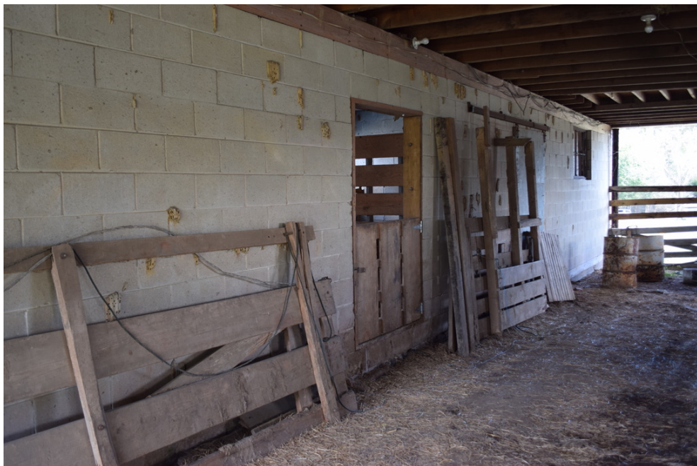
Concrete block wall installed in the 1950s or 1960s, view to the east
