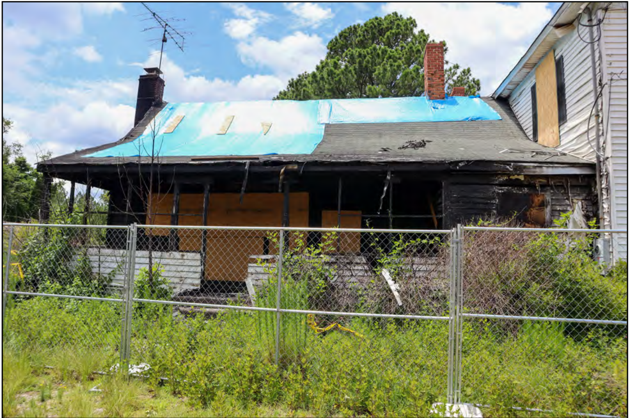
Figure 4.6: View of the primary (east) elevation of the circa-1810 section of the Hunter-Prince House.
