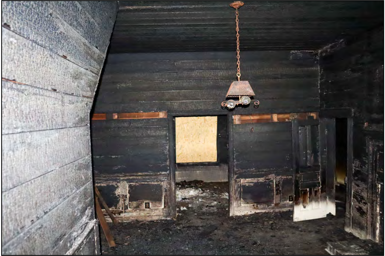
Figure 4.24: Interior view of the parlor of the circa-1810 section of the Hunter-Prince House looking west. Note the staircase on the left side of the photo and the wainscoting along the west wall of the parlor.
