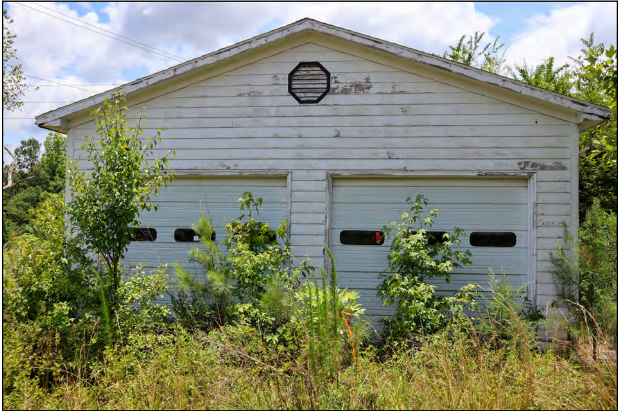
Figure 4.32: View of the primary (north) elevation of the garage.
