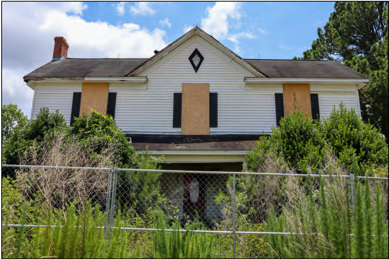
Figure 4.4: View of the primary (north) elevation of the Hunter-Prince House.
