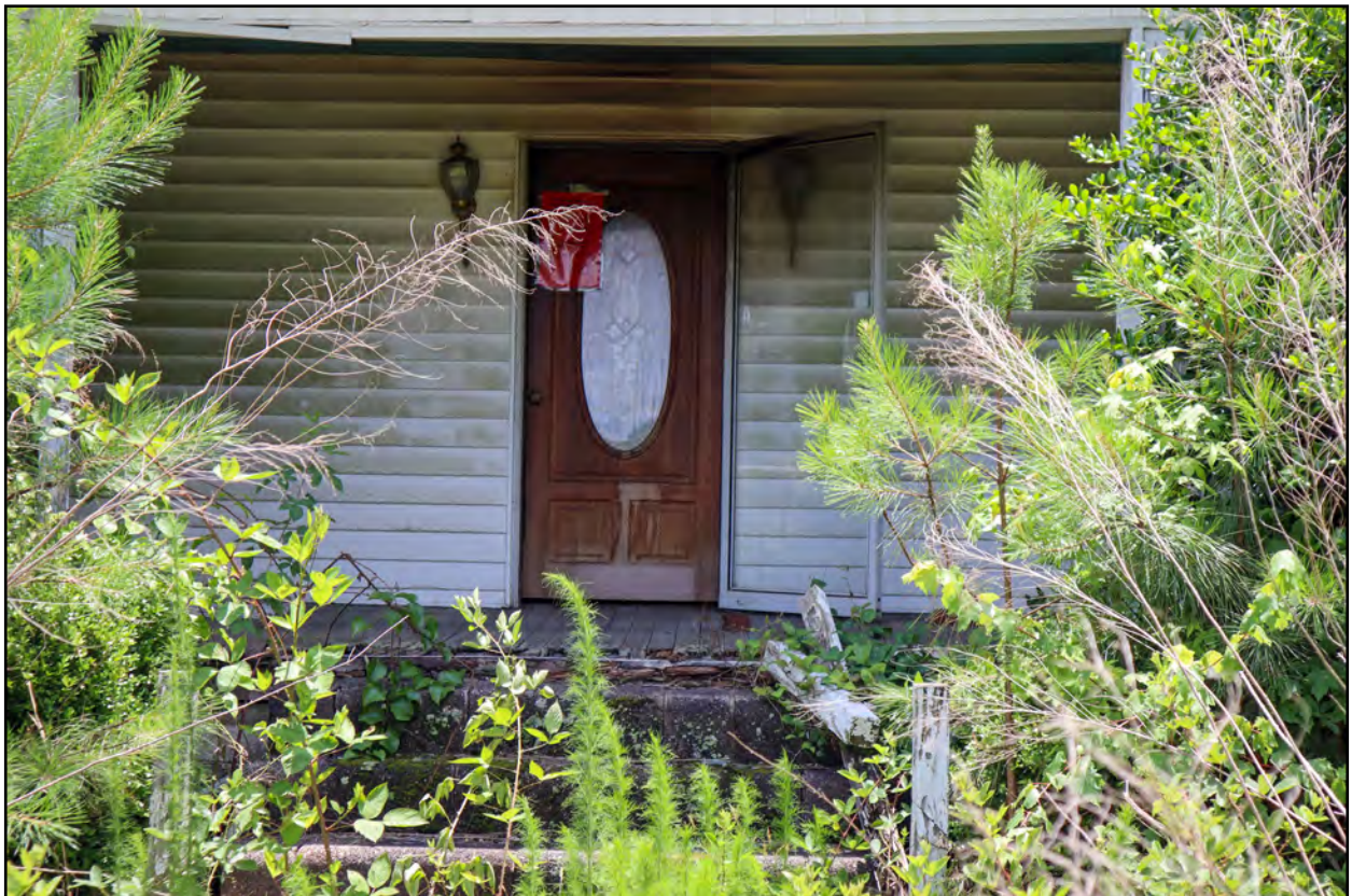
Figure 4.13: Detail view of the replacement front door to the Hunter-Prince House on the primary (north) elevation.
