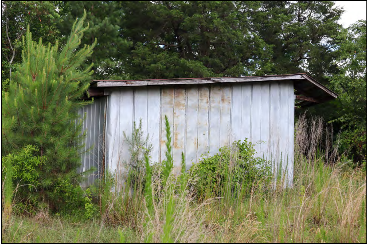
Figure 4.40: View of the west elevation of the storage shed.
