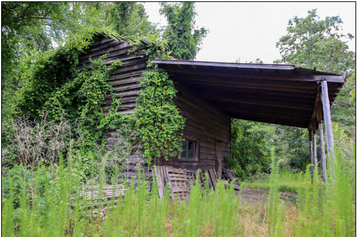
Figure 4.35: View of the west elevation of the barn.
