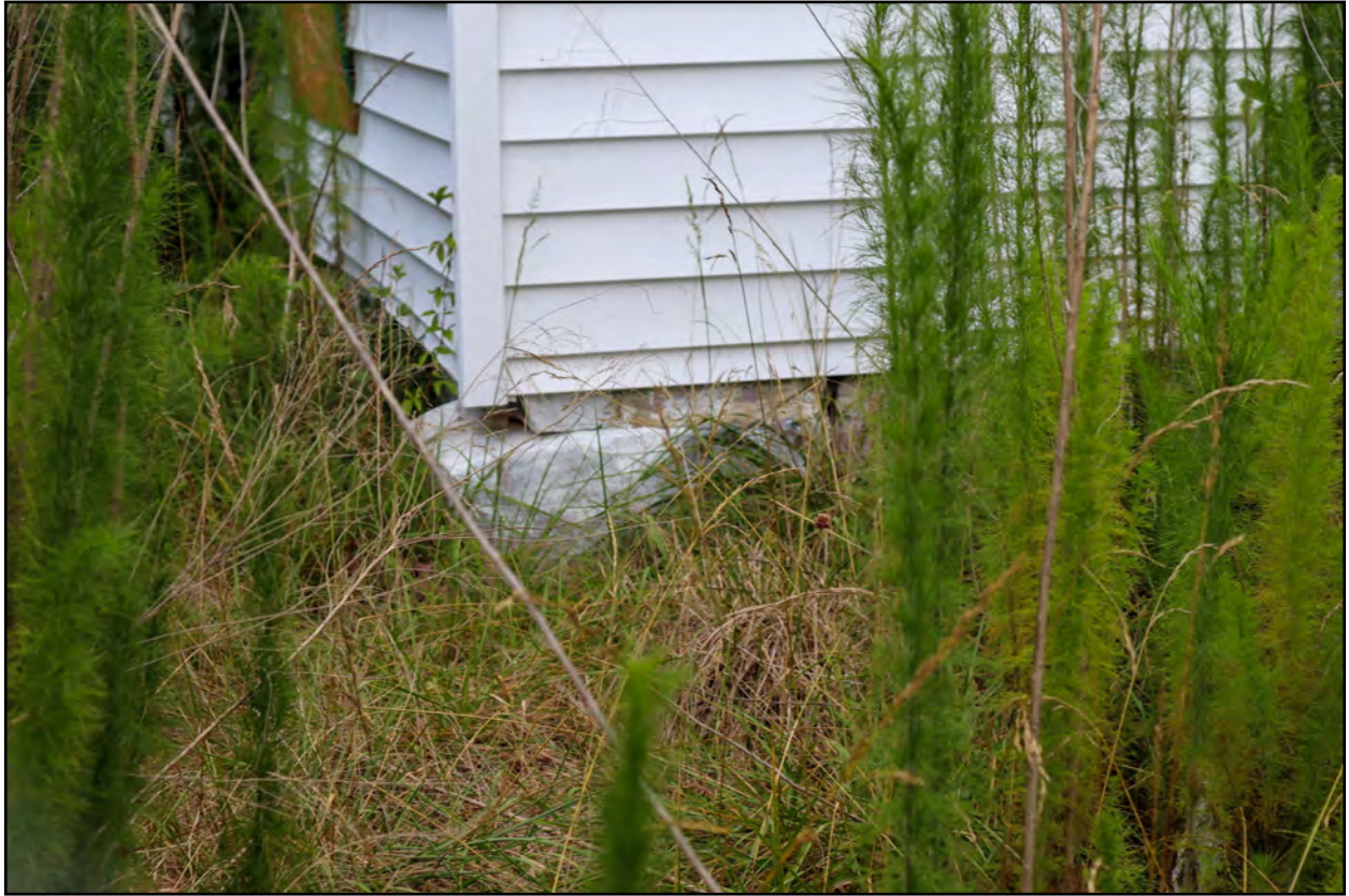
Figure 4.22: View of the stone foundation on which the southwest corner of the circa-1810 section of the Hunter-Prince House sits.
