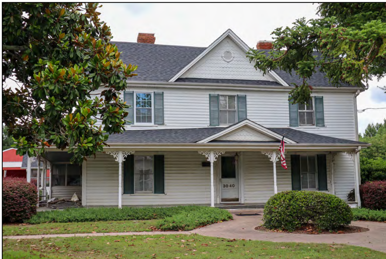
Figure 4.65: The William Henry Carpenter House (WA0754).
