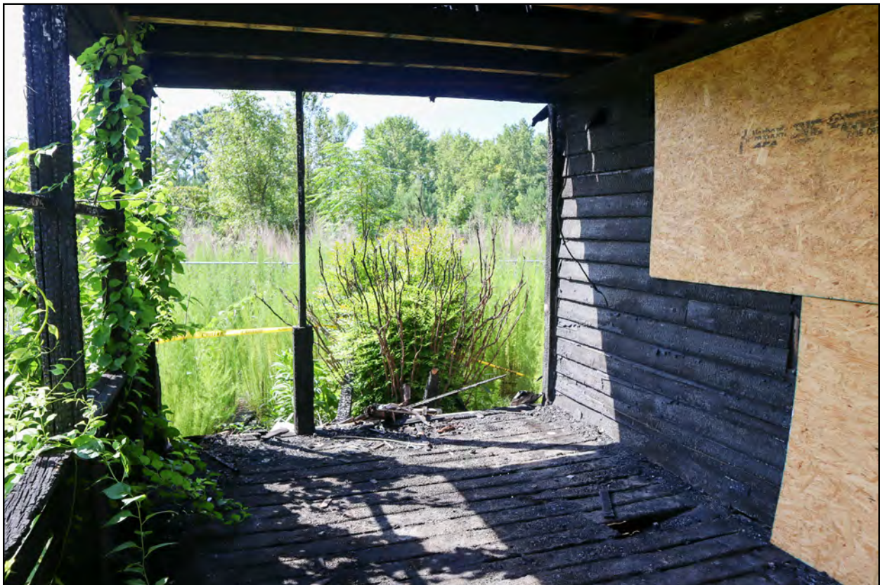
Figure 4.19: Detail view of the front porch on the circa-1810 section of the Hunter-Prince House looking south.
