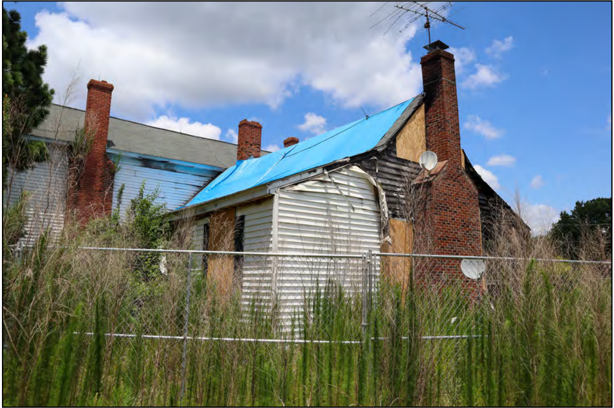
Figure 4.8: View of the south and rear (west) elevations of the circa-1810 section of the Hunter-Prince House.
