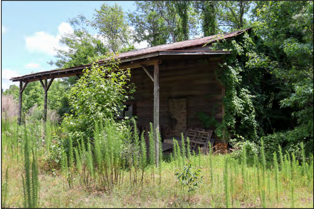
Figure 4.36: View of the north and west elevations of the barn.
