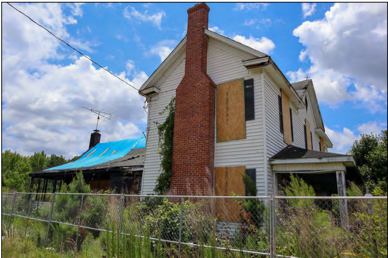
Figure 4.5: View of the east elevation of the Hunter-Prince House.
