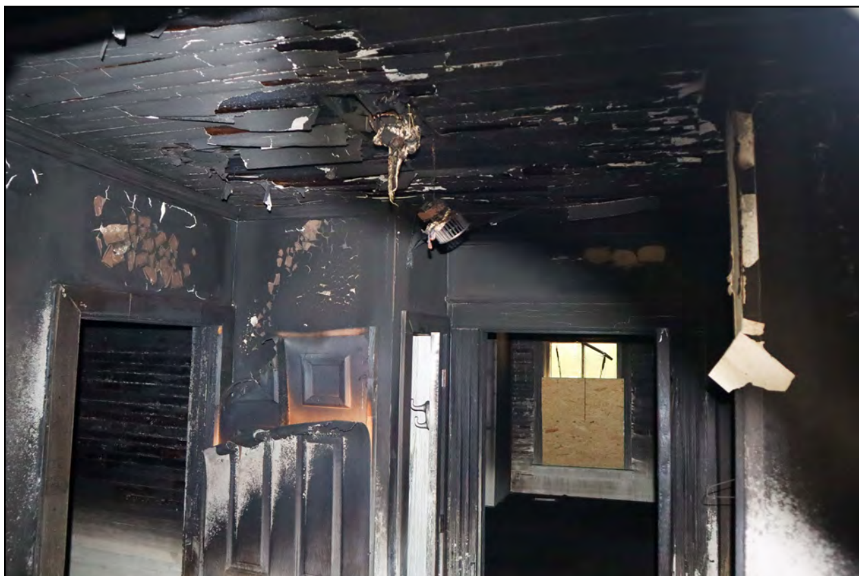
Figure 4.27: Interior view of the I-house section of the house looking north from the porch of the circa-1810 section of the Hunter-Prince House.
