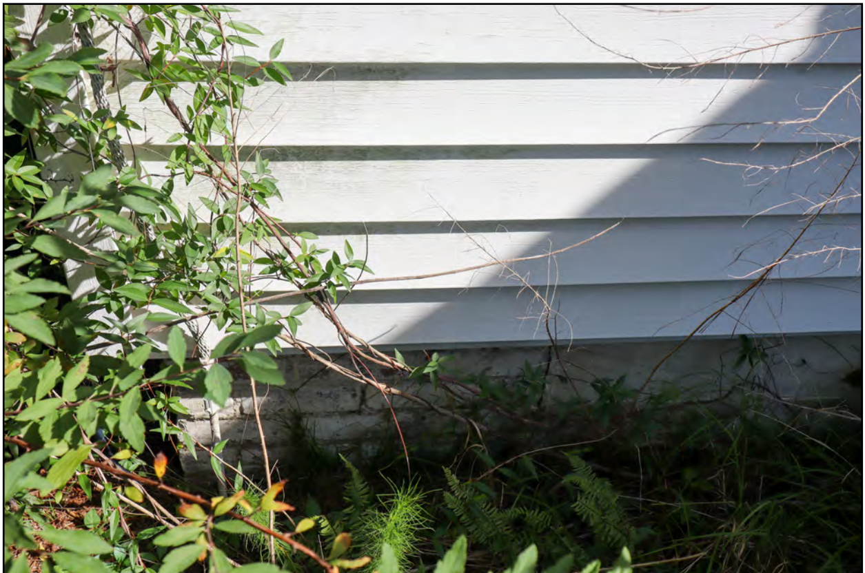
Figure 4.23: View of the brick pier and concrete block foundation that supports the I-house section of the Hunter-Prince House.
