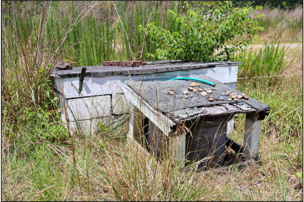
Figure 4.34: View of the wellhouse looking northeast.
