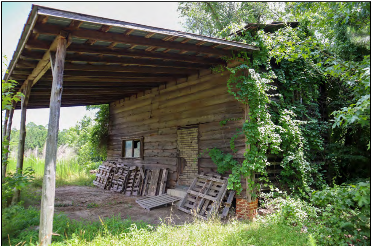
Figure 4.37: Detail view of the north and west elevations of the barn protected by the shed.
