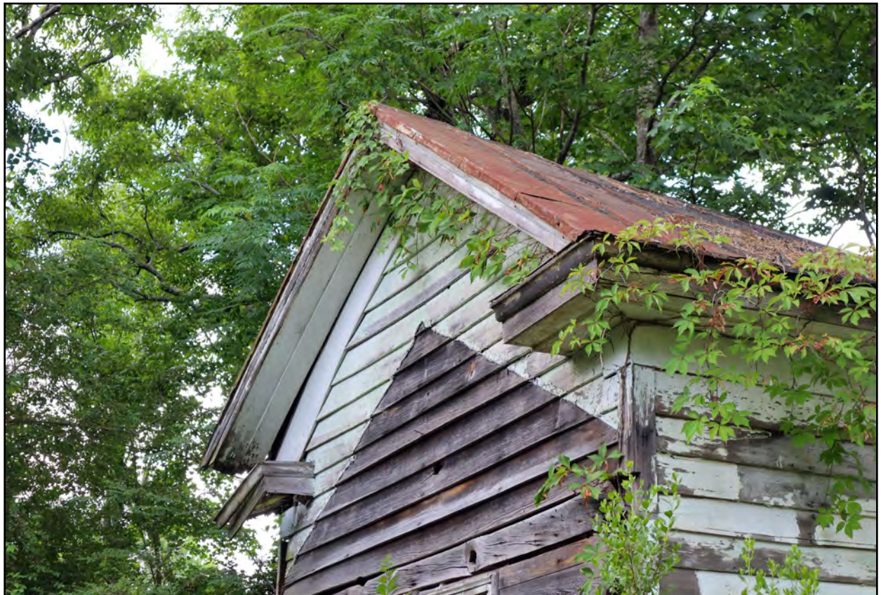
Figure 4.43: Detail view of the east gable-end of the (former) kitchen.
