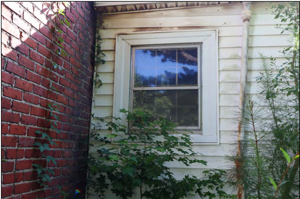
Figure 4.21: View of an intact six-over-six, wood-sash window on the rear (west) elevation of the circa-1810 section of the Hunter-Prince House.
