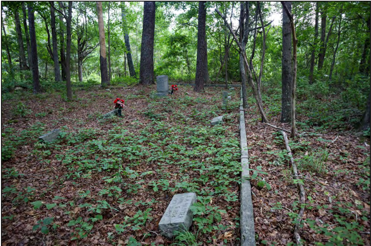
Figure 4.45: Overall view of the west boundary wall of the Hunter Cemetery looking south.
