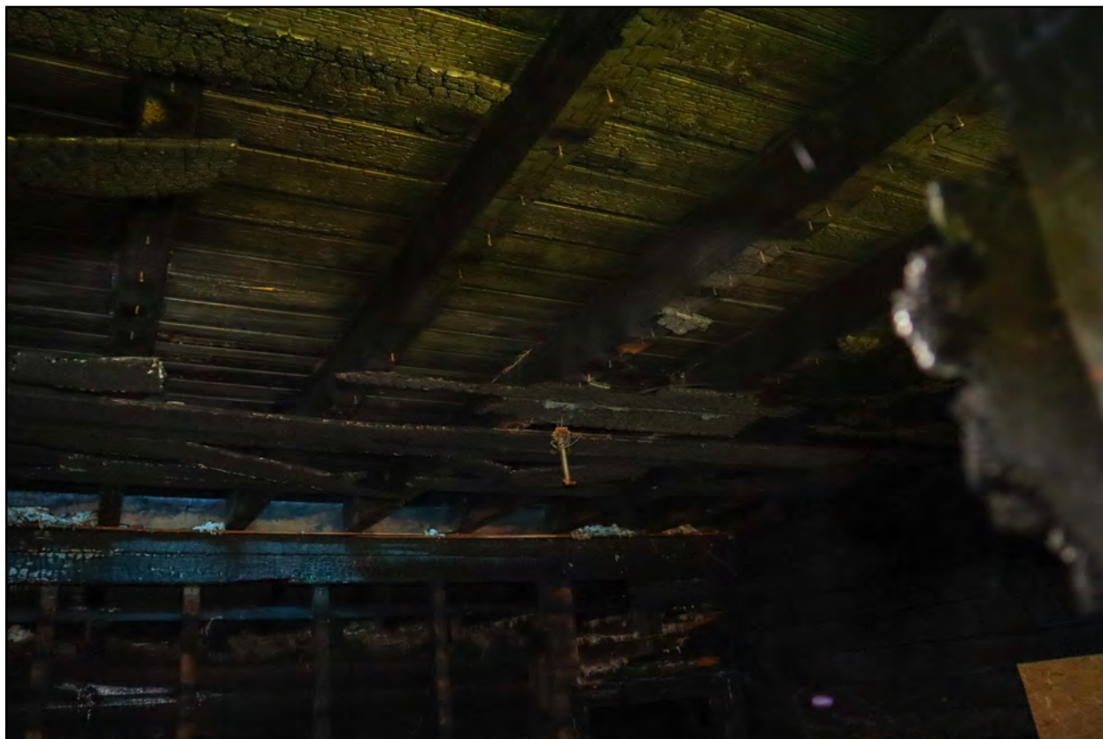
Figure 4.26: Interior view of the ceiling and west wall of hall of the circa-1810 section of the Hunter-Prince House.
