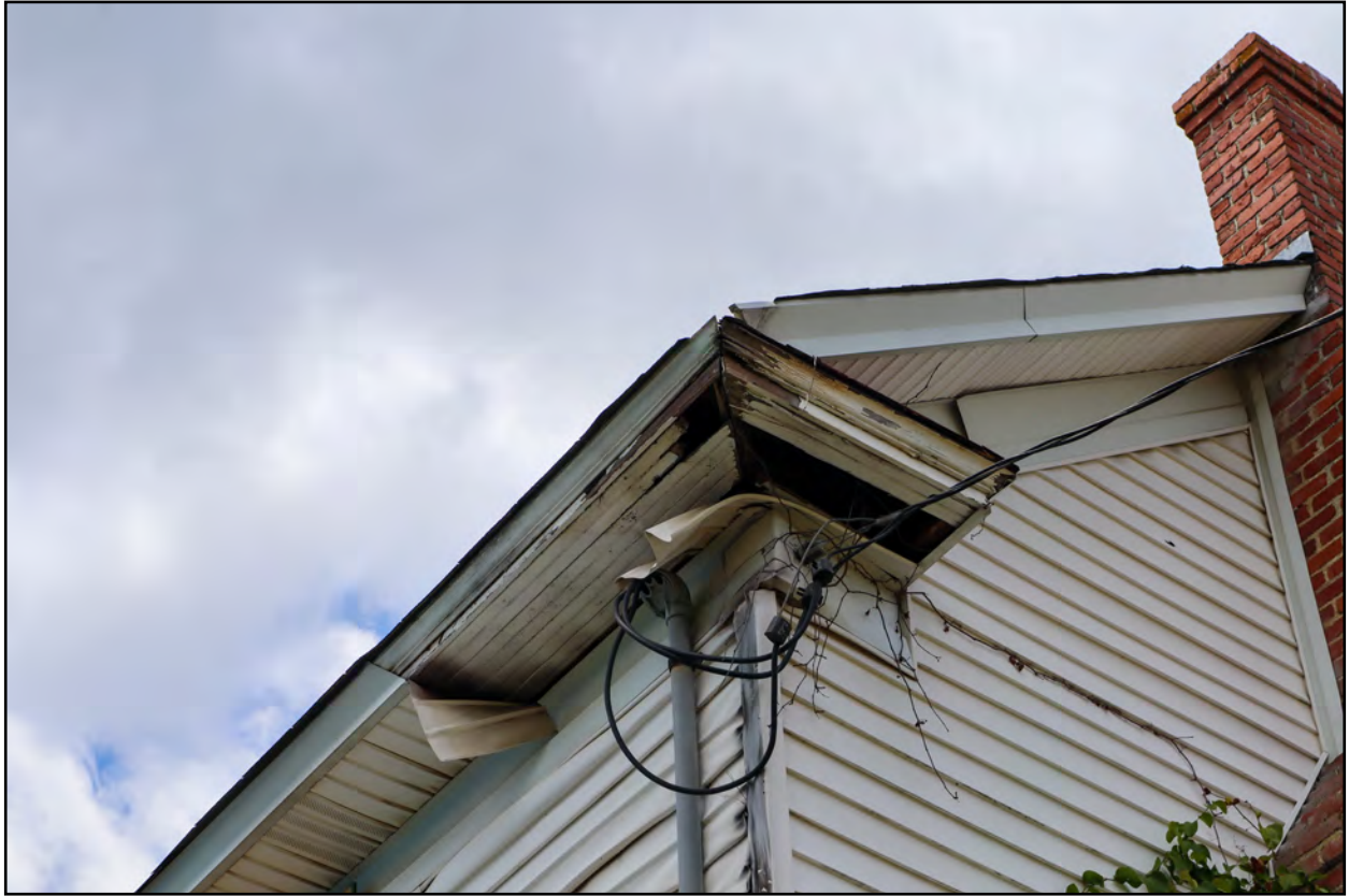
Figure 4.12: Detail view of the gable return on the southeast corner of the I-house section of the Hunter-Prince House.
