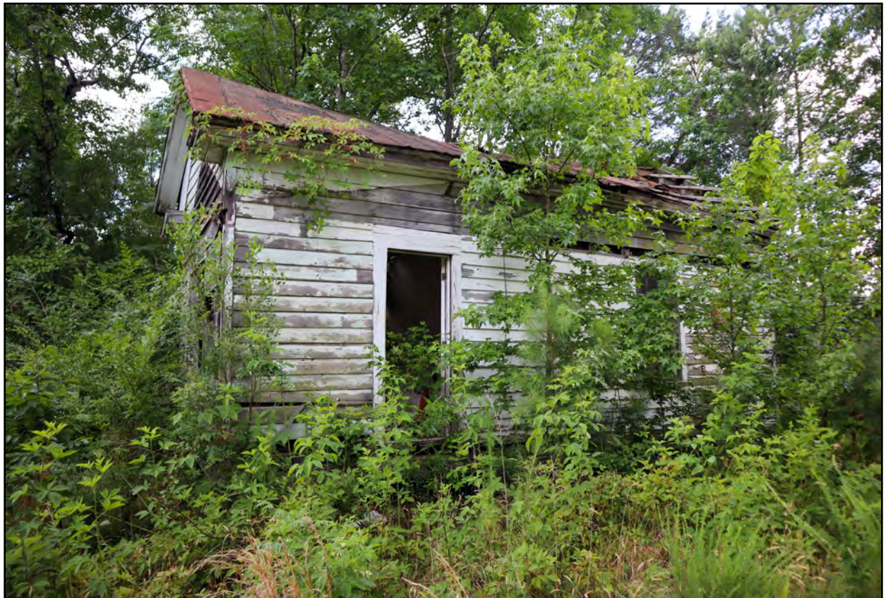
Figure 4.41: View of the primary (north) elevation of the (former) kitchen.
