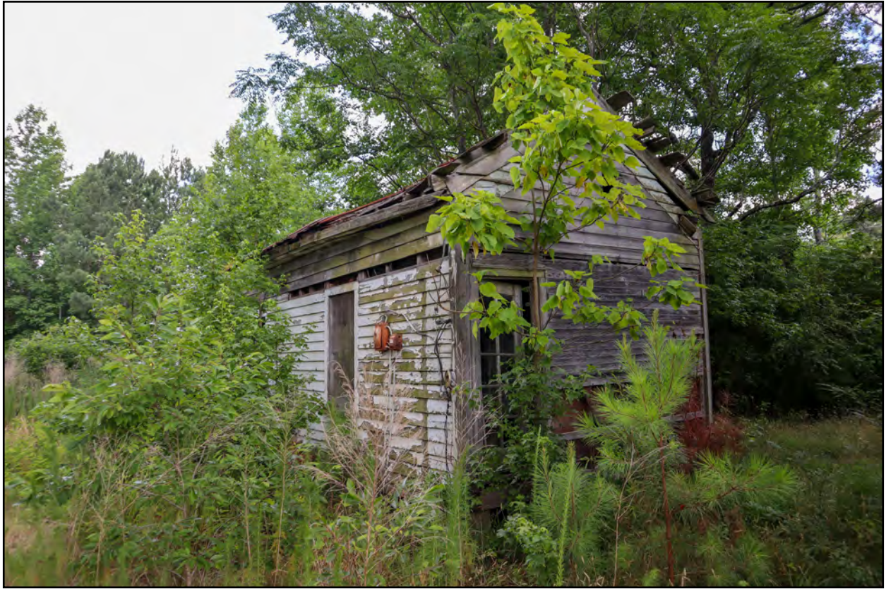
Figure 4.42: View of the primary (north) and west elevations of the (former) kitchen.
