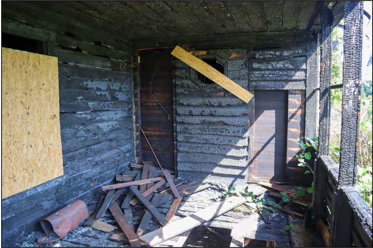
Figure 4.18: Detail view of the front porch on the circa-1810 section of the Hunter-Prince House looking north.
