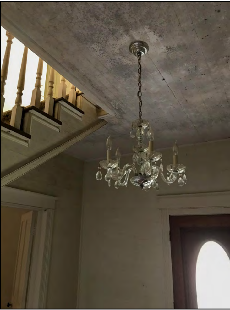
Figure 4.30: Interior view of the front entry of the I-house prior to the fire (Courtesy of Jeremy Bradham, Capital Area Preservation).
