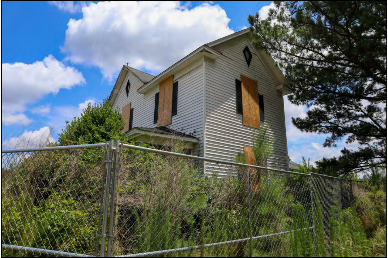
Figure 4.10: View of the west and primary (north) elevations of the Hunter-Prince House.
