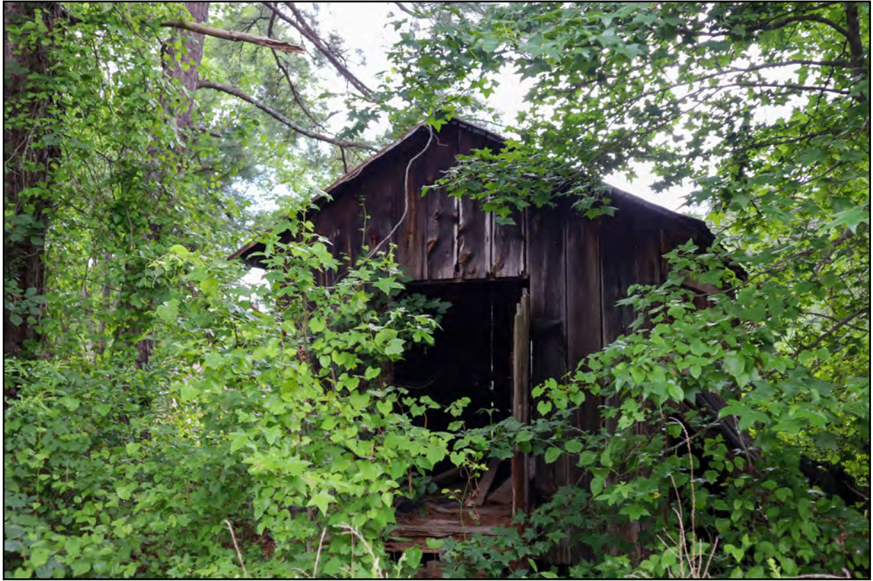
Figure 4.44: View of the primary (south) elevation of the shed.
