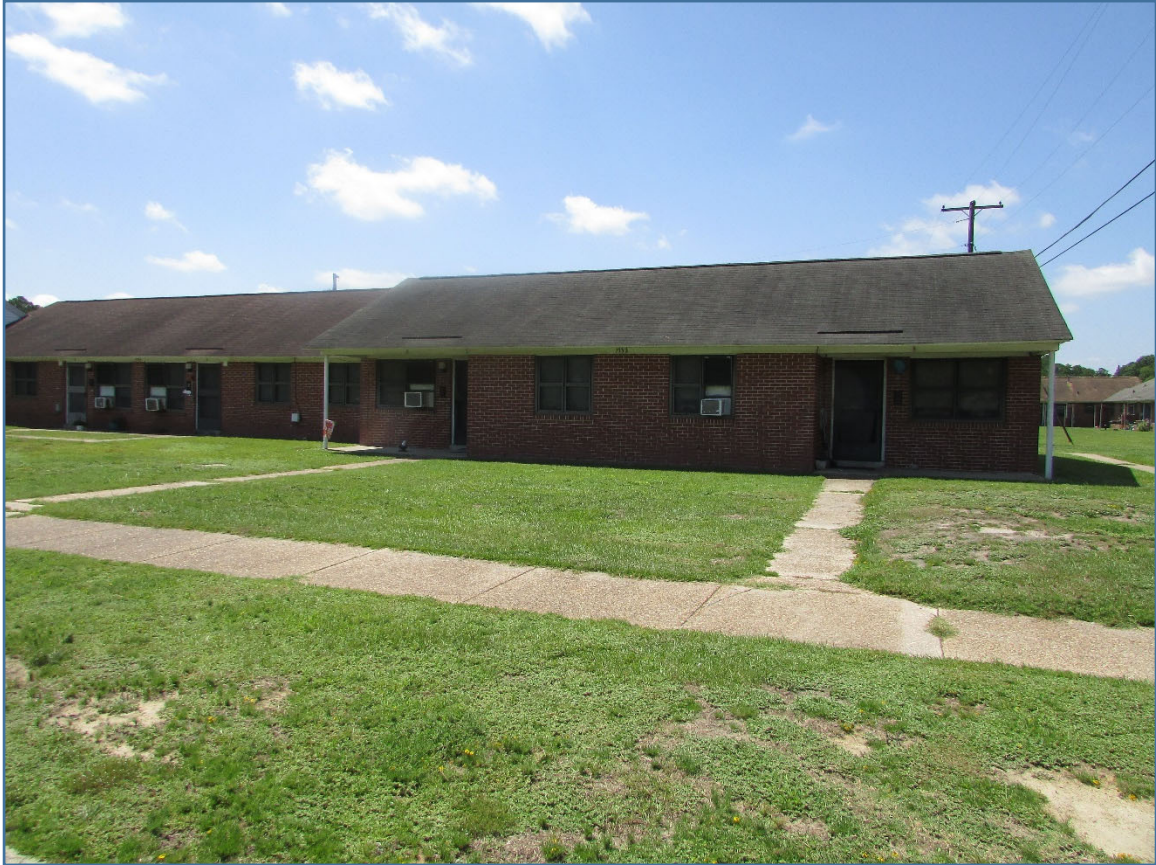
Figure 11. Fairview Apartment, 1721 Edgerton Street facade, view to the south.
