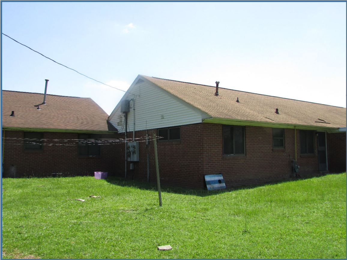
Figure 7. Fairview Apartments, 905 Fairview Circle, building B, rear elevation, view to the east.
