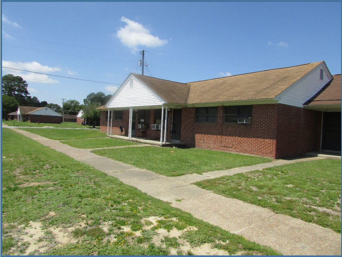
Figure 17. Fairview Apartments, 1728 Edgerton Street, view to the southwest.
