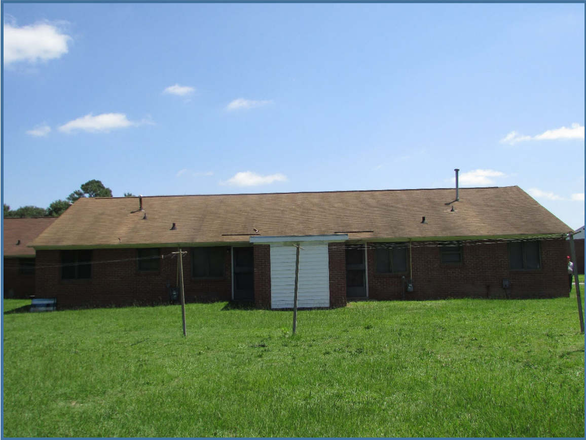
Figure 6. Fairview Apartments, 905 Fairview Circle, building B, rear elevation, view to the east.
