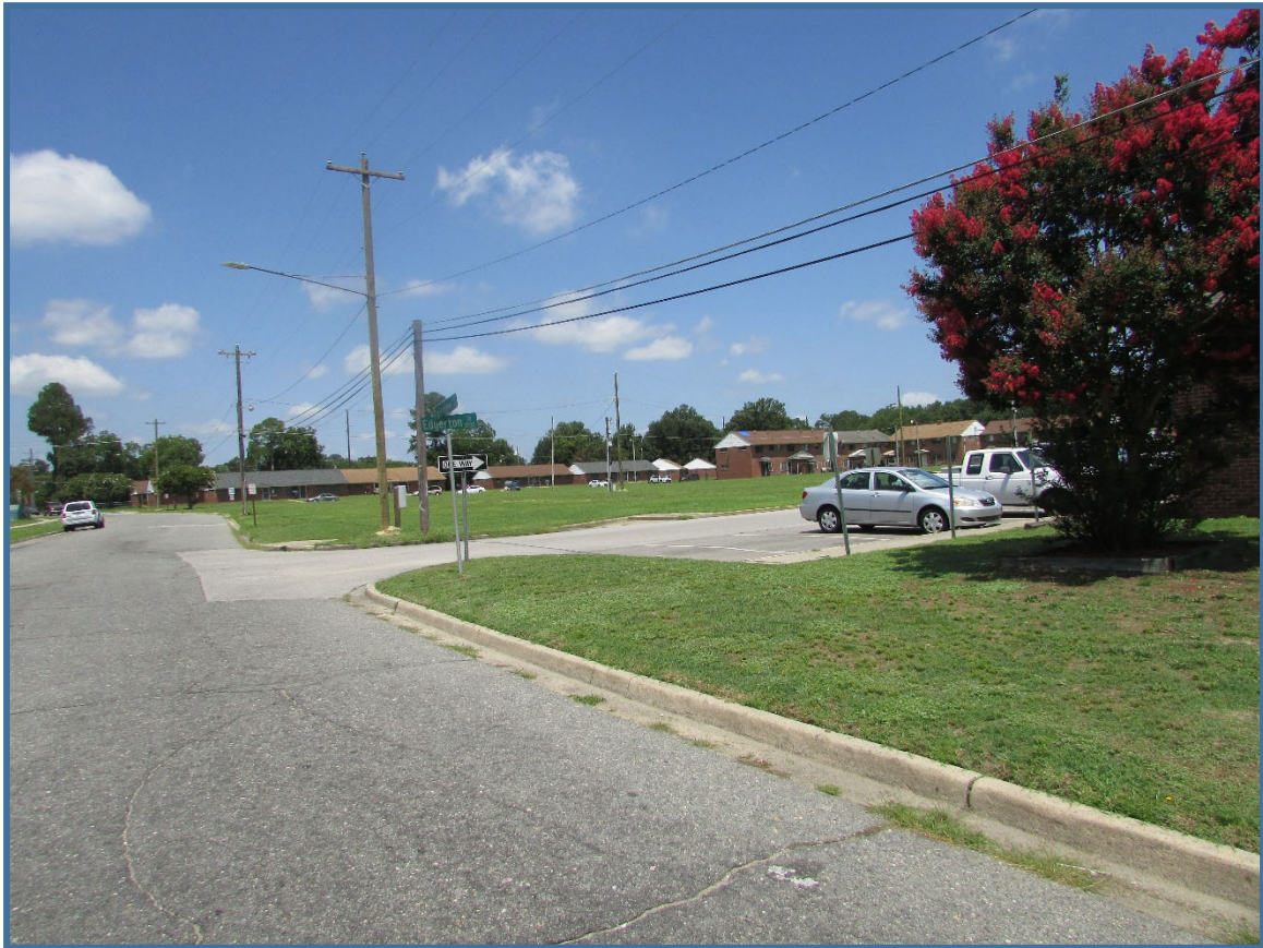
Figure 24. Fairview Apartments, intersection of Edgerton Street and Fairview Circle, view to the northwest.
