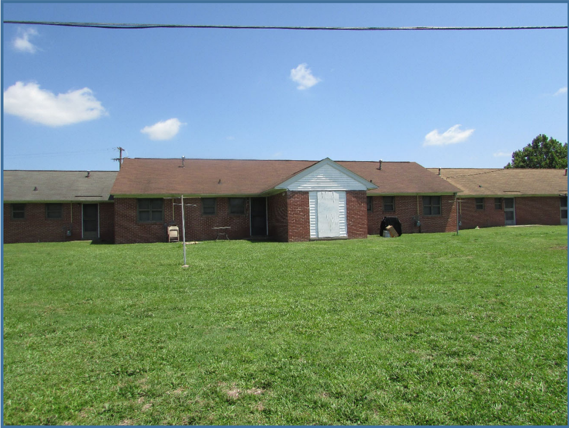
Figure 13. Fairview Apartments, 1726 Edgerton Street, rear elevation, view to the north.
