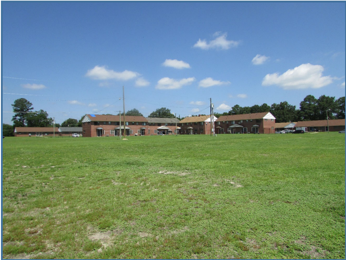
Figure 4. Fairview Apartments, buildings slated for demolition, view to the northwest.
