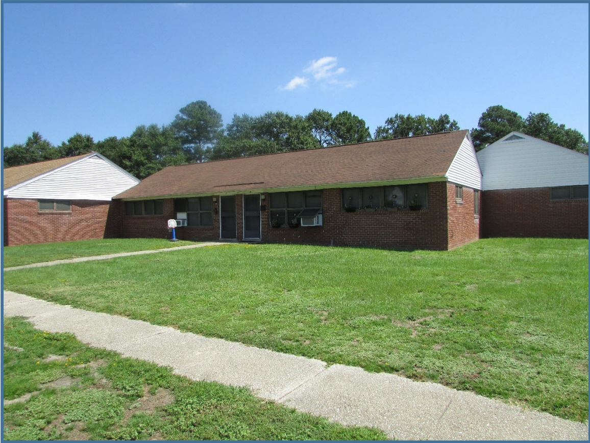
Figure 8. Fairview Apartments, 937 Fairview Circle, building B, view to the northeast.
