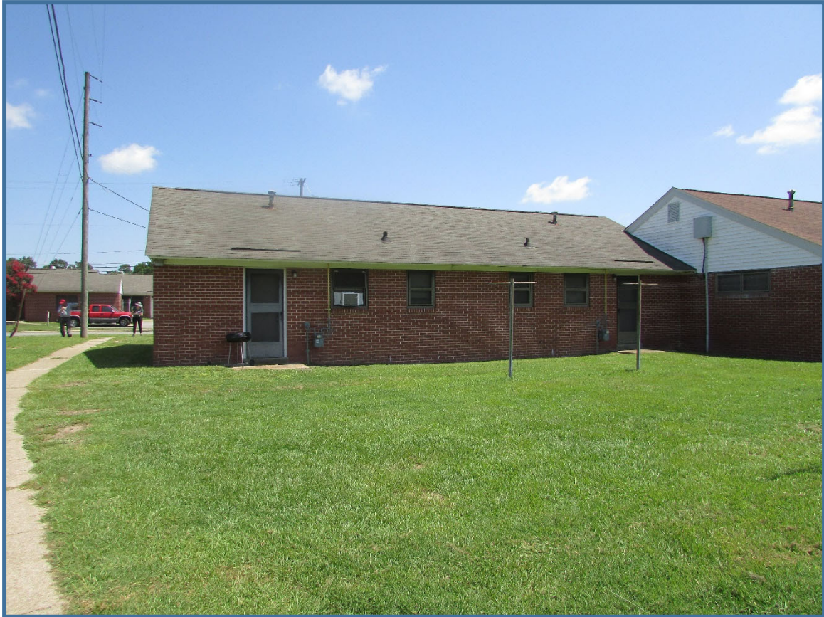
Figure 12. Fairview Apartments, 1724 Edgerton Street, rear elevation, view to the north.
