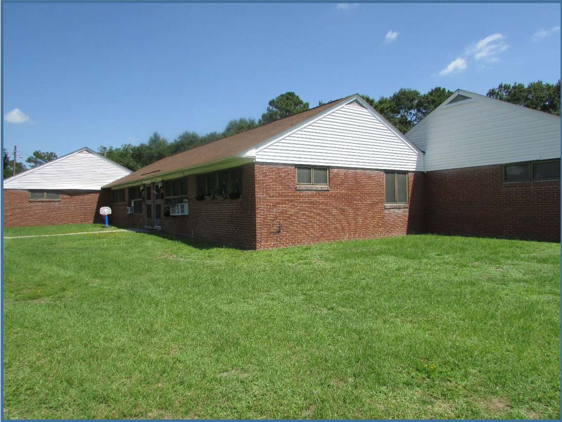
Figure 9. Fairview Apartment, 937 Fairview Circle, building B, view to the northeast.
