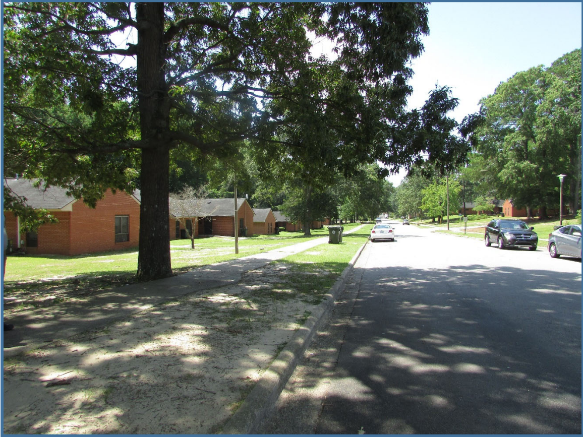
Figure 22. Fairview Apartments, North Claiborne Street, view to the south.
