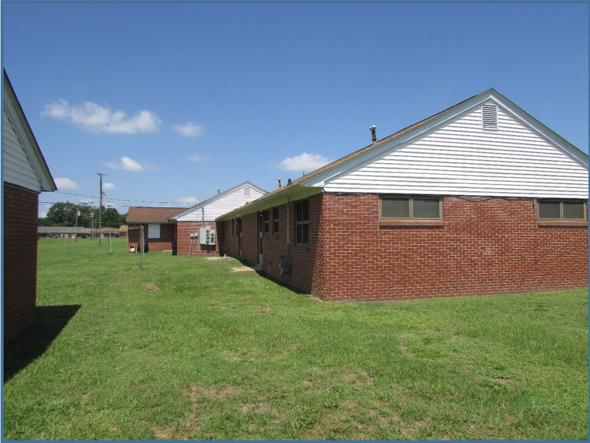
Figure 16. Fairview Apartments, 1728 Edgerton Street, view to the west.
