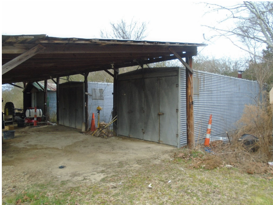
Photograph 19: Three metal sheds at 3033 Watkins Town Road, facing northwest.
