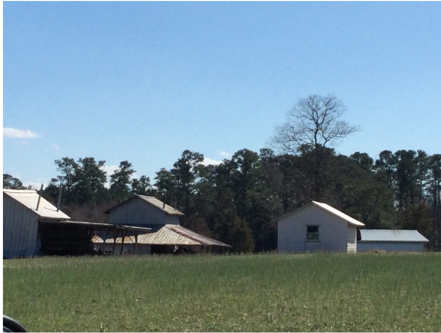
Photograph 70: Agricultural Outbuildings at Charles H Horton Farm (WA1929), facing south.
