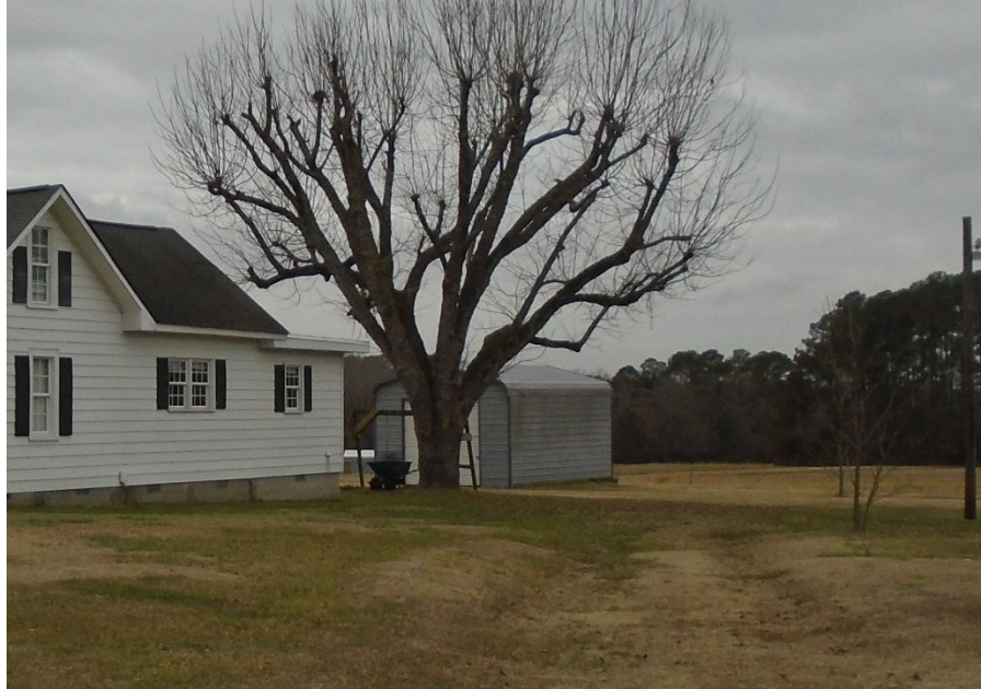
Photograph 11: Quonset hut on property line between 3031 and 3033 Watkins Town Rd, looking southwest.
