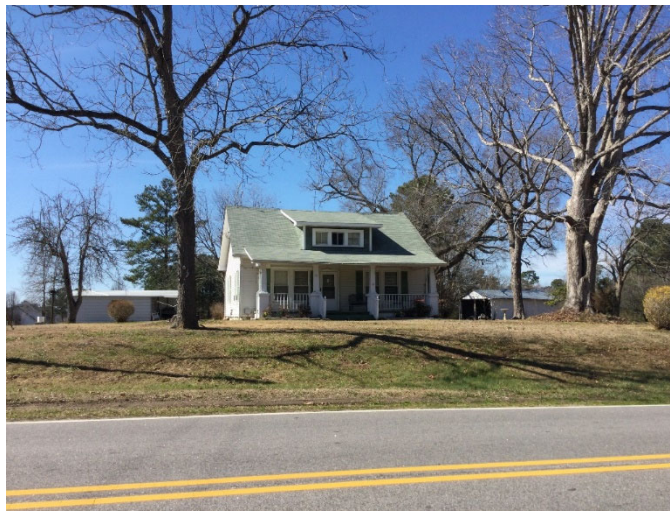
Photograph 31: Otha Massey House (WA1900), 3129 Watkins Town Rd, facing west.
