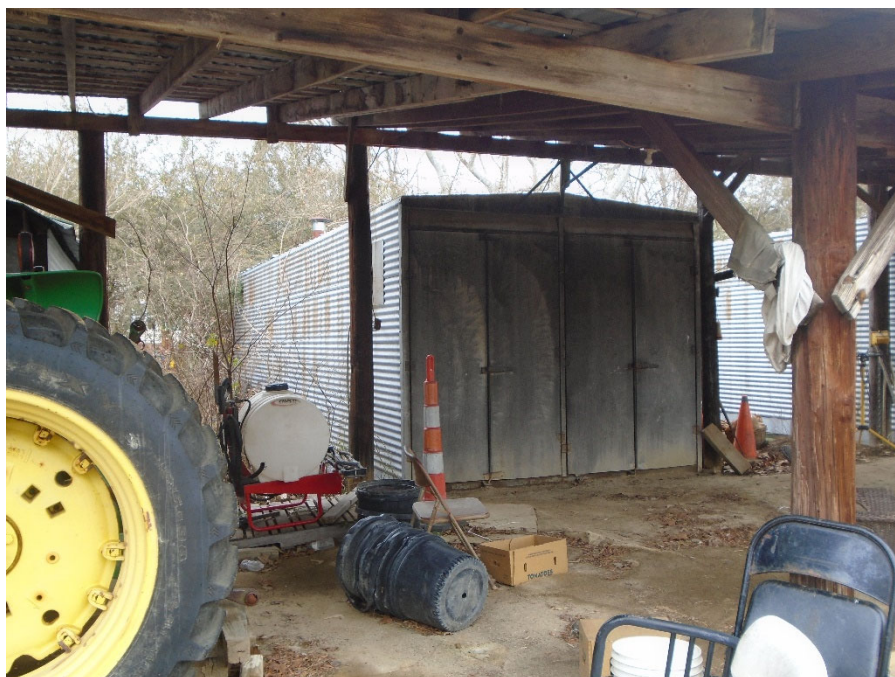
Photograph 17: Metal shed at 3033 Watkins Town Rd, looking north.
