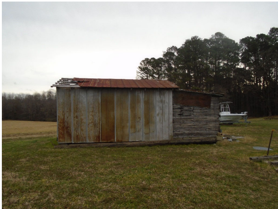
Photograph 55: Shed Barn at Robert Watkins Farm (WA1699), facing east.
