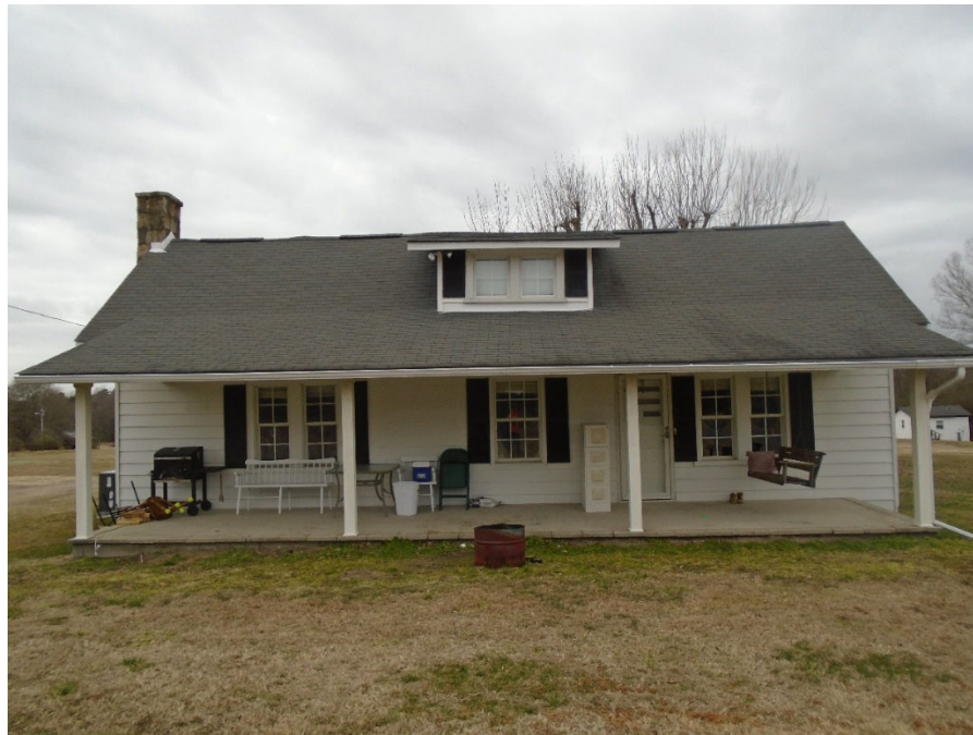
Photograph 2: 3031 Watkins Town Rd, east (main) façade, looking west.
