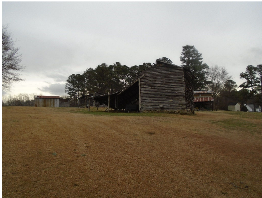
Photograph 53: Overview of Robert Watkins Farm Outbuildings (WA1699) from Watkins Town Road, facing southeast.
