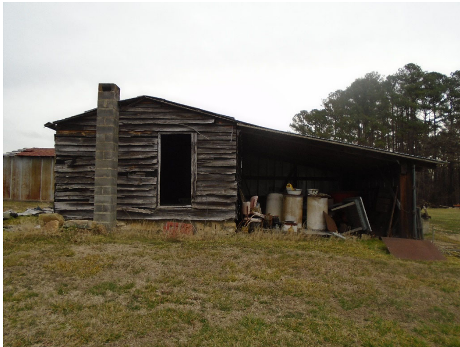
Photograph 58: Strip Room at Robert Watkins Farm (WA1699), facing east.
