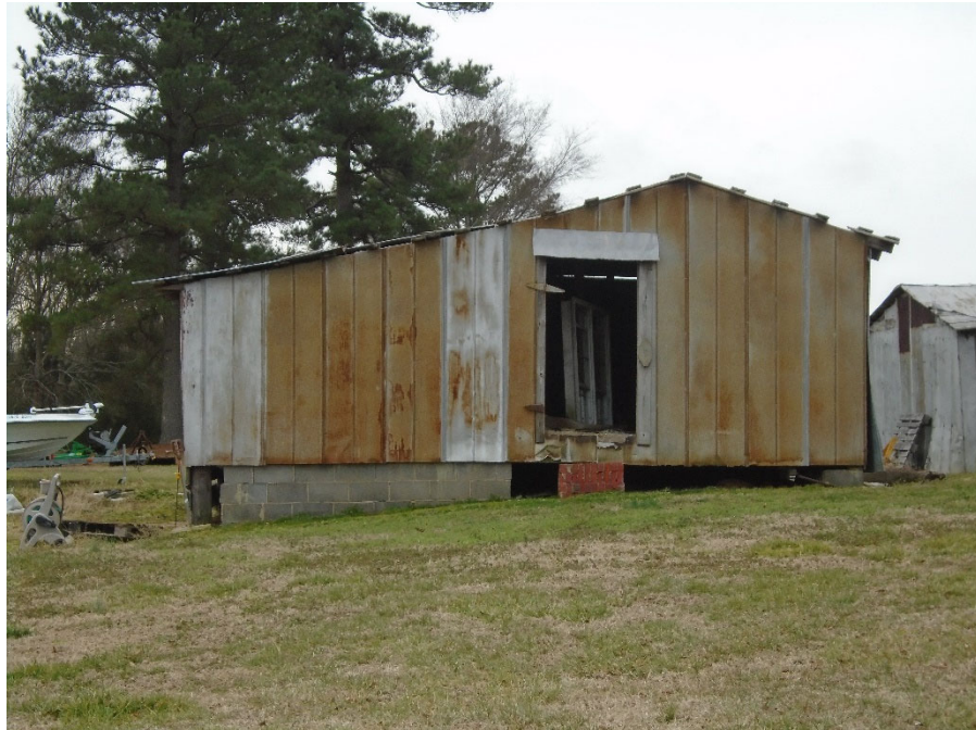
Photograph 54: Shed Barn at Robert Watkins Farm (WA1699), facing south.
