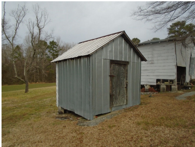
Photograph 40: Metal Shed at the Willard E. and Joyce Watkins Duke House, facing north.
