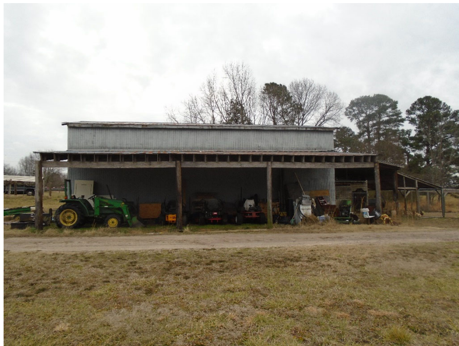
Photograph 27: Side of Barn at 3029 Watkins Town Rd, facing southeast.
