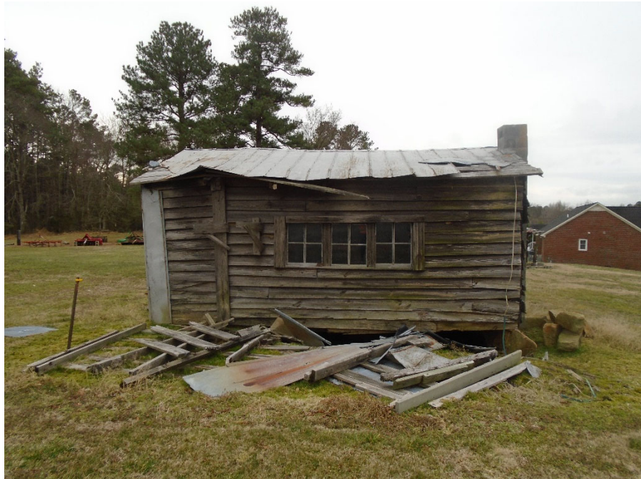
Photograph 59: Strip Room at Robert Watkins Farm (WA1699), facing south.
