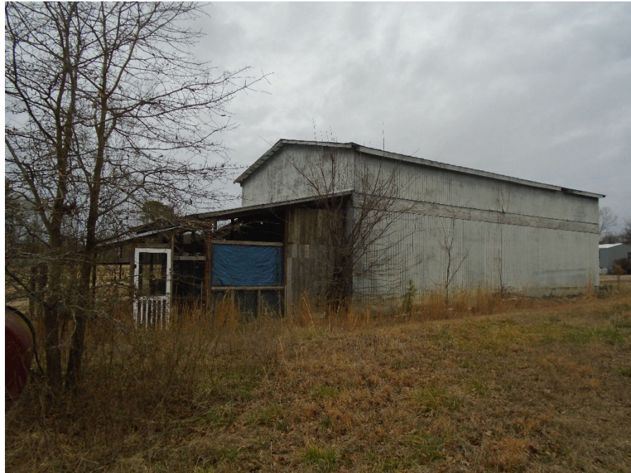
Photograph 28: Rear elevation of Barn at 3029 Watkins Town Rd, facing north.
