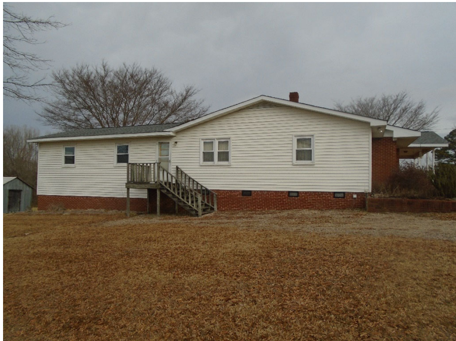
Photograph 36: The Willard E. and Joyce Watkins Duke House, south elevation, facing north.
