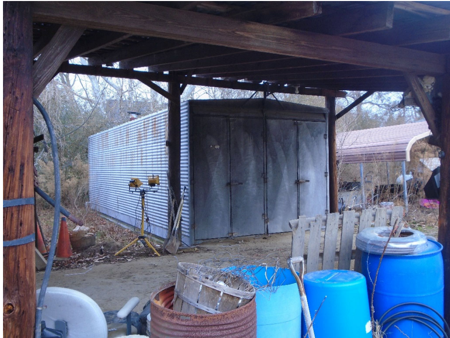
Photograph 18: Metal shed at 3033 Watkins Town Rd, looking north.
