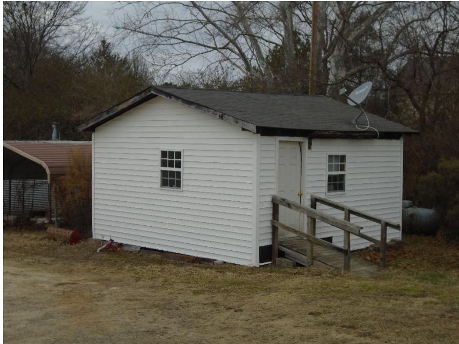
Photograph 15: Small shed at 3033 Watkins Town Rd, looking northwest.
