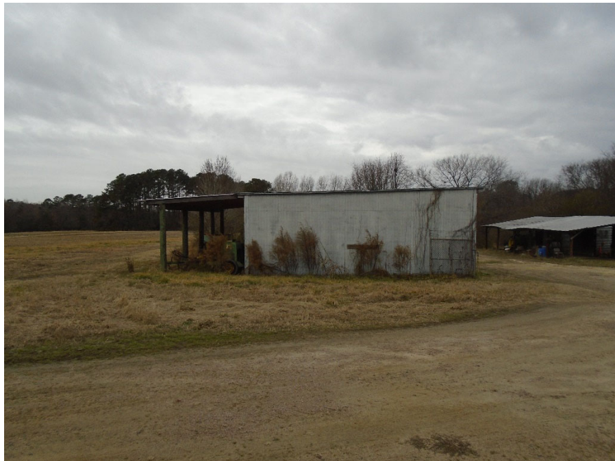
Photograph 13: Tractor Garage, east elevation, looking west.
