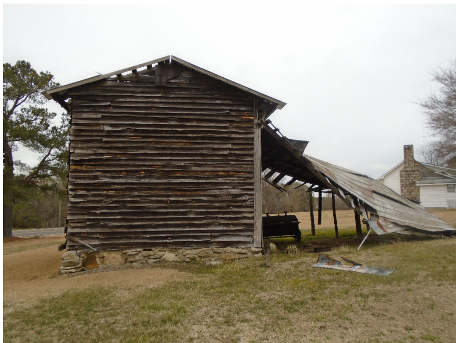
Photograph 63: Two-story barn at Robert Watkins Farm (WA1699), facing west.
