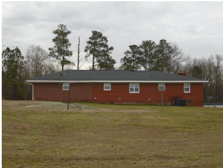
Photograph 9: 3033 Watkins Town Rd, northwest elevation, looking southeast.
