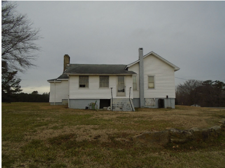
Photograph 51: Main house at Robert Watkins Farm (WA1699), east elevation, facing west.
