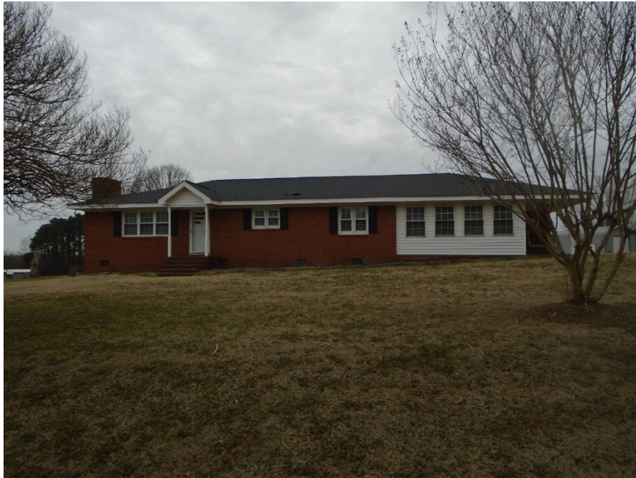
Photograph 7: 3033 Watkins Town Rd, main southeast façade, looking northwest.
