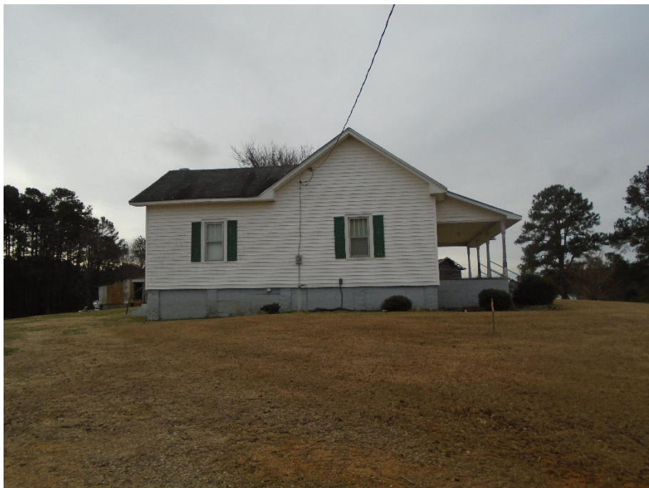
Photograph 52: Main house at Robert Watkins Farm (WA1699), north elevation, facing south.
