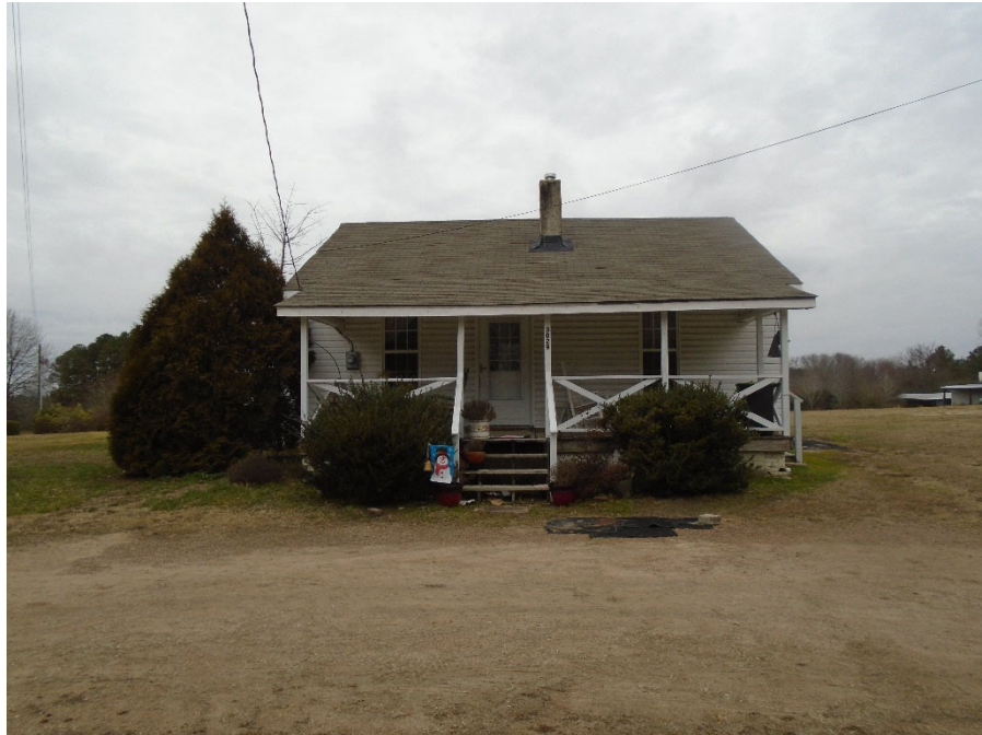
Photograph 21: 3029 Watkins Town Rd, main southeast facade, facing northwest.
