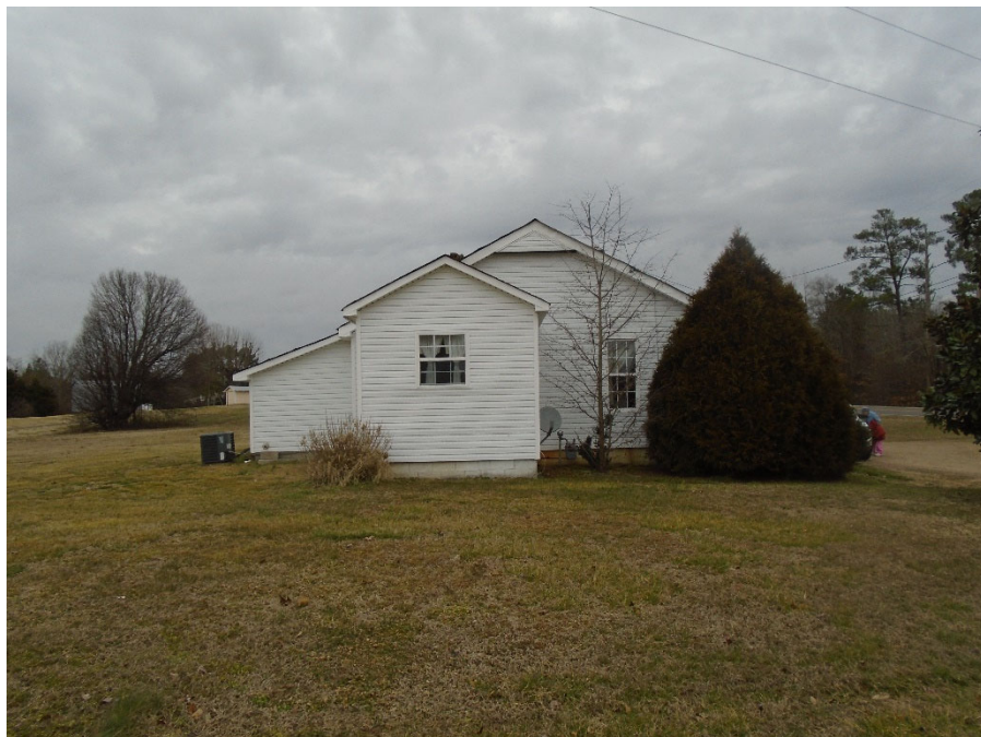
Photograph 24: 3029 Watkins Town Rd, southwest elevation, facing northeast.
