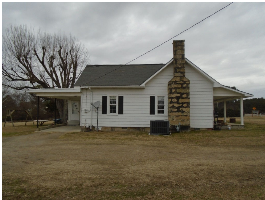
Photograph 3: 3031 Watkins Town Rd, north elevation, looking south.
