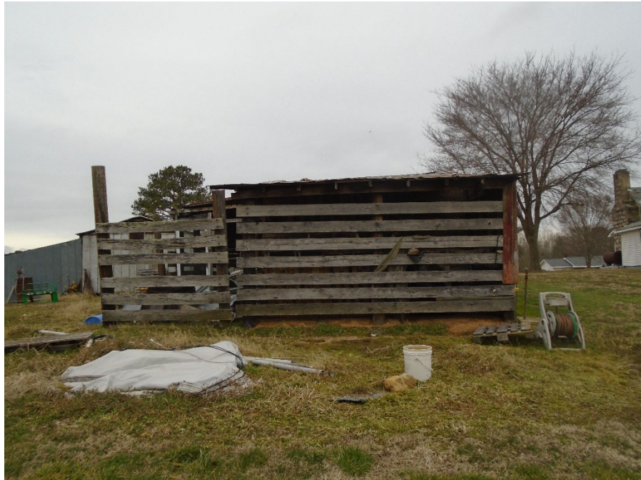
Photograph 56: Shed Barn at Robert Watkins Farm (WA1699), facing north.
