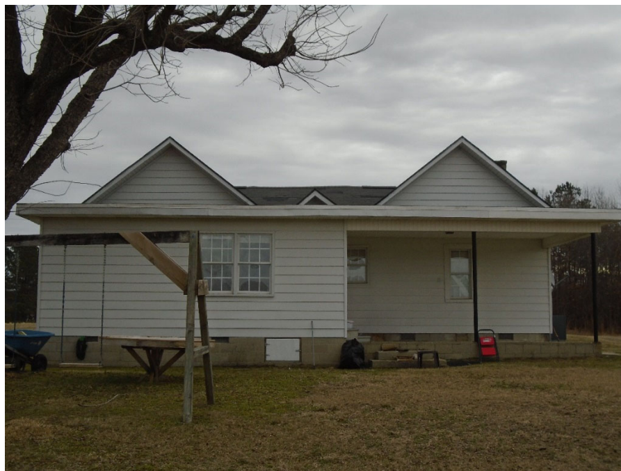
Photograph 4: 3031 Watkins Town Rd, west elevation, looking east.
