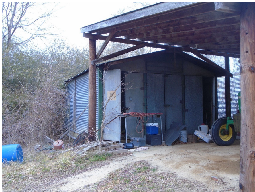
Photograph 16: Metal shed at 3033 Watkins Town Rd, looking north.
