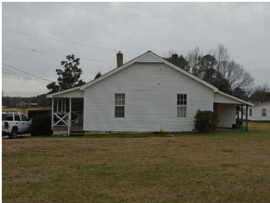
Photograph 22: 3029 Watkins Town Rd, northeast elevation, facing southwest.
