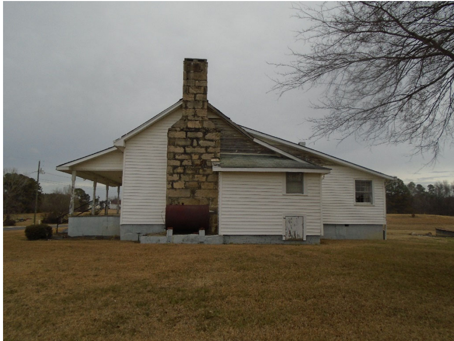
Photograph 50: Main house at Robert Watkins Farm (WA1699), south elevation, facing north.
