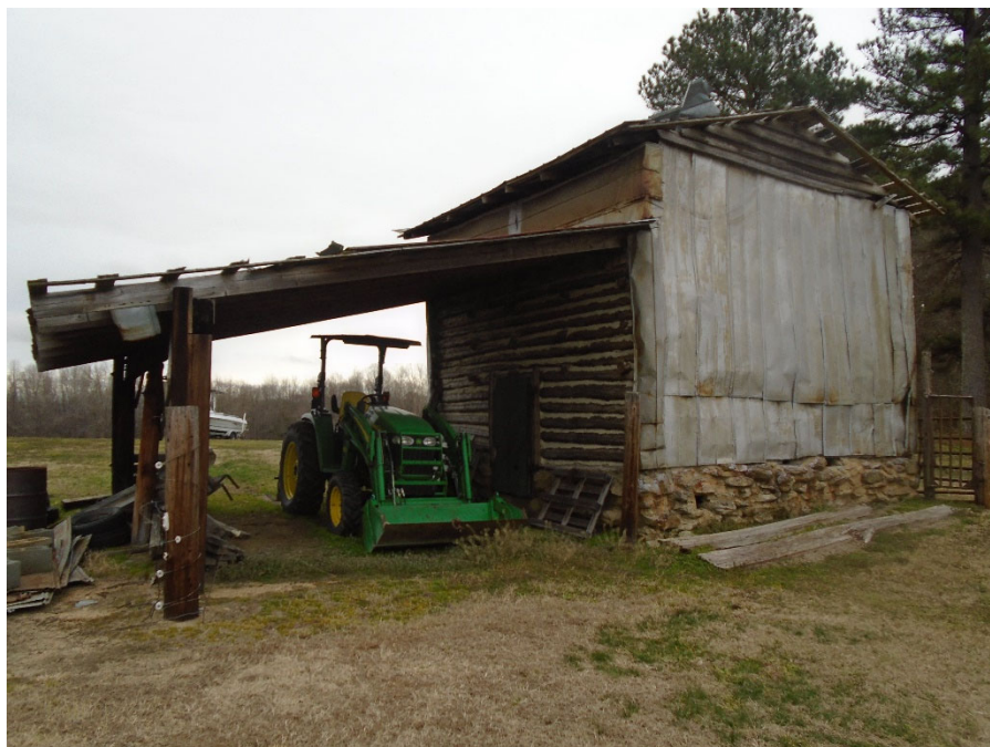
Photograph 67: Log Barn at Robert Watkins Farm (WA1699), facing east.
