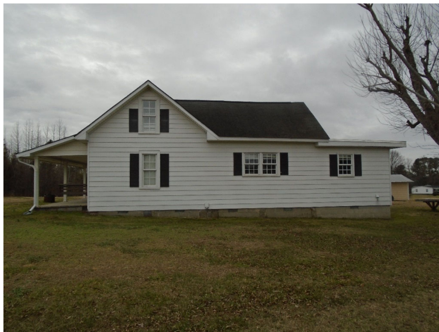
Photograph 5: 3031 Watkins Town Rd, south elevation, looking north.
