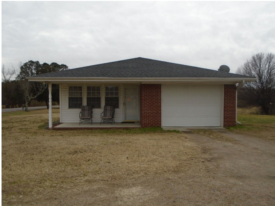
Photograph 8: 3033 Watkins Town Rd, northeast elevation, looking southwest.
