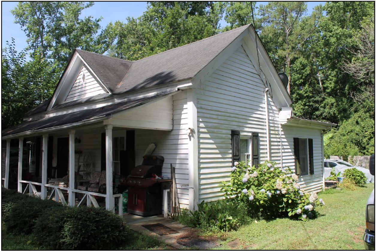
Figure 5.3: WA8801, oblique view of northeast and southeast elevations, facing southwest.
