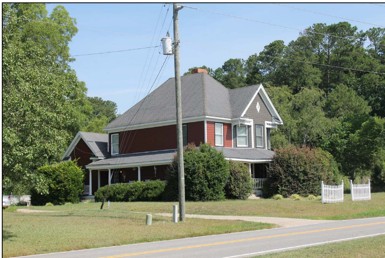
Figure 4.3: Chamblee House, oblique view of southwest and southeast elevations, facing northwest.
