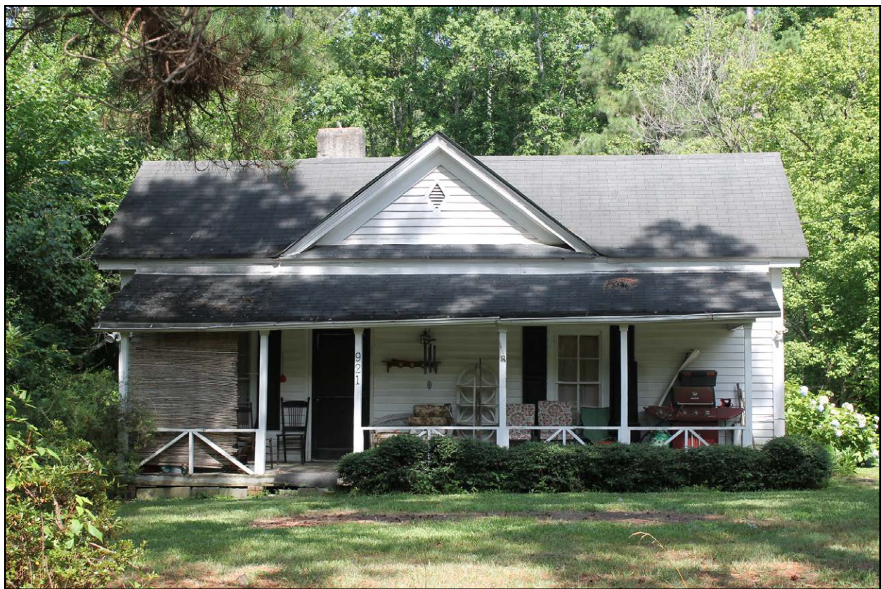
Figure 5.2: WA8801, view of southeast elevation (façade), facing northwest.
