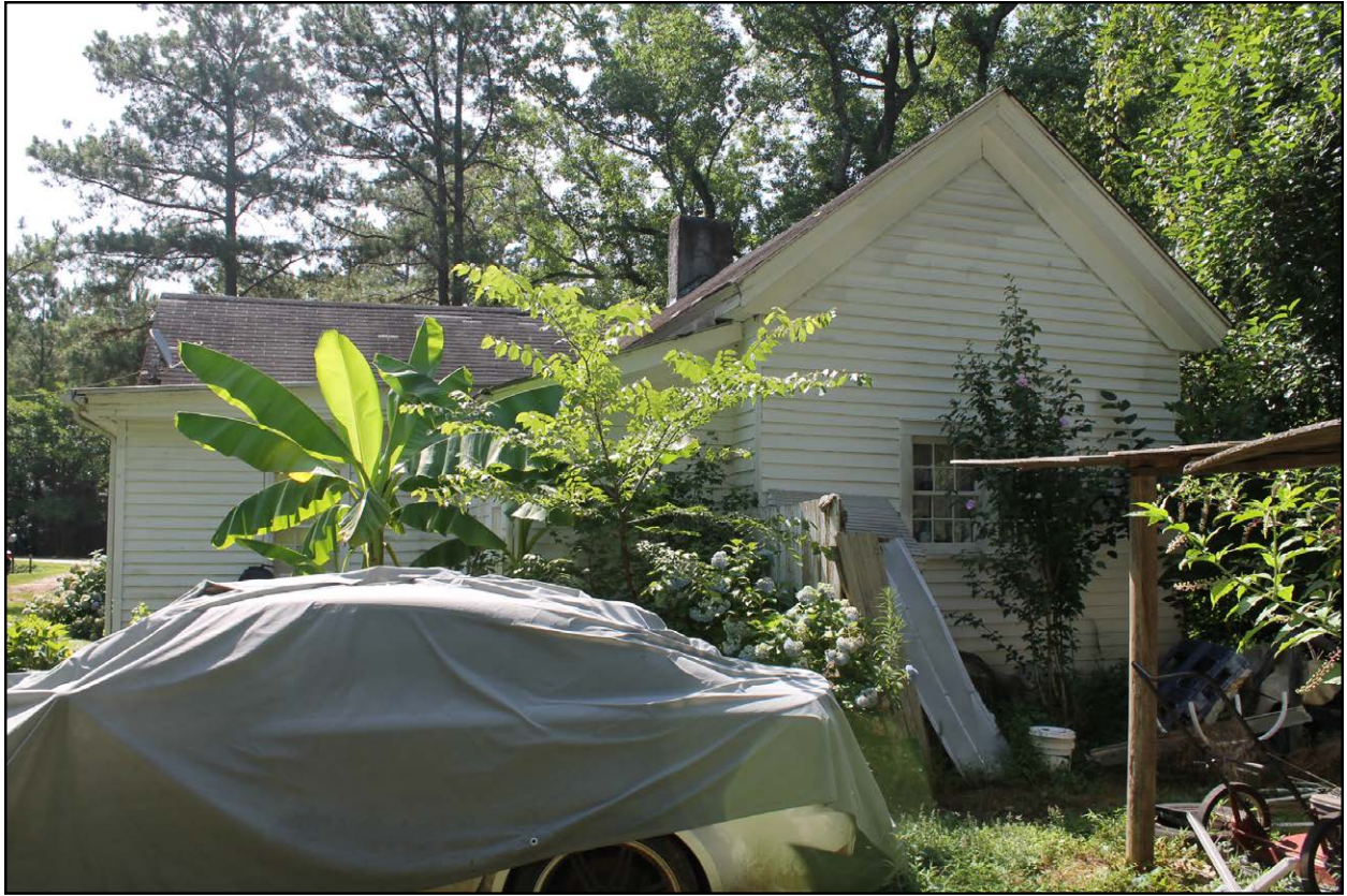
Figure 5.9: WA8801, view of northwest (rear) elevation, facing southeast.
