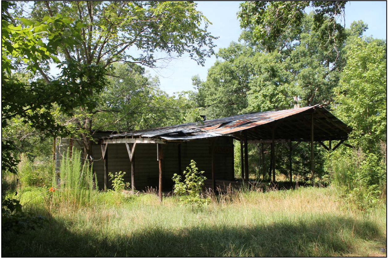
Figure 4.11: Bulk tobacco barn shed, view facing northwest.
