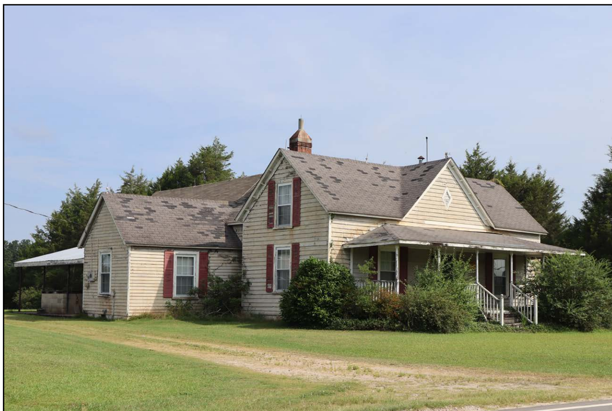
Figure 5.19: Pace Farm house (WA2080)
