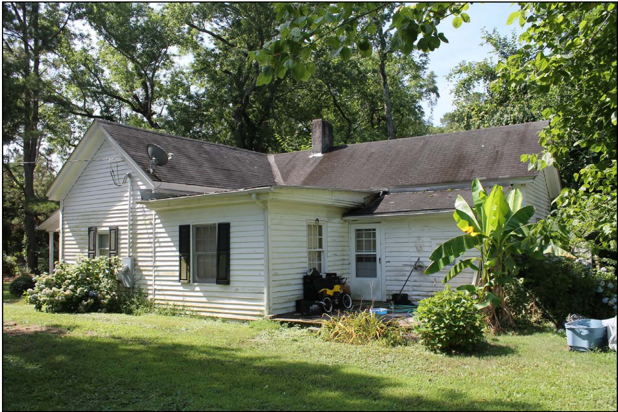
Figure 5.7: WA8801, view of northeast side elevation, facing southeast.
