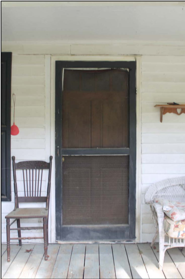
Figure 5.5: WA8801, view of principal entry, facing northwest.
