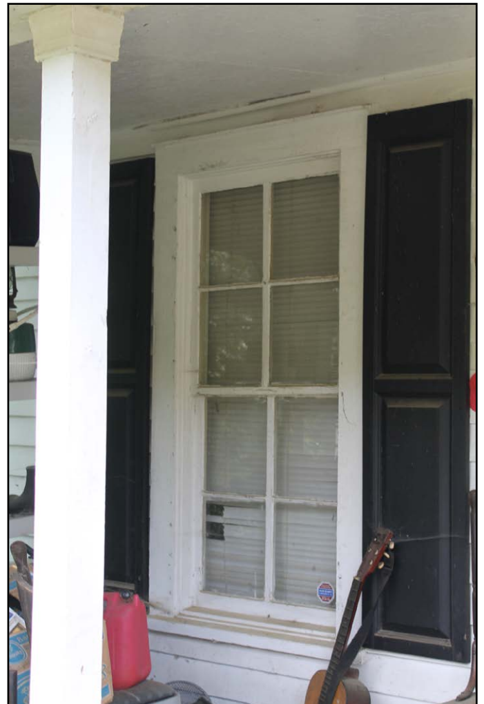
Figure 5.6: WA8801, view of typical original window.
