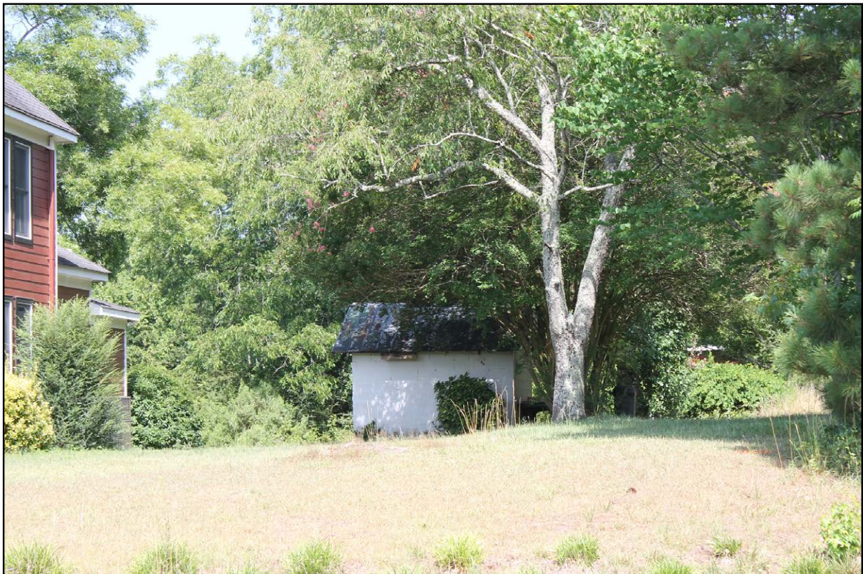
Figure 4.8: Outbuilding, view of southeast side elevation, facing northwest.
