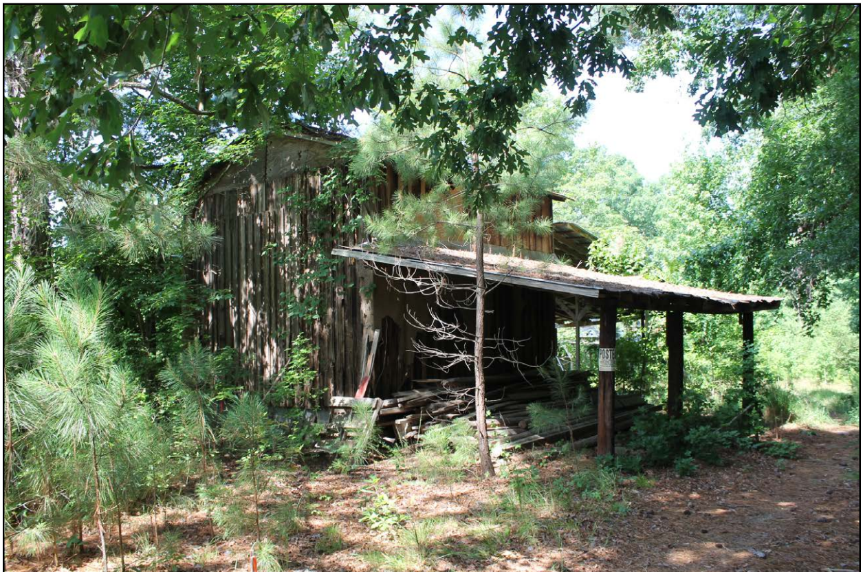
Figure 4.10: Tobacco barn, view of north and east elevations, facing southwest.
