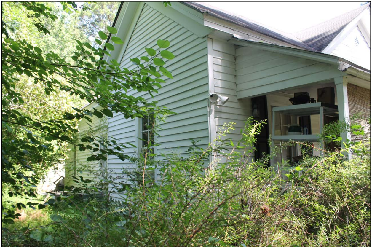
Figure 5.4: WA8801, oblique view of southwest side elevation, facing north.
