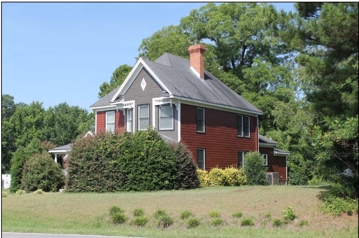
Figure 4.5: Chamblee House, oblique view of northeast and southeast elevations, facing southwest.
