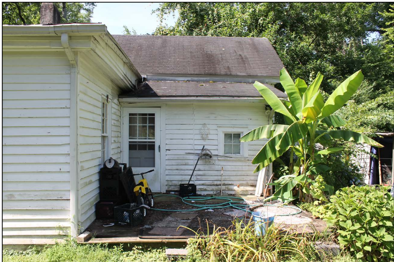
Figure 5.8: WA8801, view of rear additions, facing southwest.
