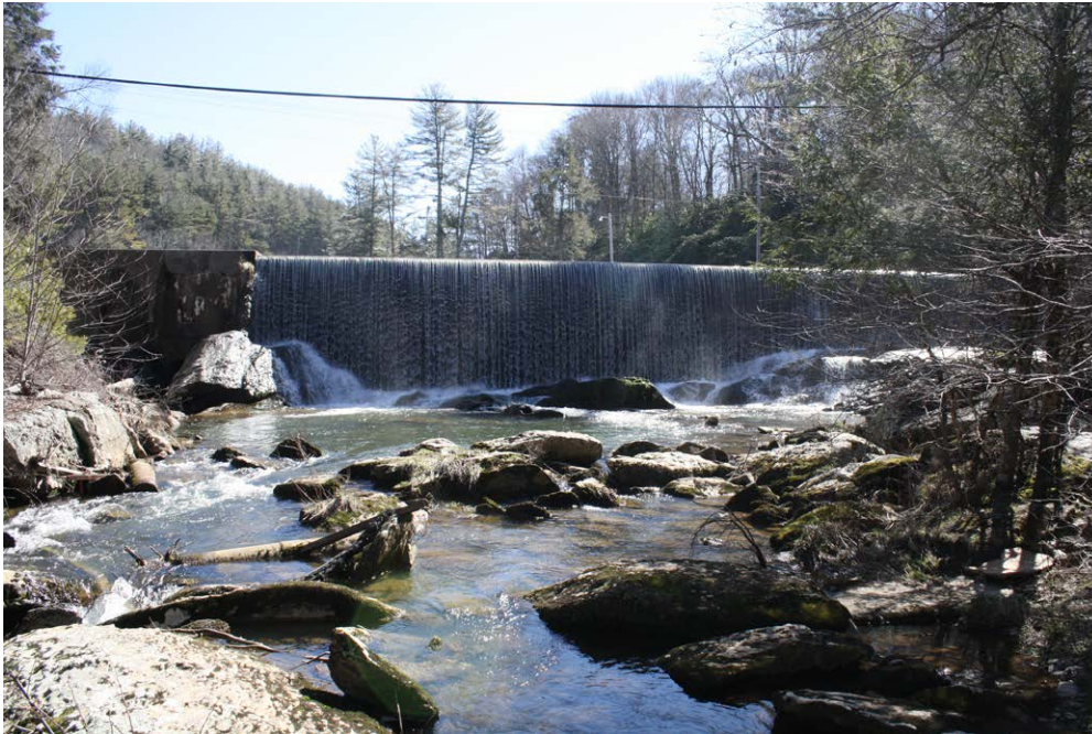
Plate 6.1: Upstream side of the Mill Pond and Dam (AV0252) at Lees-McRae College.
