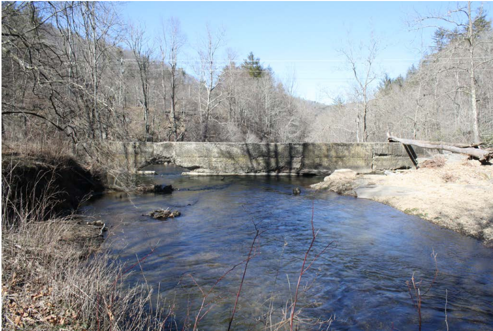
Plate 13.1: View downstream of Shull's Mill Dam (WT0955).
