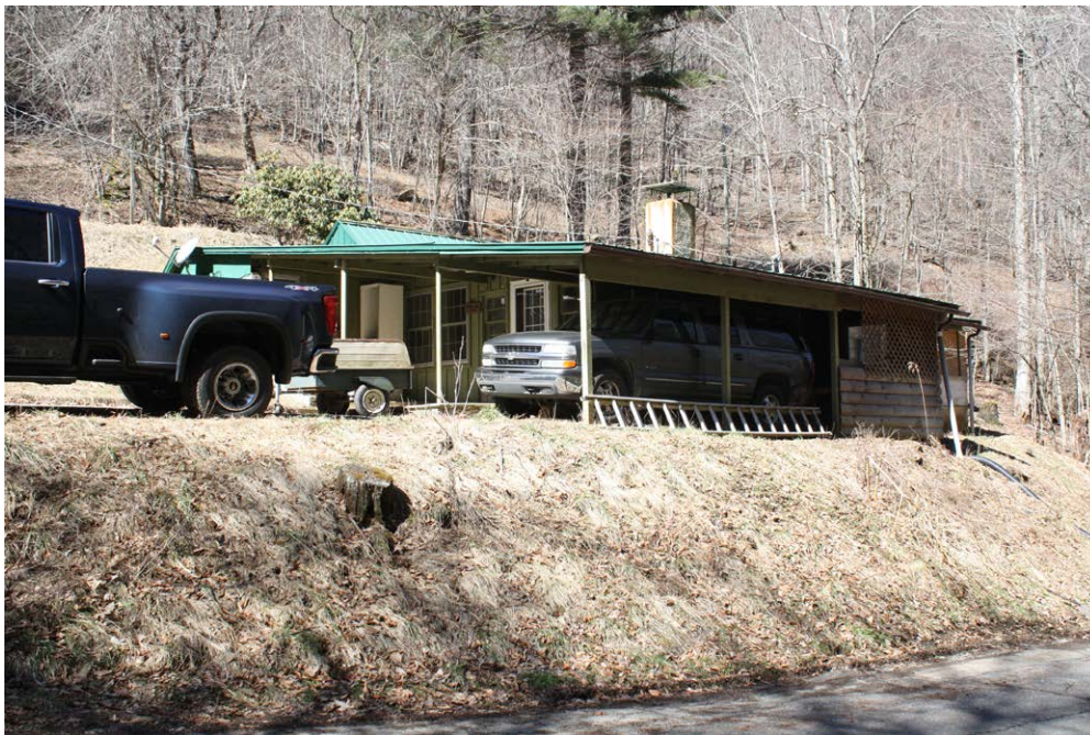
Plate 12.14: Southeast corner of the dwelling on the west side of Trivett Branch.
