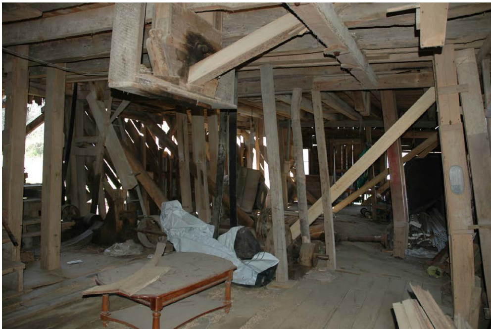
Plate 9.6: Interior view of the west end of the first floor of Winebarger Mill (WT0478).
