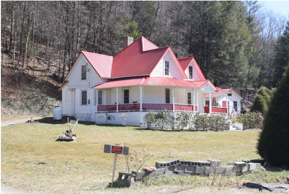
Plate 5.1: Northwest corner of the house situated north of the Knight Pond Dam (AV0215), from Millers Gap Highway.
