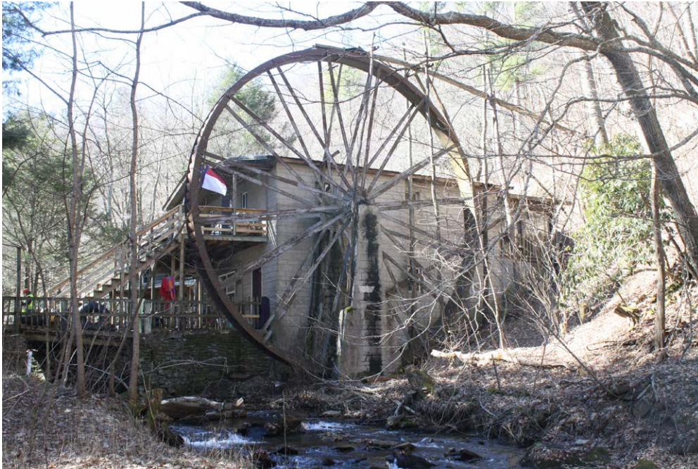
Plate 12.19: North elevation of the mill and machine shop.
