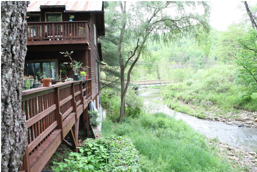
Plate 8.3: West elevation of Sugar Grove Mill (WT0406), showing the site of the former dam.
