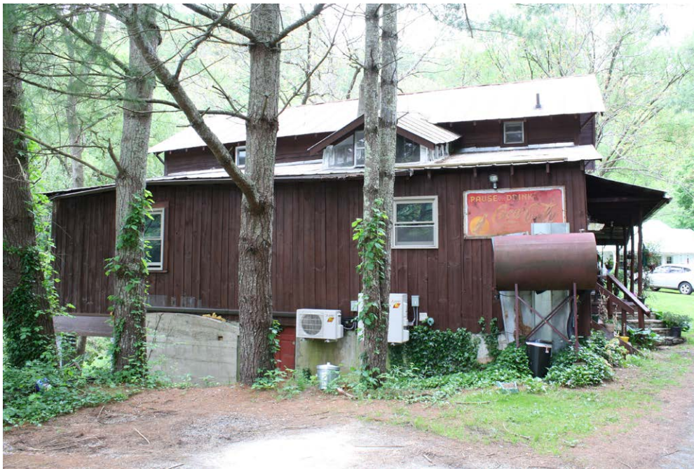
Plate 8.2: South elevation of Sugar Grove Mill (WT0406), from Old Mill Road.
