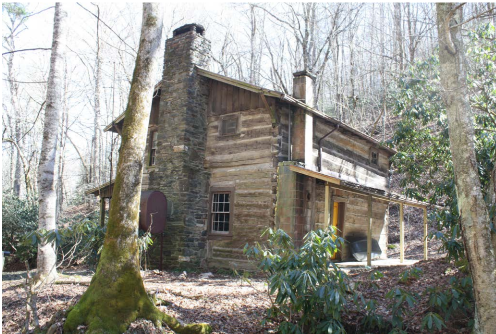
Plate 12.16: West and south elevations of the log house on the east side of Trivett Branch.
