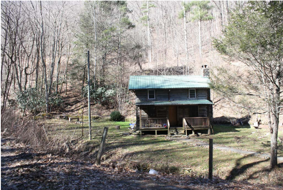
Plate 12.17: East elevation of the log house on the west side of Trivett Branch.
