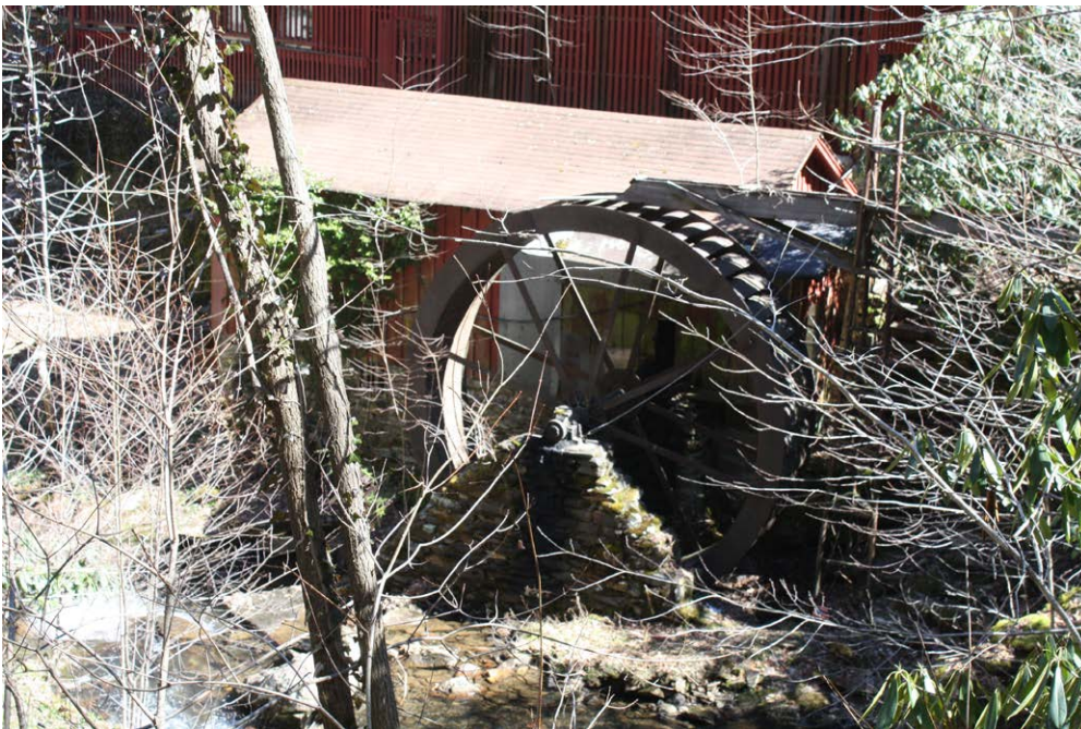
Plate 12.6: Mill building to the west of the 1953 house, viewed from the bridge over Trivett Branch.
