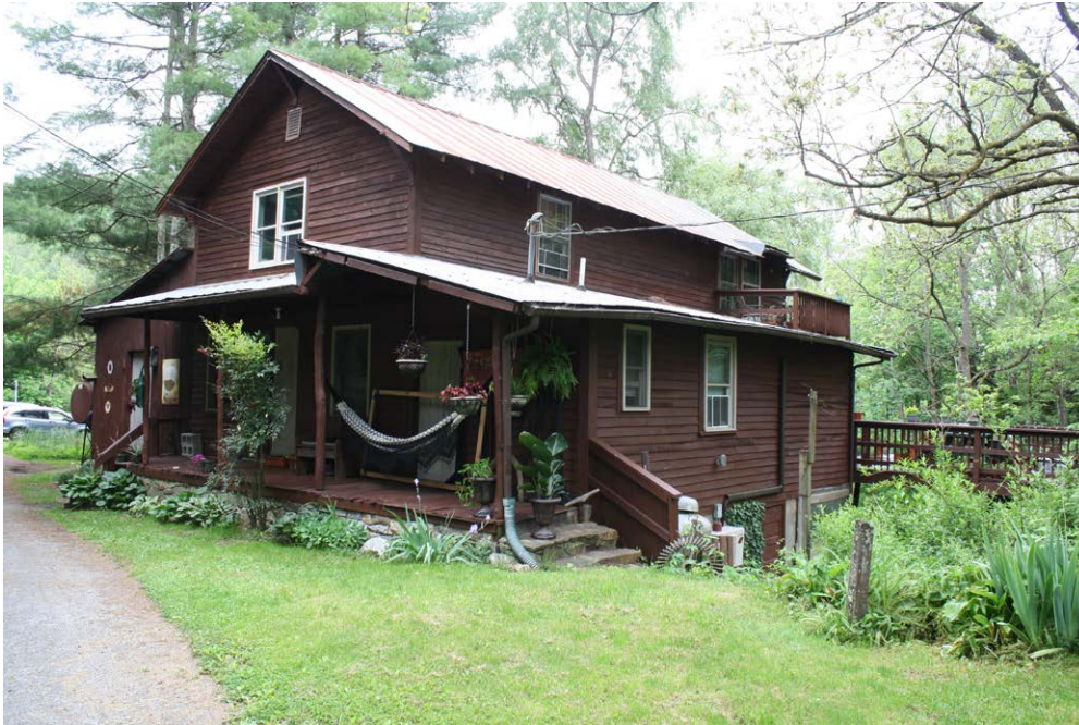
Plate 8.1: North and east elevations of Sugar Grove Mill (WT0406), from Old Mill Road.
