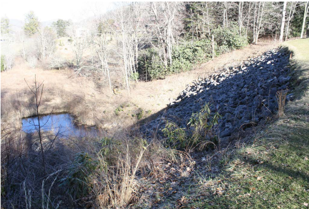
Plate 4.2: Downstream side of the earth-and-riprap Wildcat Lake Dam (AV0214).
