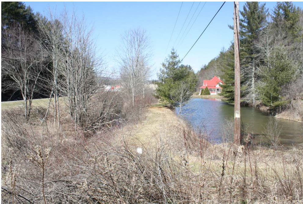
Plate 5.2: Knight Pond Dam (AV0215), showing Millers Gap Highway to the left.
