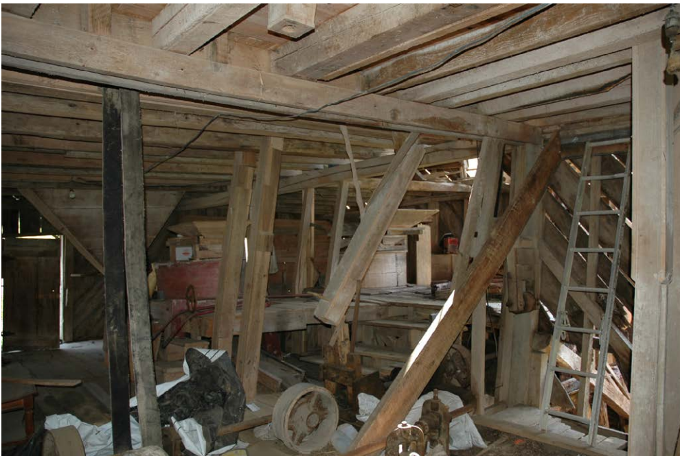
Plate 9.4: Interior view of the east end of the first floor of Winebarger Mill (WT0478).
