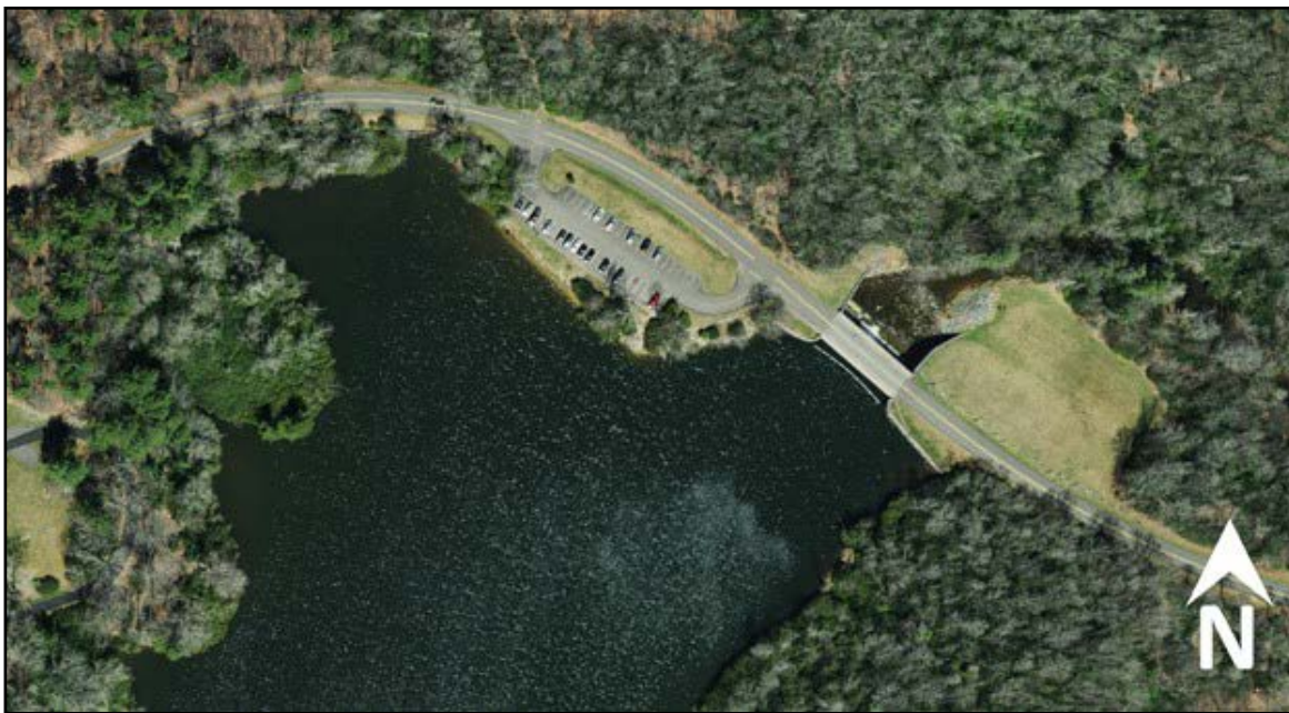
Figure 10.2: Aerial image of Price Lake Dam (WT0734) on the Boone Fork (World Imagery, ESRI 2020).
