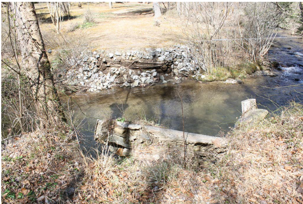
Plate 2.1: Hayes Dam remnant.
