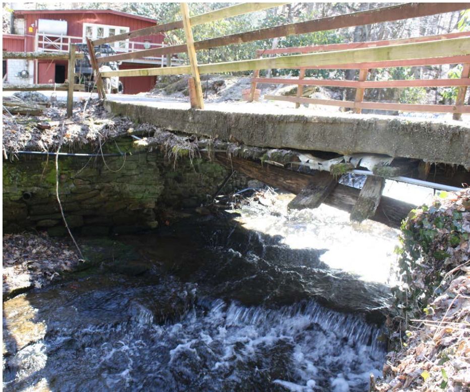
Plate 12.2: Bridge over Trivett Branch on the downstream side of the dam at the Ray Estes Complex (WT0954).
