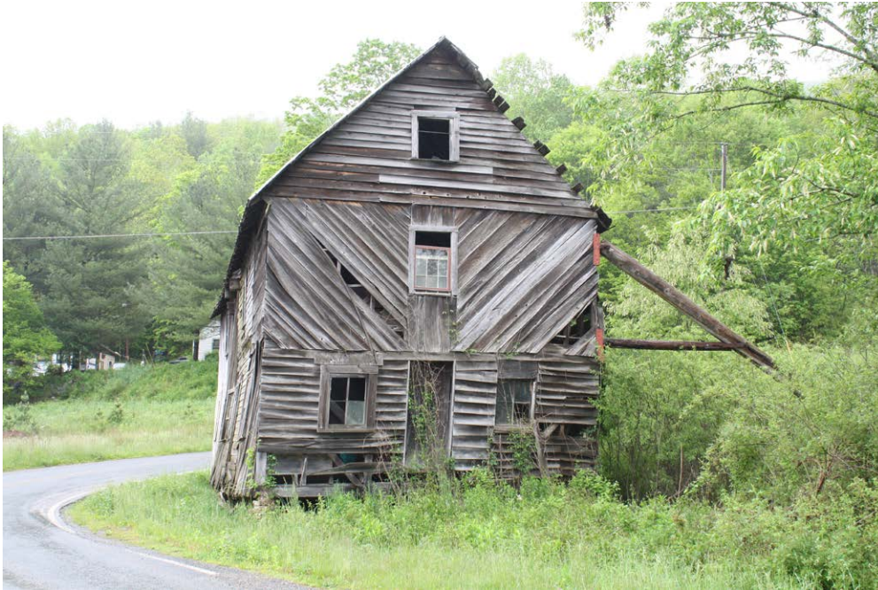
Plate 9.1: West elevation of Winebarger Mill (WT0478), from Hopewell Church Road.
