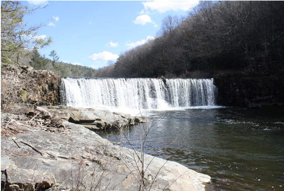
Plate 3.1: View upstream of Sloop's Lake Dam (AV0082) on the Linville River.
