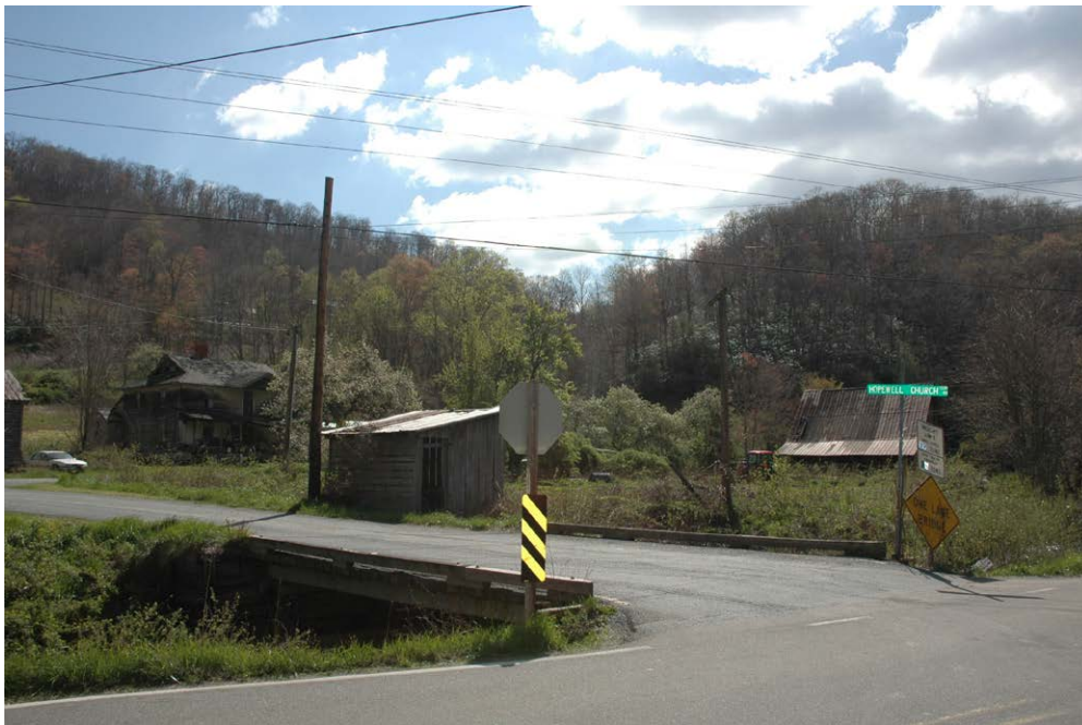
Plate 9.8: Outbuildings historically associated with Winebarger Mill (WT0478), from the intersection of Hopewell Church Road and Meat Camp Road.
