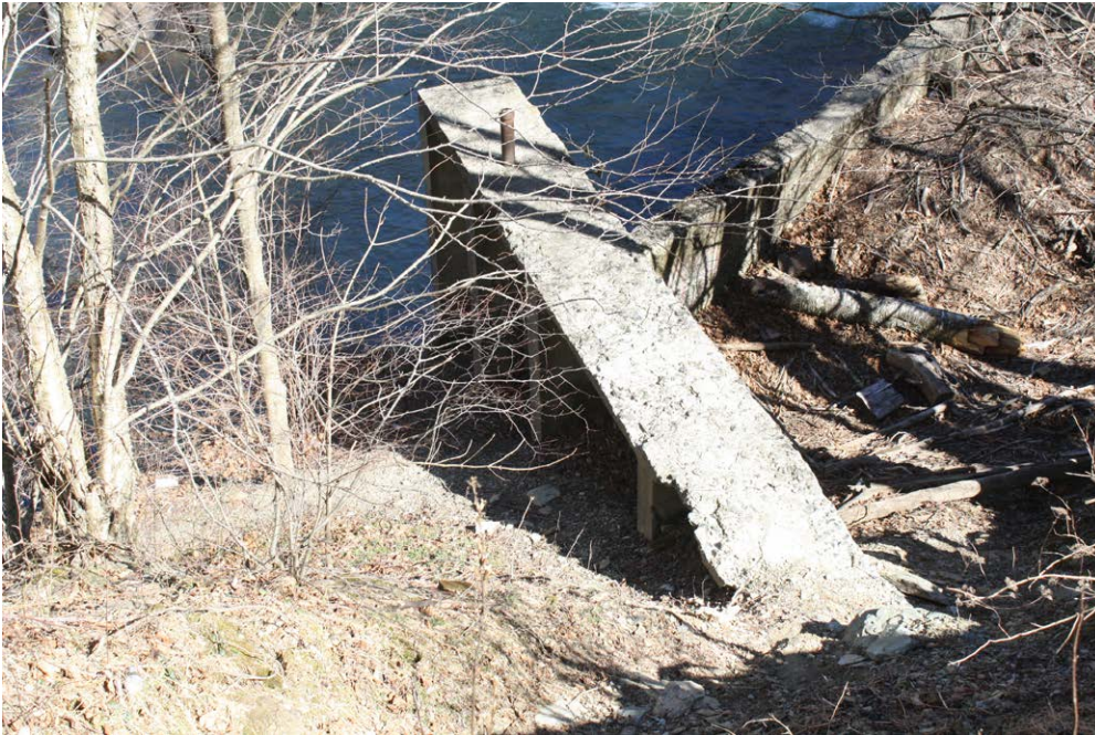
Plate 13.3: Close-up of west abutment at Shull's Mill Dam (WT0955).
