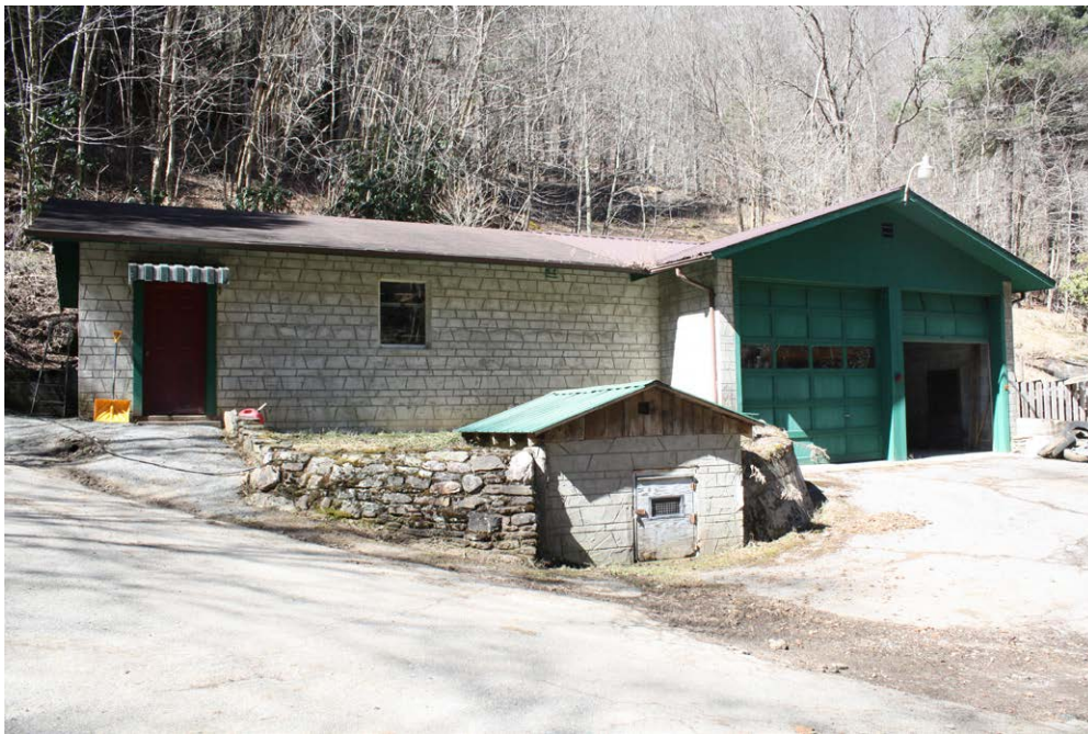
Plate 12.12: Garage/shop and storage building on the west side of Trivett Branch.
