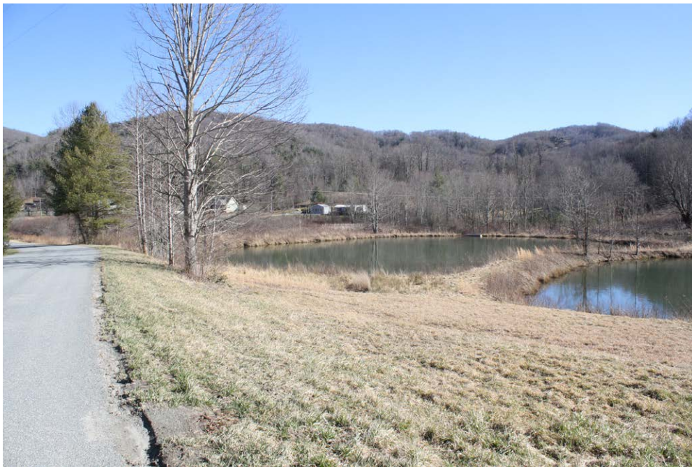
Plate 14.2: Spice Bottom Creek Farm Pond Dam (WT0956), showing Church Hollow Road to the left.
