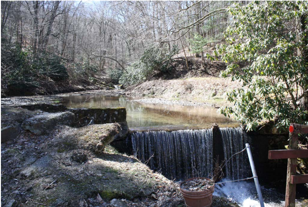
Plate 12.1: Stone dam on Trivett Branch at the southern end of the Ray Estes Complex (WT0954).
