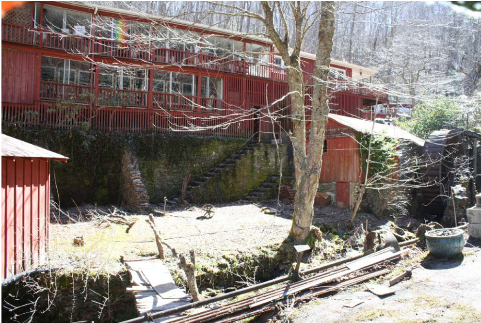
Plate 12.5: West elevation of the 1953 house at the Ray Estes Complex (WT0954).
