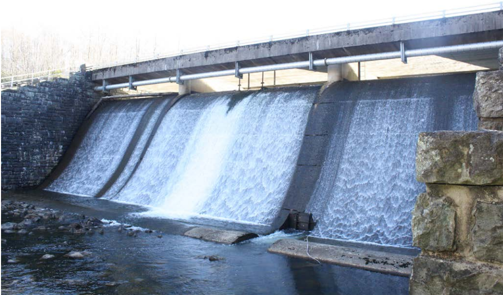
Plate 10.3: Price Lake Dam spillway (WT0734), viewed downslope on the east side of the Blue Ridge Parkway.
