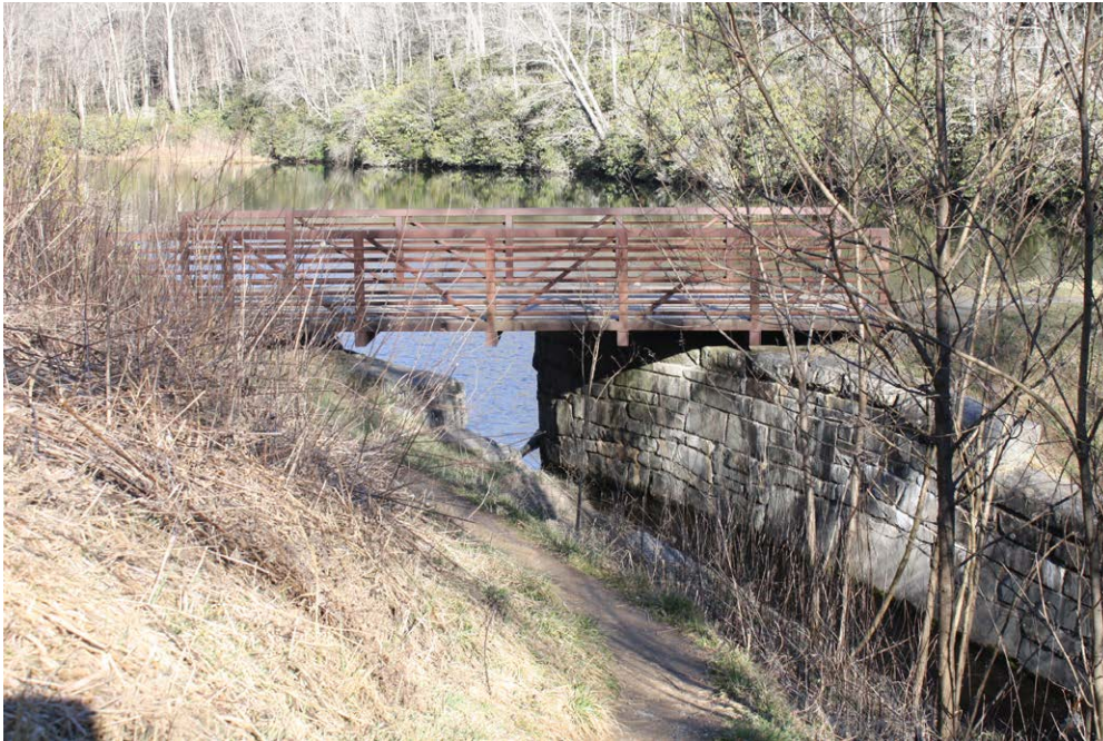
Plate 11.3: The uncoursed, dressed stone walls lining the spillway at Sims Pond Dam (WT0957).
