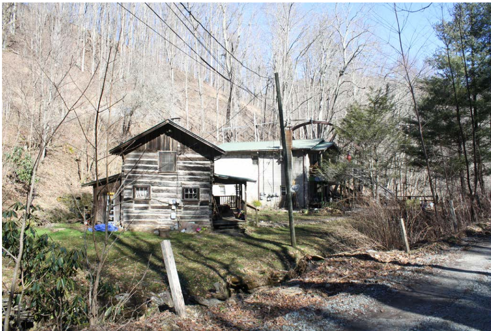
Plate 12.18: South elevation of the log house on the west side of Trivett Branch, showing the mill and machine shop in the background.
