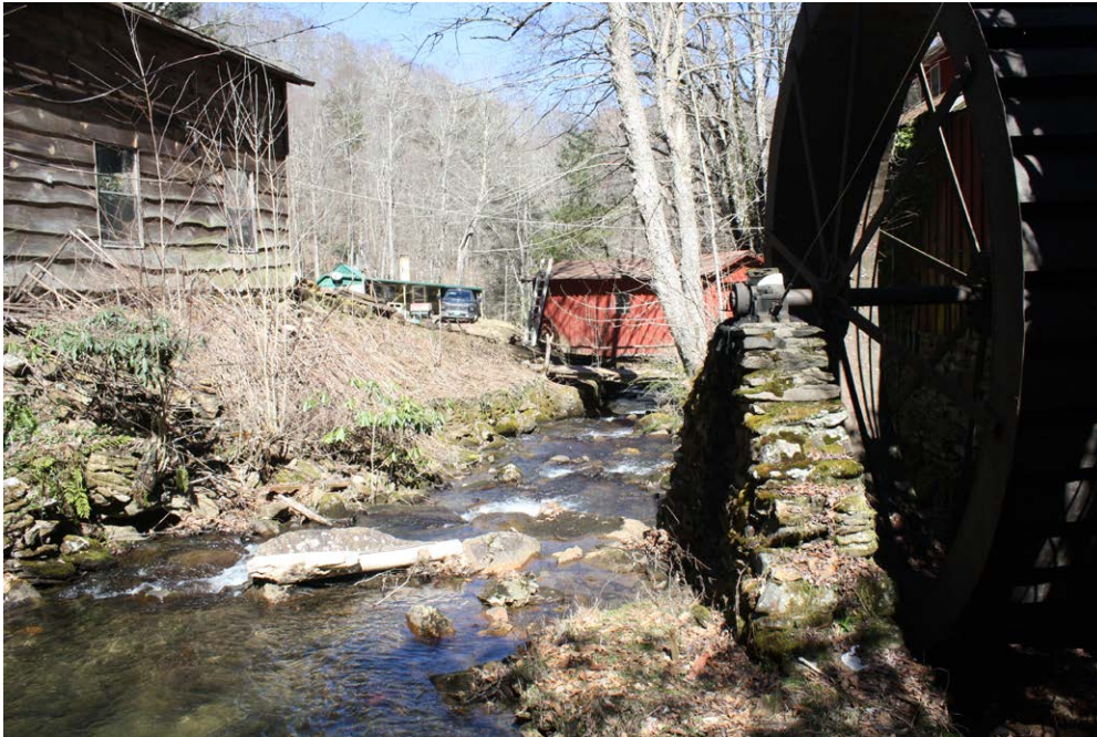
Plate 12.11: Shed over Trivett Branch, showing the barn (left) and mill (right).
