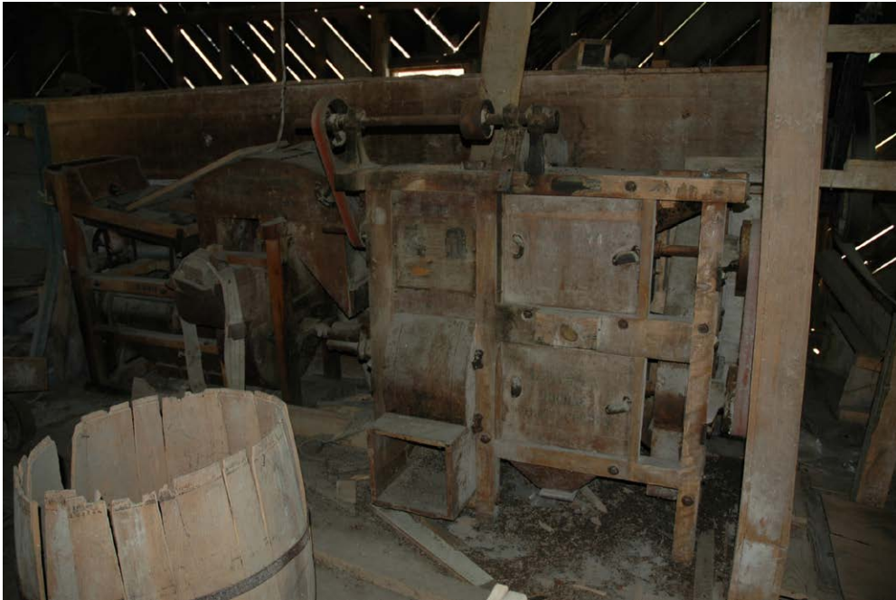
Plate 9.5: Detail of machinery inside Winebarger Mill (WT0478).
