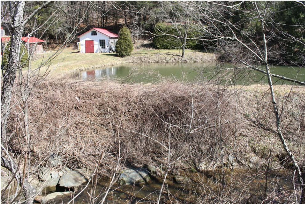
Plate 5.3: Northern embankment of Knight Pond Dam (AV0215), from Millers Gap Highway.
