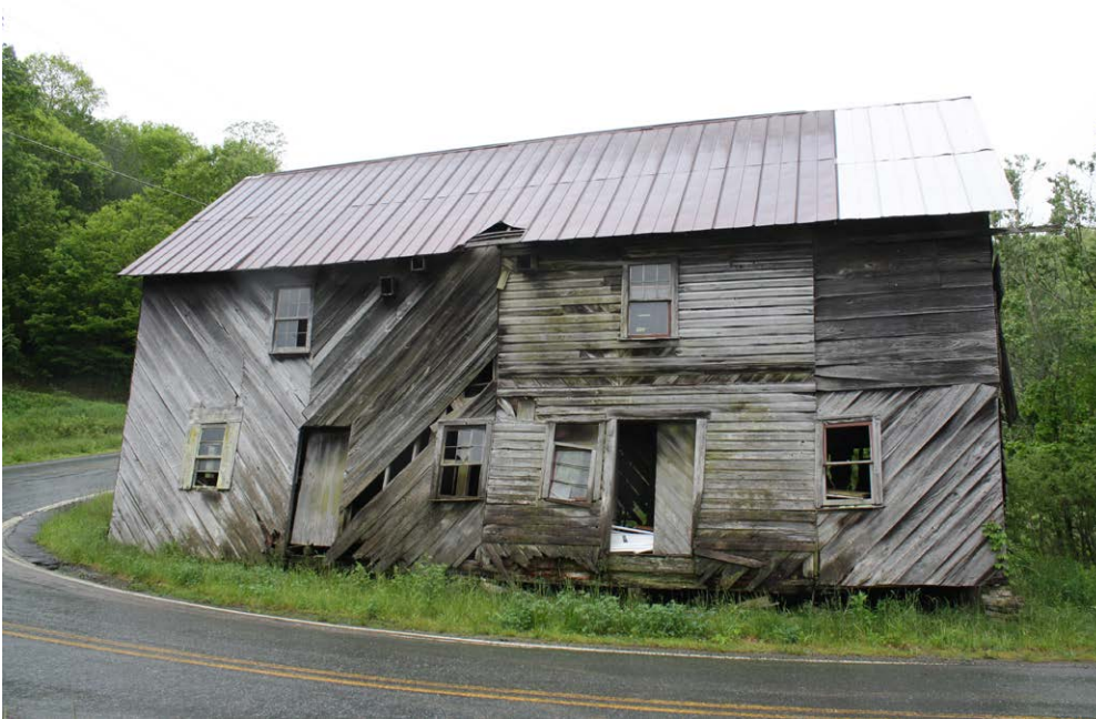
Plate 9.2: North elevation of Winebarger Mill (WT0478), from Hopewell Church Road.
