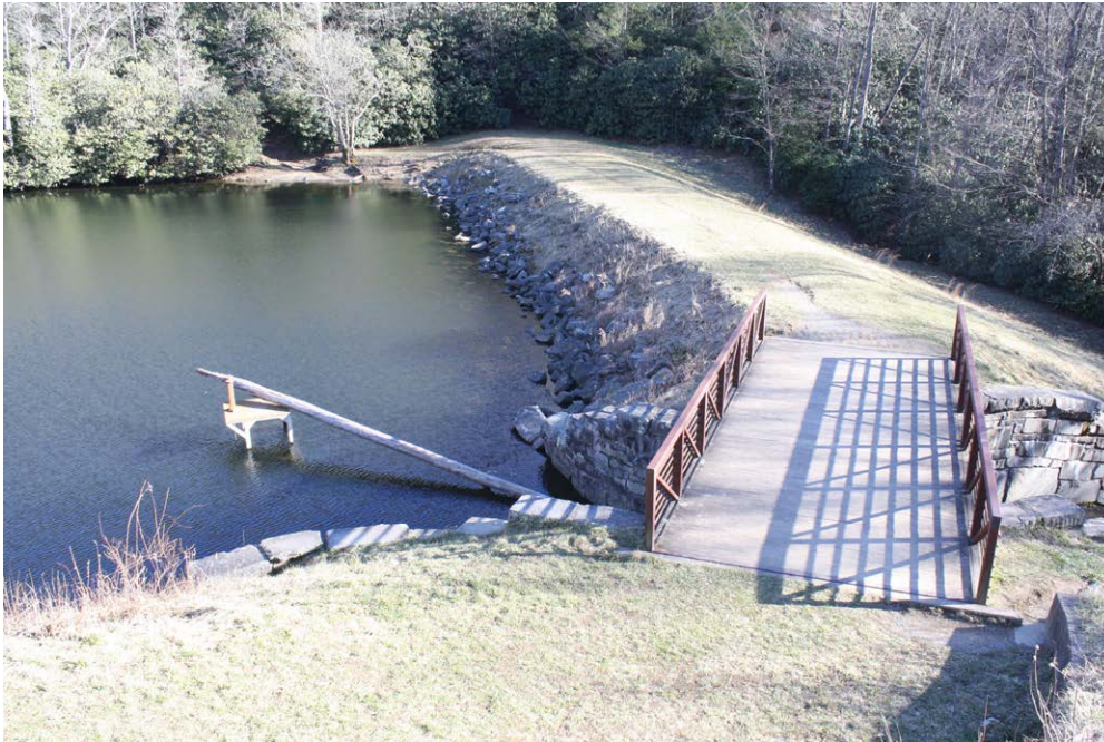
Plate 11.1: Bridge over the Sims Pond Dam spillway (foreground) and the earthen dam beyond it (WT0957), from the Sims Pond Overlook on the Blue Ridge Parkway.
