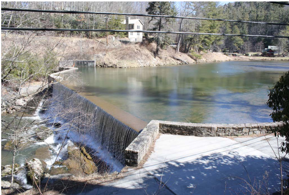
Plate 6.2: Uncoursed rubble stone wall on the south side of the Lees-McRae College Mill Pond and Dam (AV0252).
