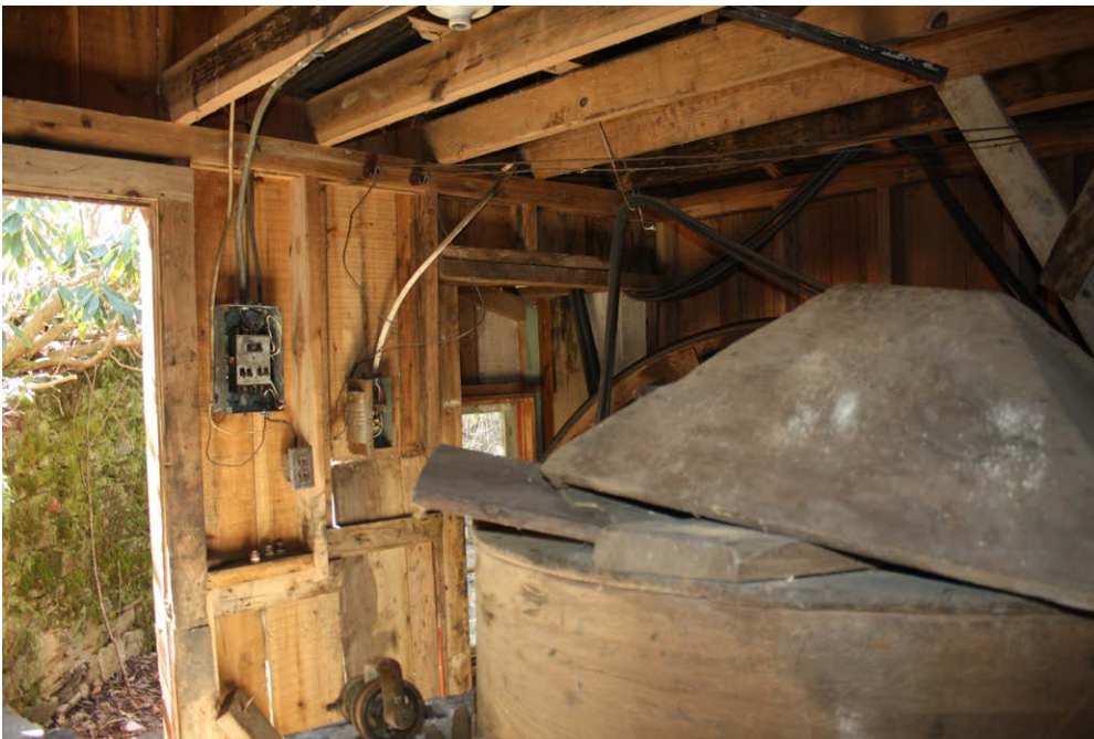
Plate 12.8: Interior of the mill.
