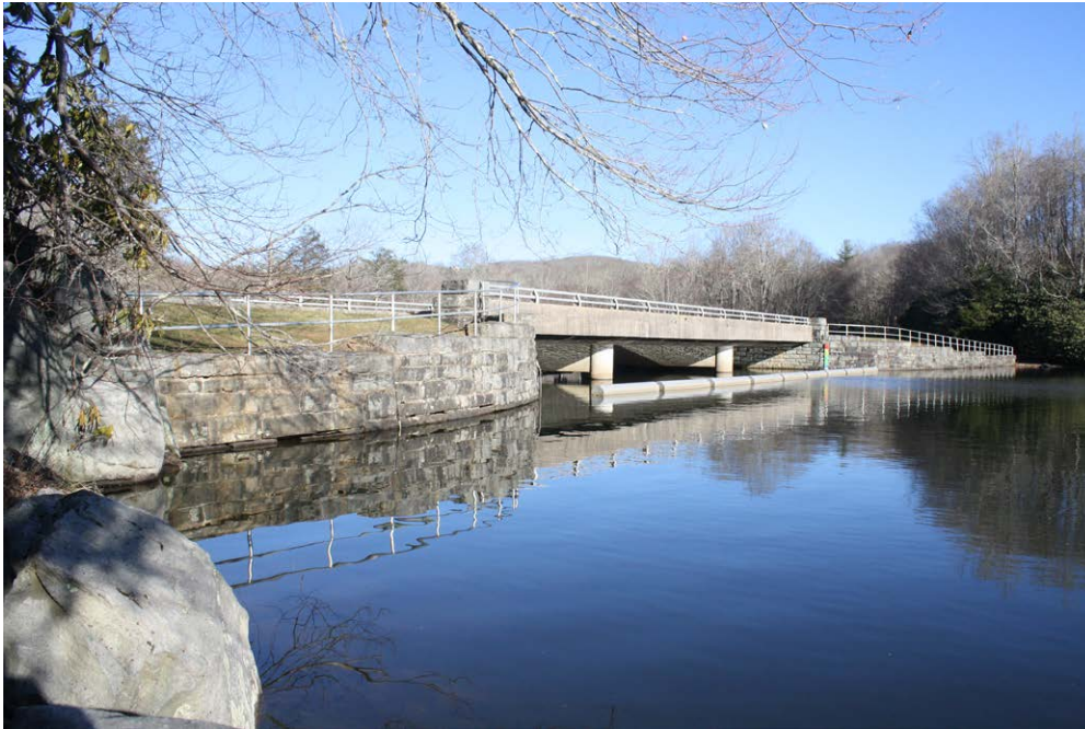
Plate 10.1: Price Lake Dam and Bridge (WT0734), on the north side of Price Lake, from the Price Lake Overlook on the Blue Ridge Parkway.
