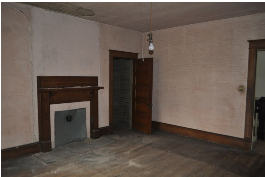
Plate 4.37: L.C. Yeargan House, east back bedroom
