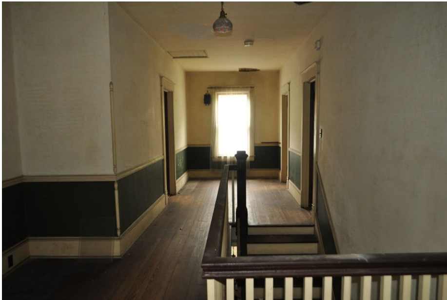
Plate 4.35: L.C. Yeargan House, upper stair hall.
