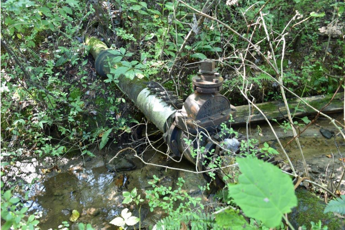
Water supply line and gate valve over branch on western edge of park, view to west
