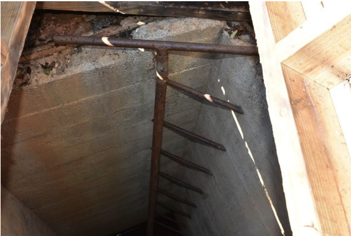
Shaft to water supply line control valve at northwest end of dam, view to south
