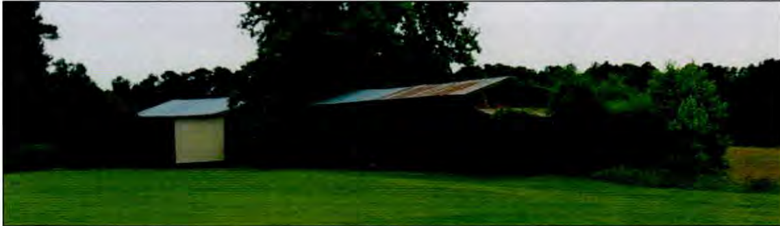
Photo 25: View of Two Machine Sheds, Looking South, Beaver House.
