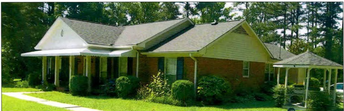
Photo 20: Southeast Oblique of Circa-1975 Ranch House.
