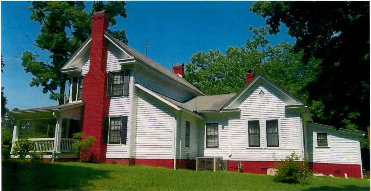
Photo 18: West Elevation of G. H. Baucom House.
