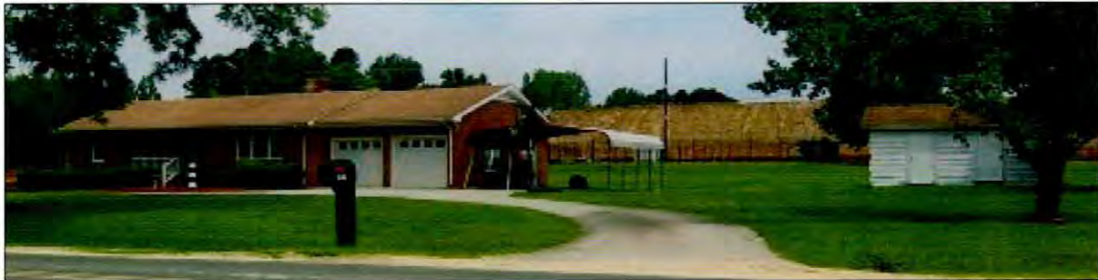
Photo 23: View of 3616 Green Level West Road, Looking North-Northwest.
