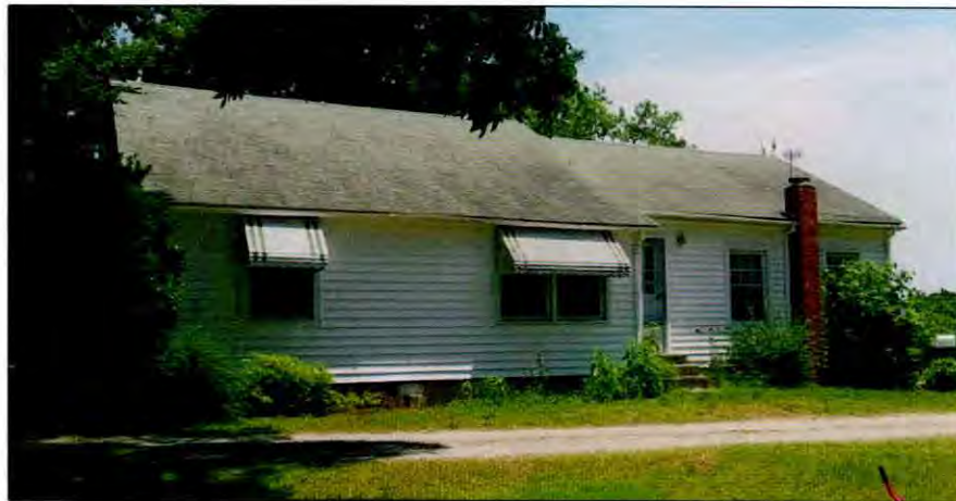
Photo 24: View of West Elevation, Karmen Strother House.
