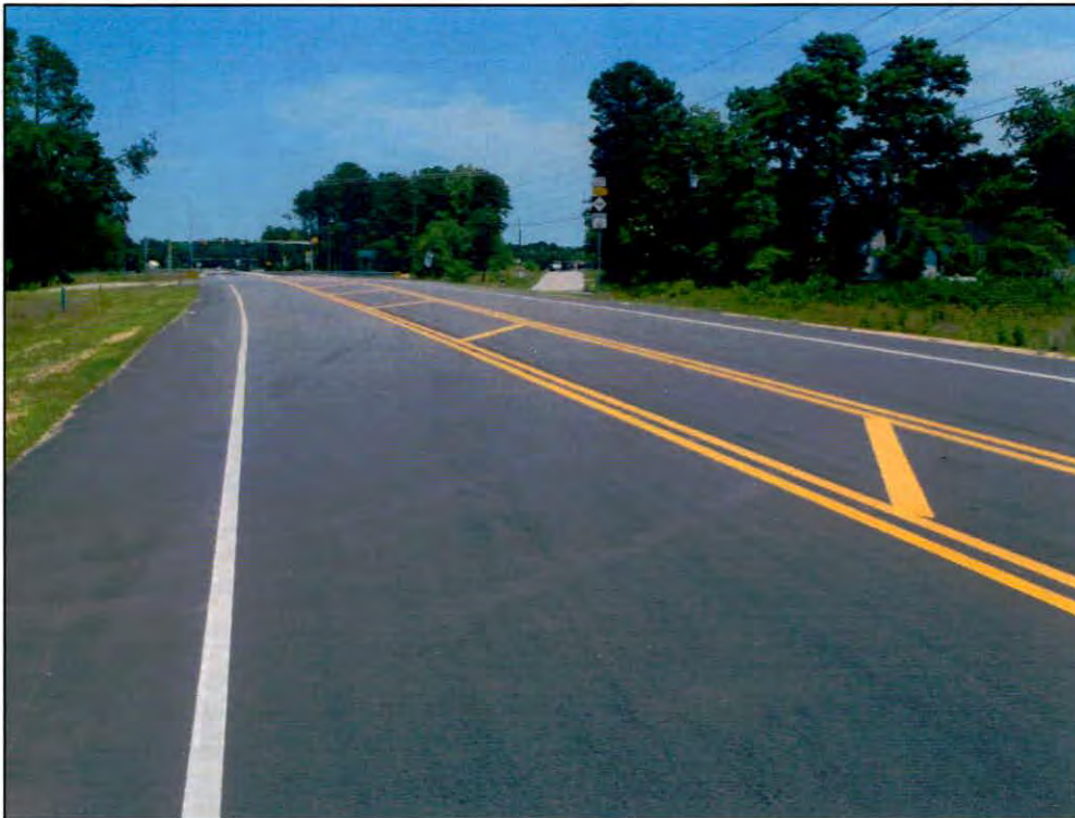
Photo 4: New Road Construction at the Intersection of Green Level West Road and I-540, Facing East.
