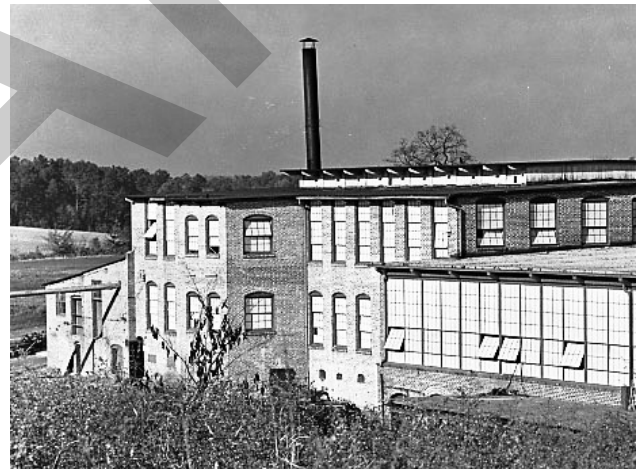
Figure 2. This view of the two-story Black Ox Mill shows the west elevation to the left and the south elevation to the right, rising above the ca. 1929 one-story addition to the far right. The small shed-roofed wing at the far left was removed in 1947.
