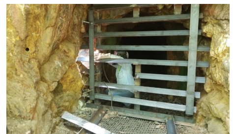
Cave Gate Installation at Crowders Mountain State Park
