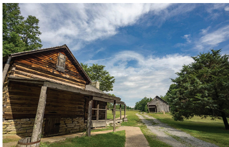
Hutchinson Homestead at Stone Mountain State Park
