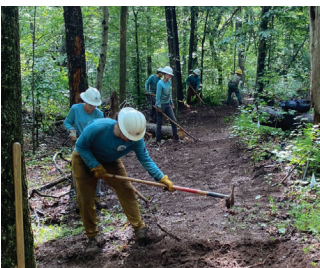
CCNC crews construct the Fox Trail at Mayo River State Park
